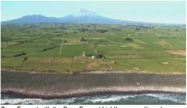
Cape Egmont with the Cape Egmont Lighthouse positioned upon a laharic dome
