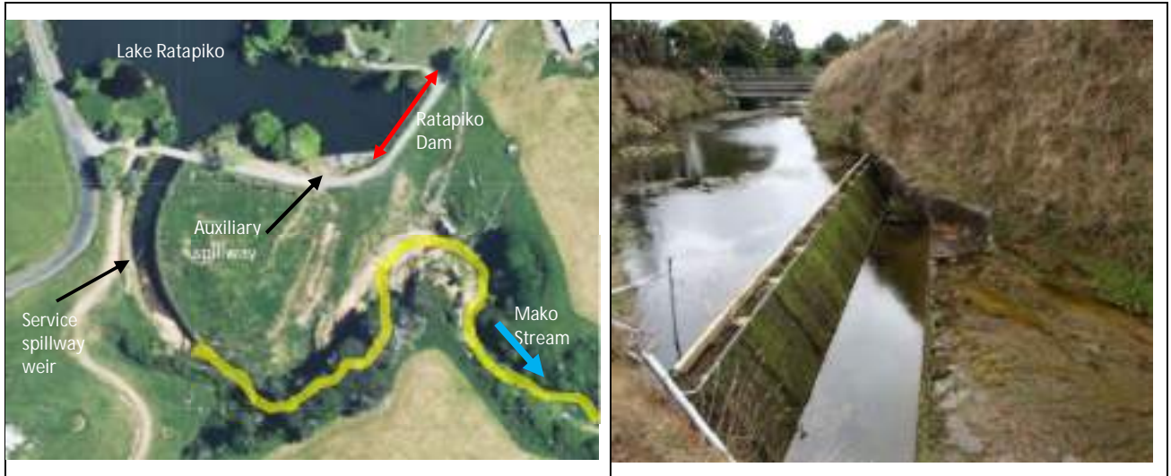
Figure 3.12 The left frame shows a vertical aerial view of the dam and its spillways (labelled). The right frame shows the service spillway and its flashboards
