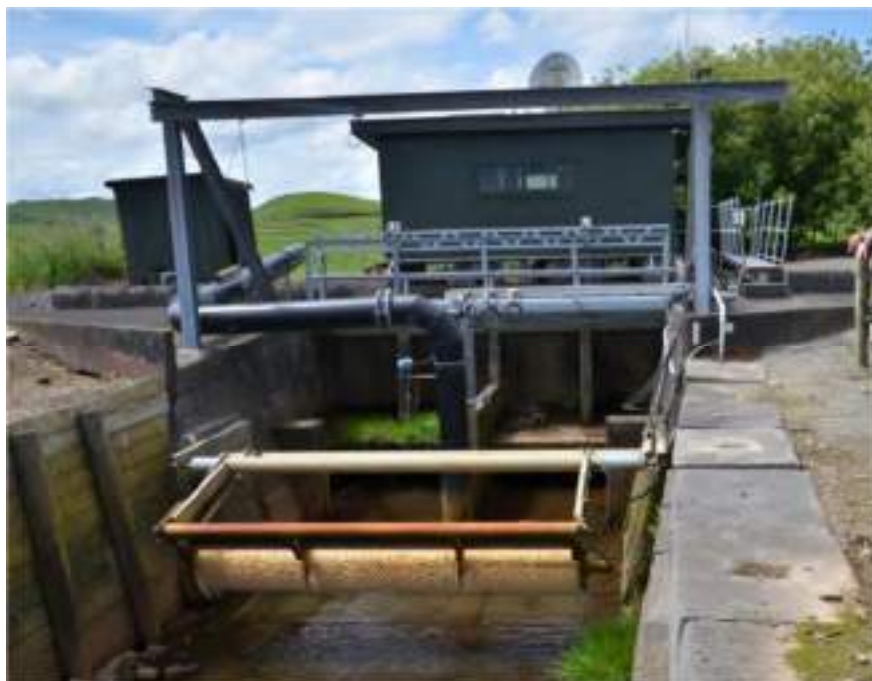
Figure 3.10 The pump station for abstracting water from Mangaotea Stream to the Motukawa Race
