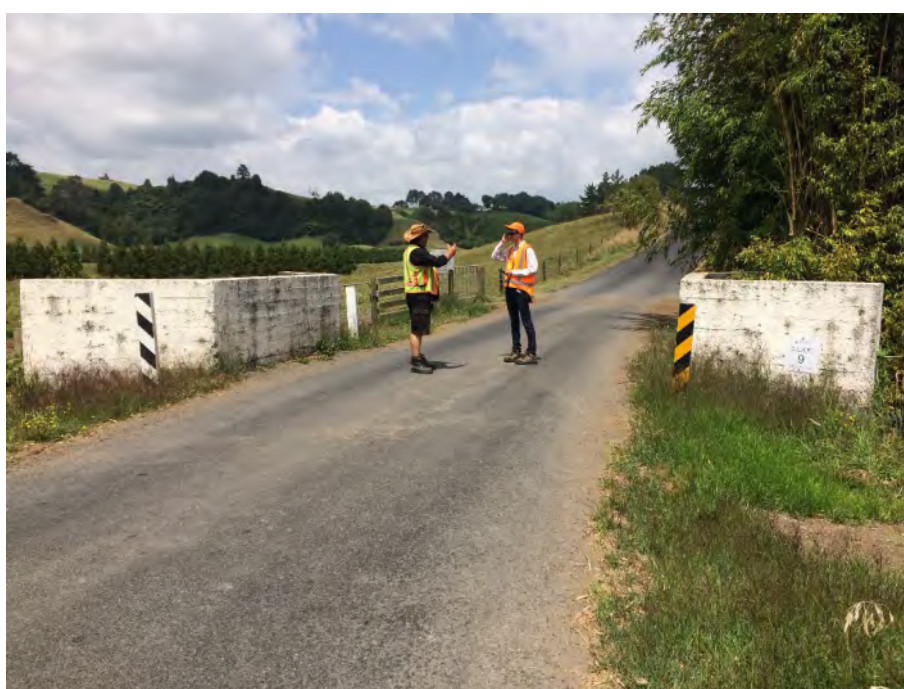
Photo 2: Salisbury Road Culvert. View towards the south along Salisbury Road
