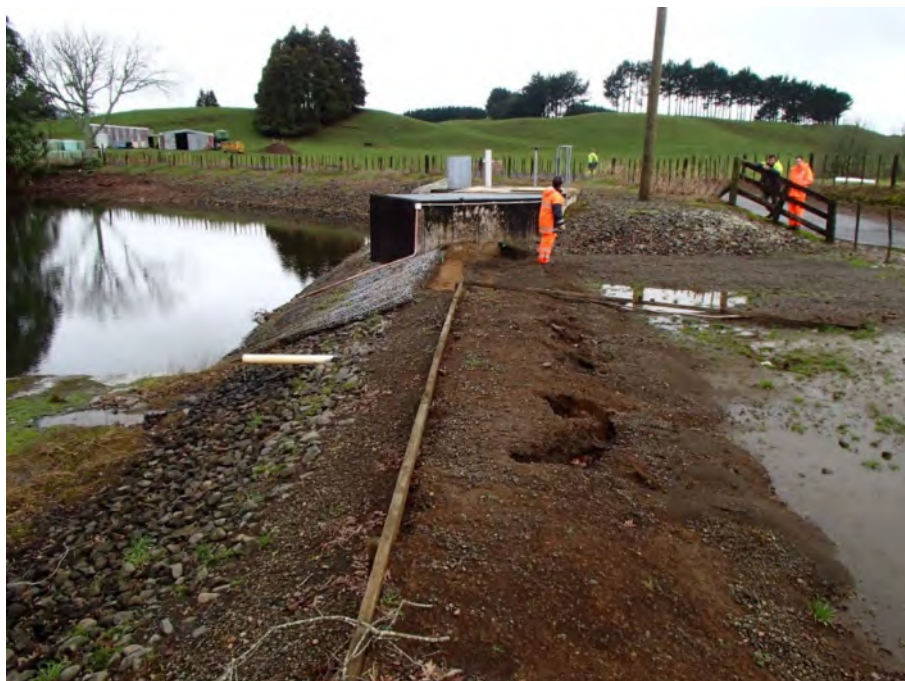
Photo 2: Photograph taken on 7 July 2015 (after June 2015 flood event) Note: Only the true left-hand-side of the fuse plug has fused, although scour is evident on the downstream face of the unfused plug. Lake level instrument MTK_H13LT_007 is located on the face of the gabion mattress.
