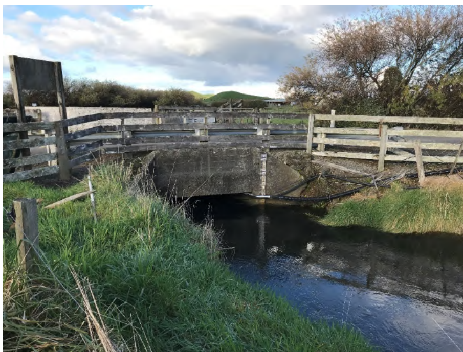
Photo 8: Mangaotea Road Culvert entrance (June 2020).
