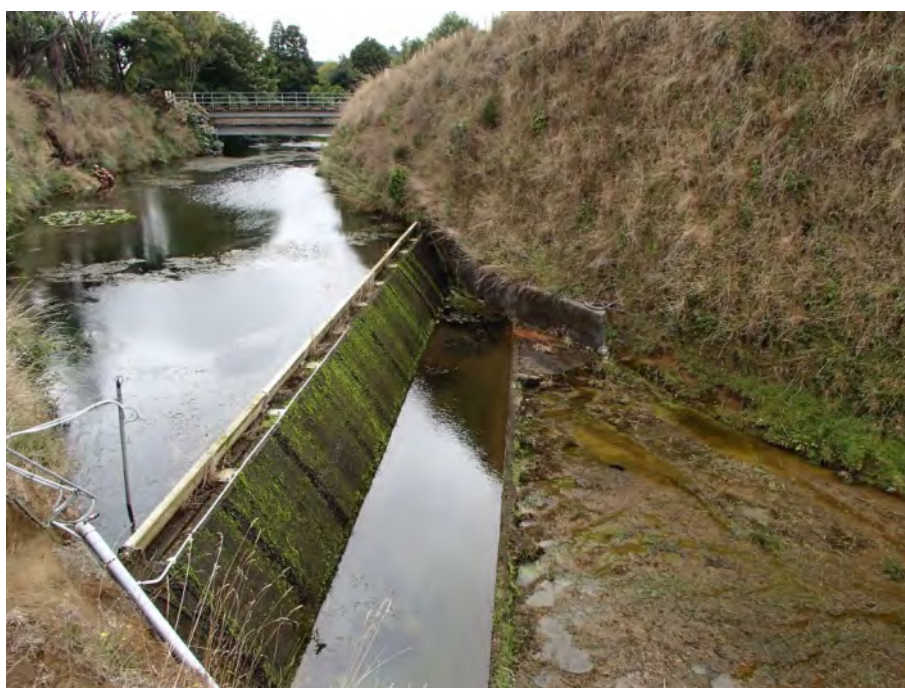
Photo 5: Service Spillway Flashboards (Photograph taken in 2016)
