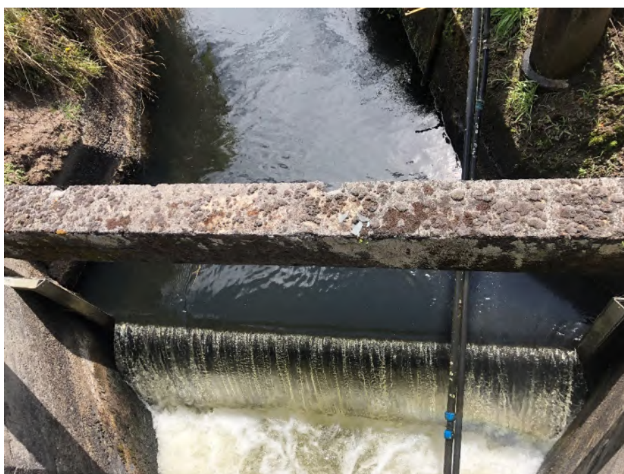
Photo 3: Flow over Tariki Weir (February 2019).
