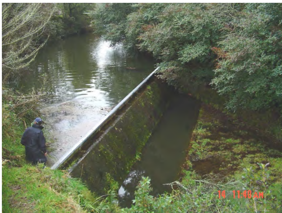
Photo 4: Service Spillway Flashboards (Photograph taken in 2004)
