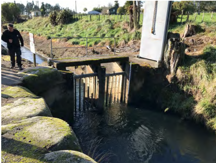
Photograph 1: Intake screens, with concrete lined Race downstream (June 2020).
