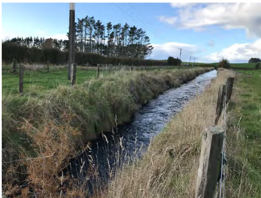
Photograph 4: View from CH 1075 (end of concrete lining) downstream (June 2020). Note the velocities reducing downstream.
