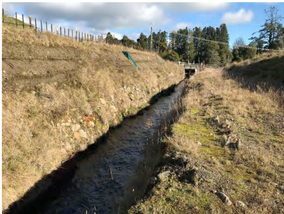
Photograph 2: View from CH150 upstream with the intake gates visible (June 2020).
