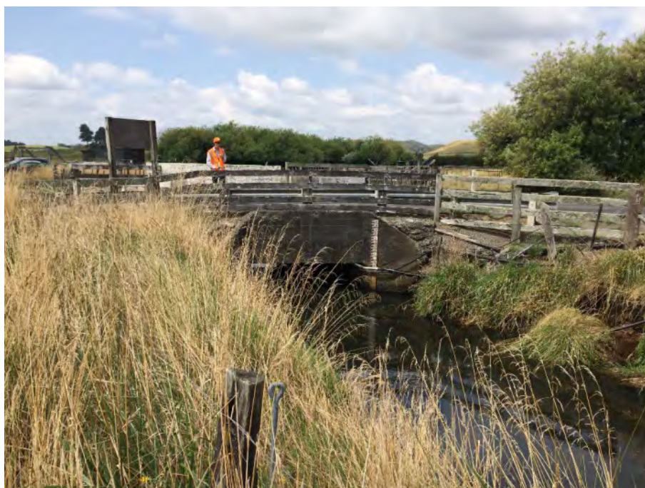
Photo 3: View downstream towards Mangaotea Road Culvert
