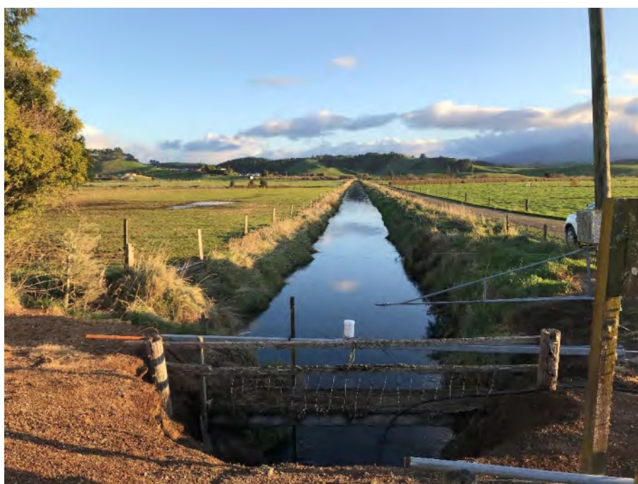
Photograph 16: View upstream from Tunnel 2 (June 2020). Note the low velocities and the well vegetated banks.
