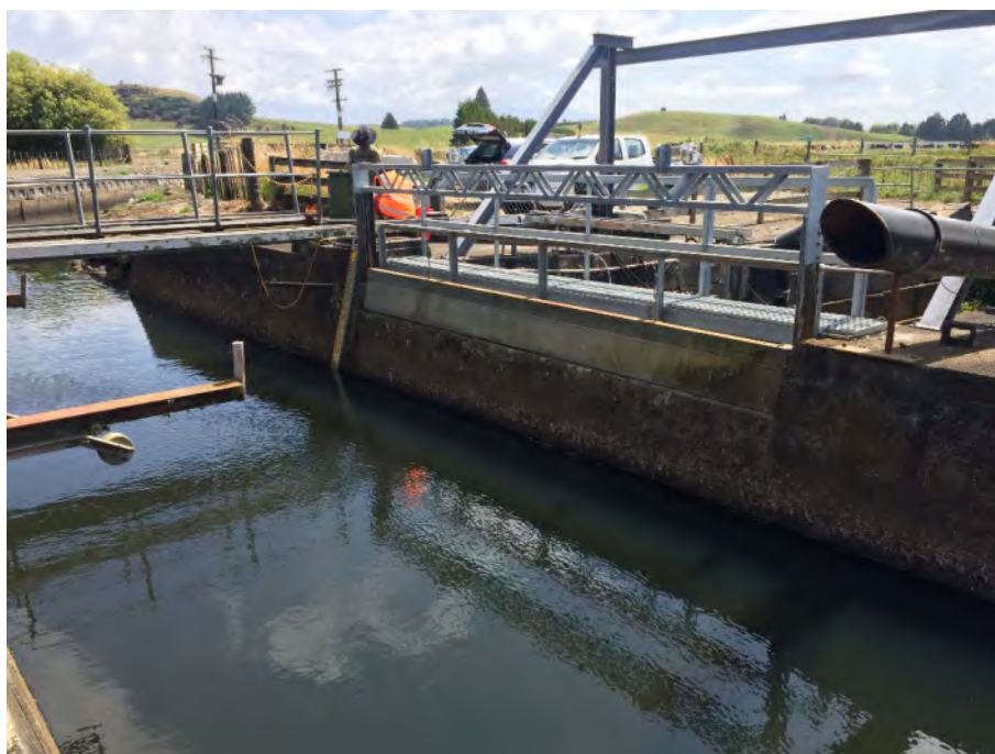
Photo 1: Mangaotea Aqueduct and Spillway Gate (February 2019)
