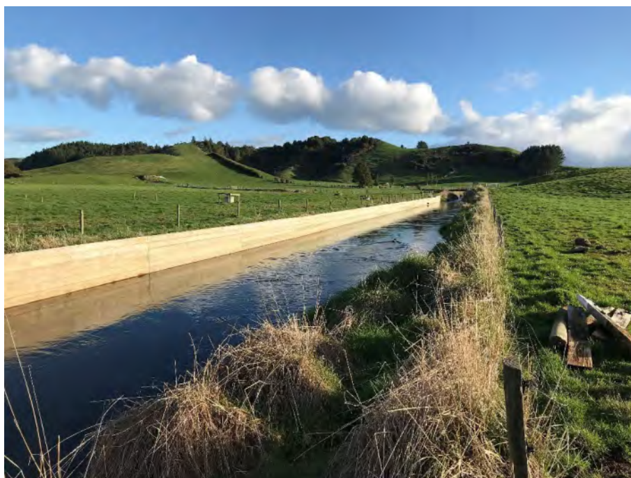
Photograph 13: Recent timber retaining wall remedial works (June 2020). Note the relatively low velocities within the Race and the low lying nature of the surrounding floodplain. Upper Mangaotea Bridge is beyond the upstream extent of the wall.
