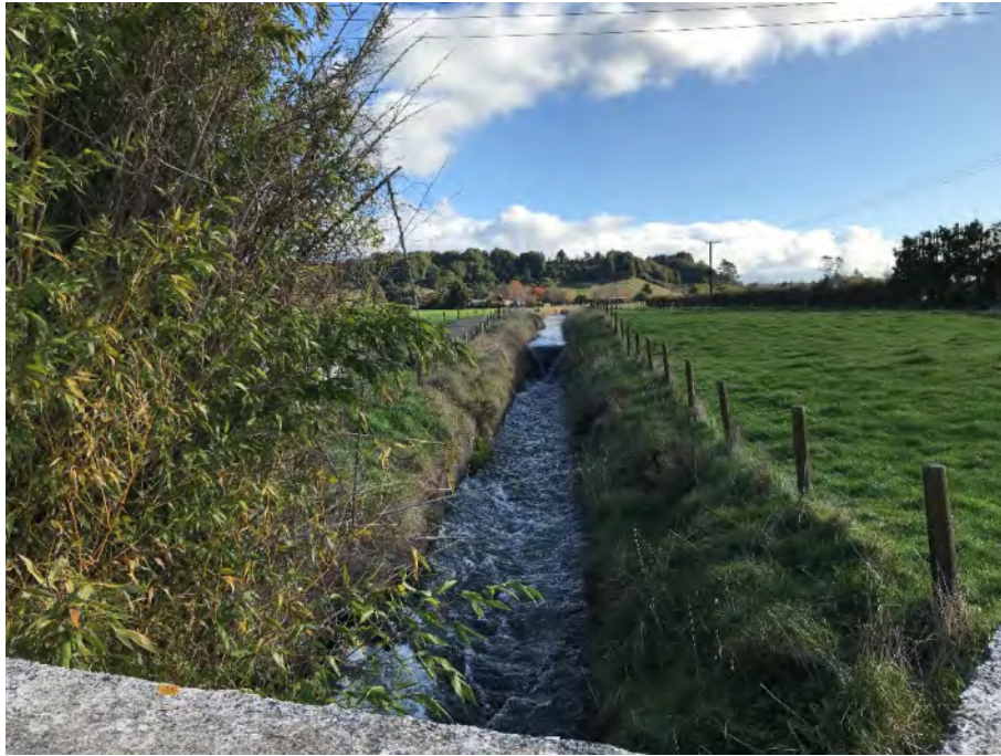
Photograph 6: View from Salisbury Road Culvert CH 1325 upstream (June 2020). Note the drop structure and the higher velocities downstream of this (concrete lined).
