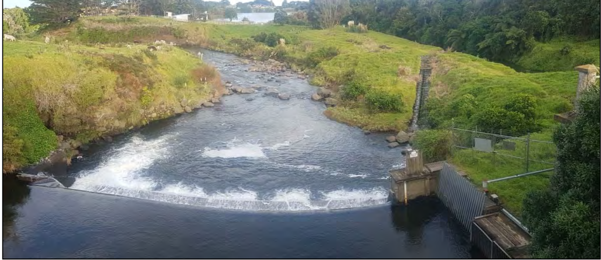
Photo 1 The Waiaua River, weir, intake, canal, fish pass and Lake Opunake, as viewed from the State Highway 45 Bridge, Opunake.
