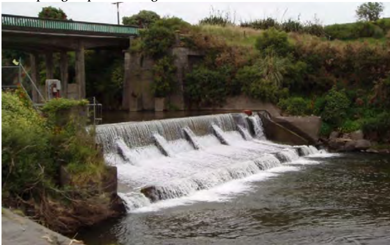
Photo 1 The weir on the Waiaua River associated with the Opunake Hydro intake.
