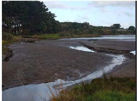
Photo: 2016 June Low level <500mm after canal wall installation
