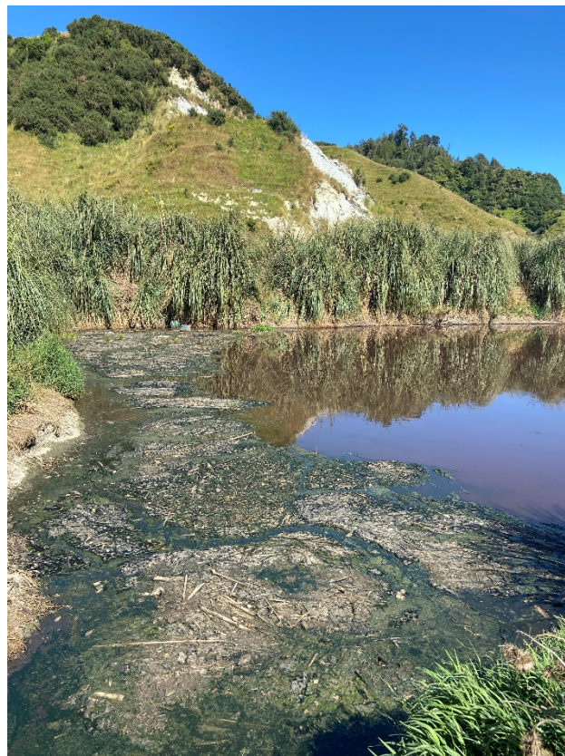
Photograph 2: Stormwater Treatment Pond with accumulated sediment
