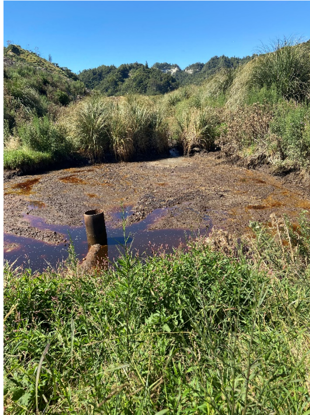
Photograph 5: Stormwater Treatment Pond with accumulated hydrocarbon product
