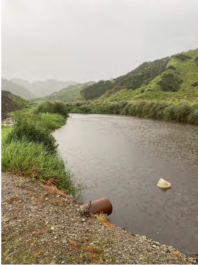
Photo 6. Irrigation pond with perched pipe inflow from drilling waste leachate collection area.
