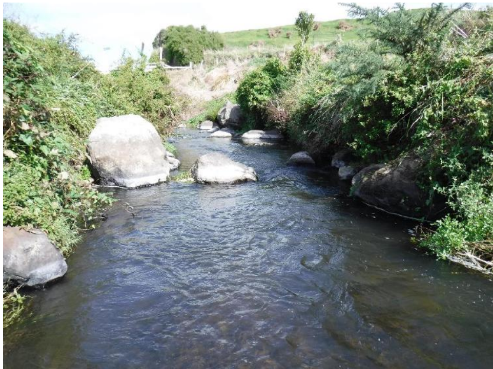
Plate 4: Inaha Stream Normanby Rd Bridge, 1450m d/s of point source discharges from the ORP.
