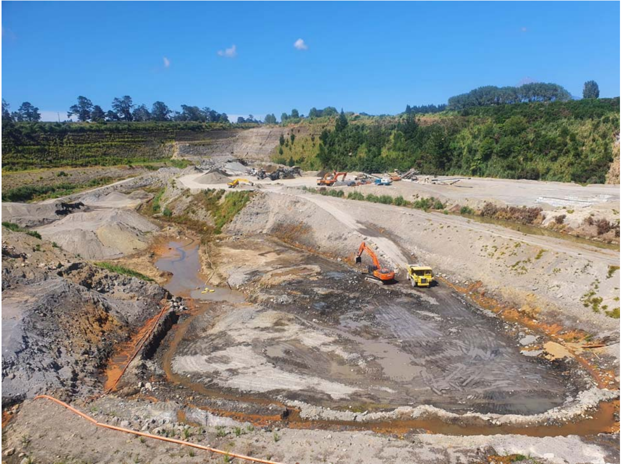
Photo 1 New excavation area west of the washwater ponds, January 2021.
