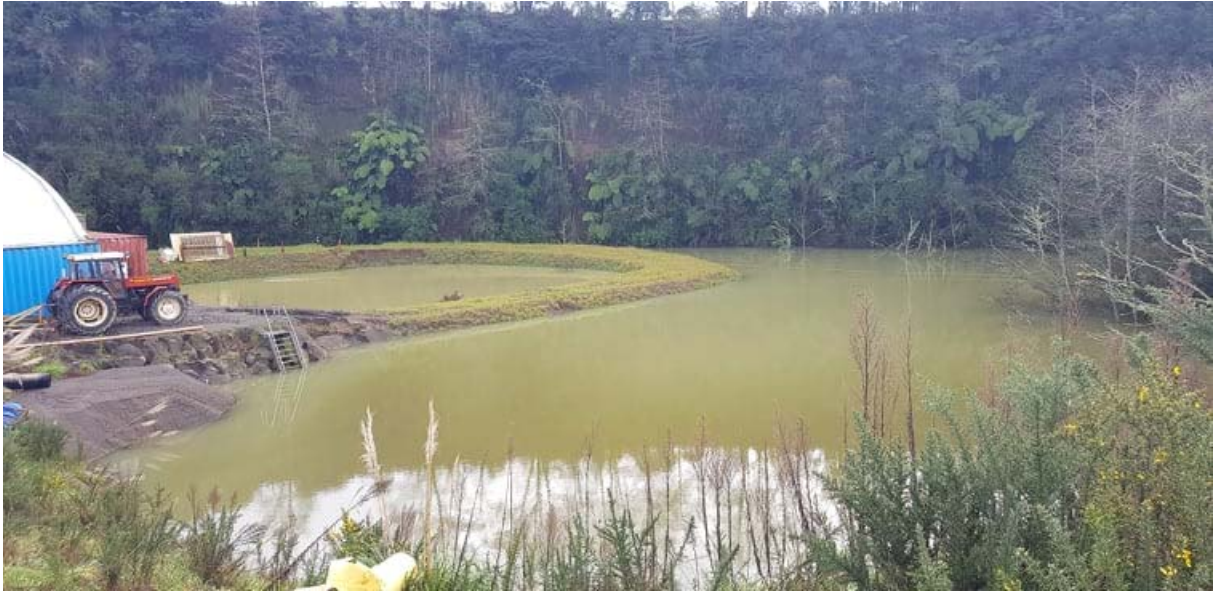
Photo 3 Stormwater Ponds B and C, July 2021.
