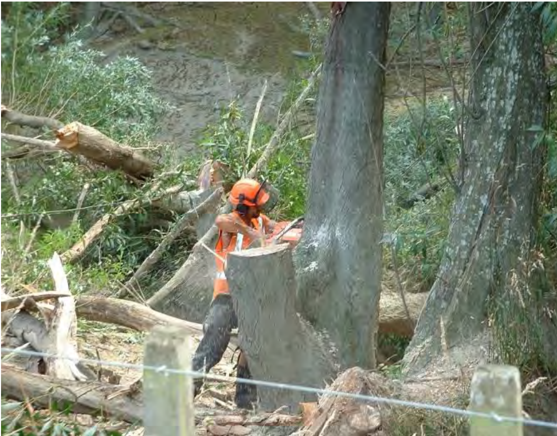
Figure 2: Willow removal showing how large some of the trees were
