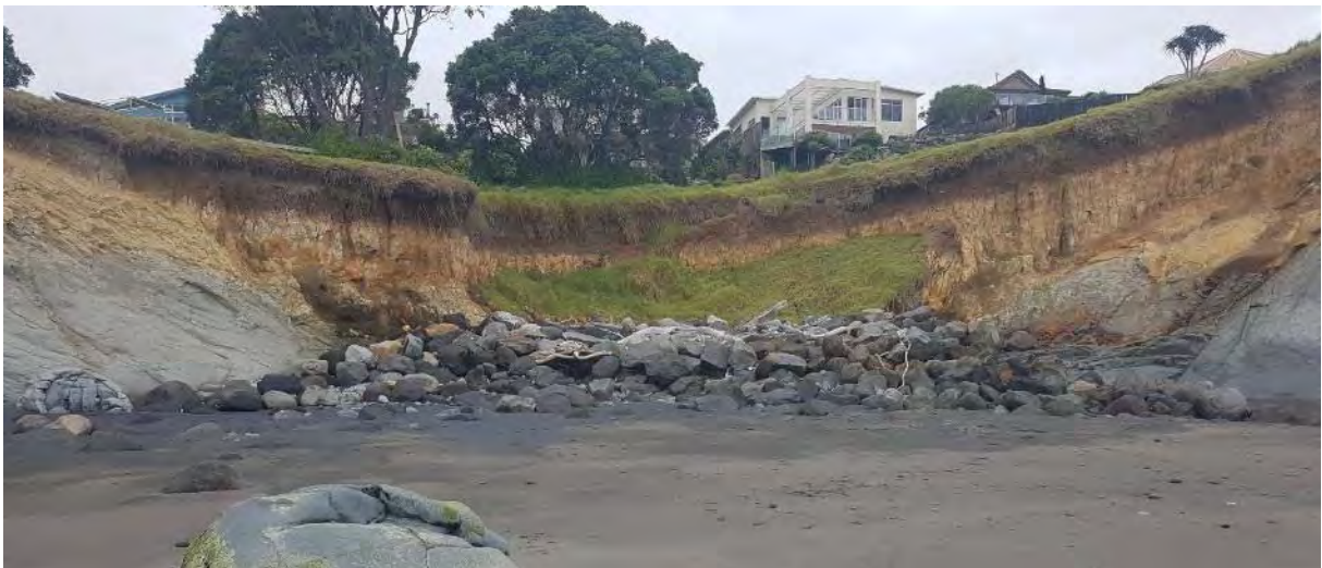
Photo 4 Onaero beach incision repair and eroding cliffs, May 2020
