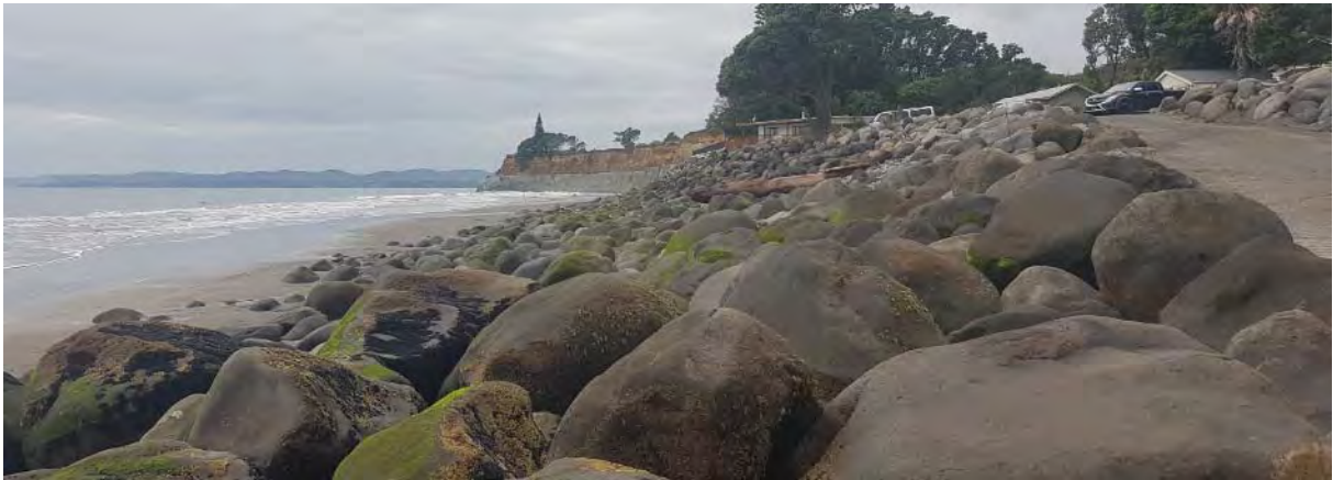
Photo 3 Onaero Beach seawall gradient, May 2020
