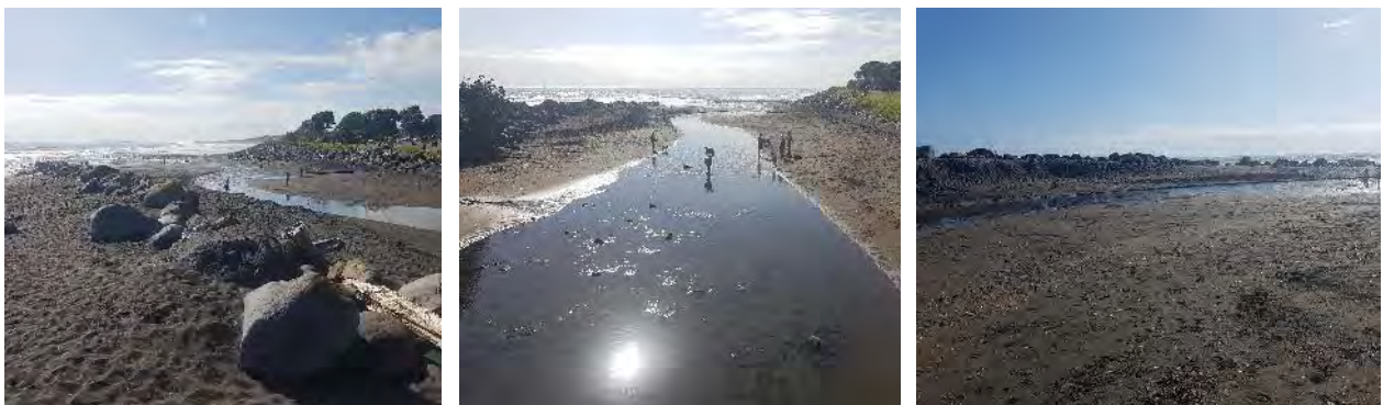
Photo 12 Sand build up at Te Henui groyne, April 2020
