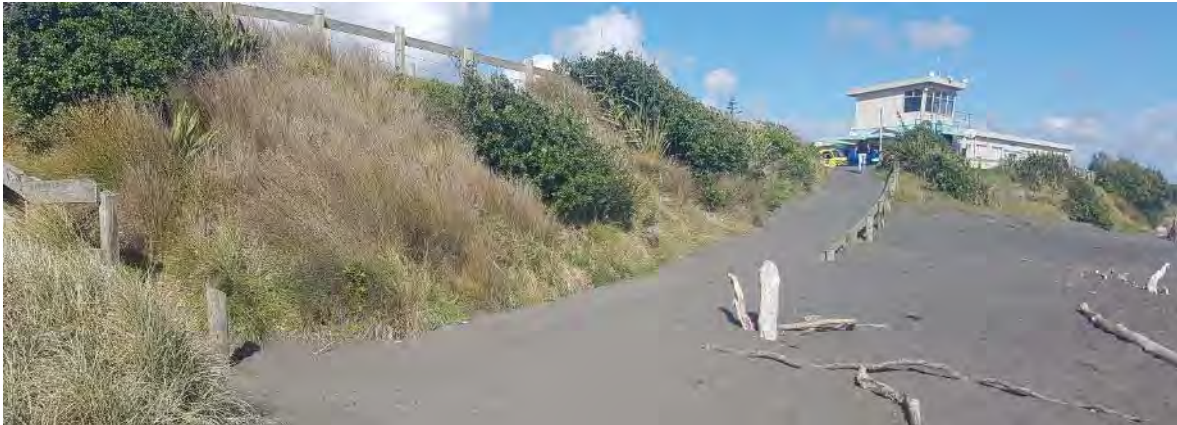
Photo 11 Sand build up on Fitzroy boat ramp, April 2020
