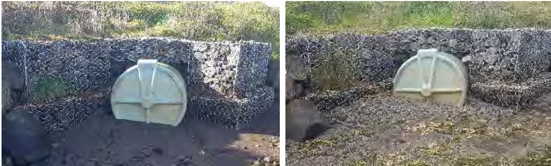
Photo 5 Atkinson/East Quay stormwater outlet (left: May 2019, right: May 2020)
