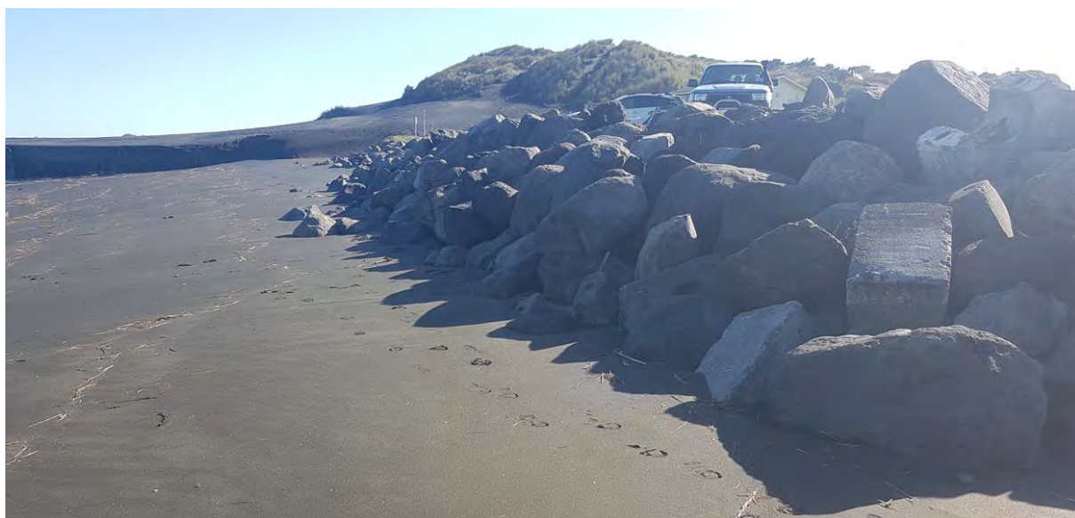
Photo 13 Mana Bay seawall, 6 May 2020
