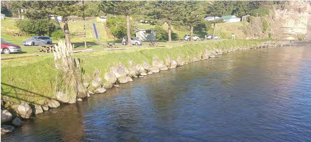
Photo 11 Kaupokonui Stream boulder rip rap protection works (6 May 2020)
