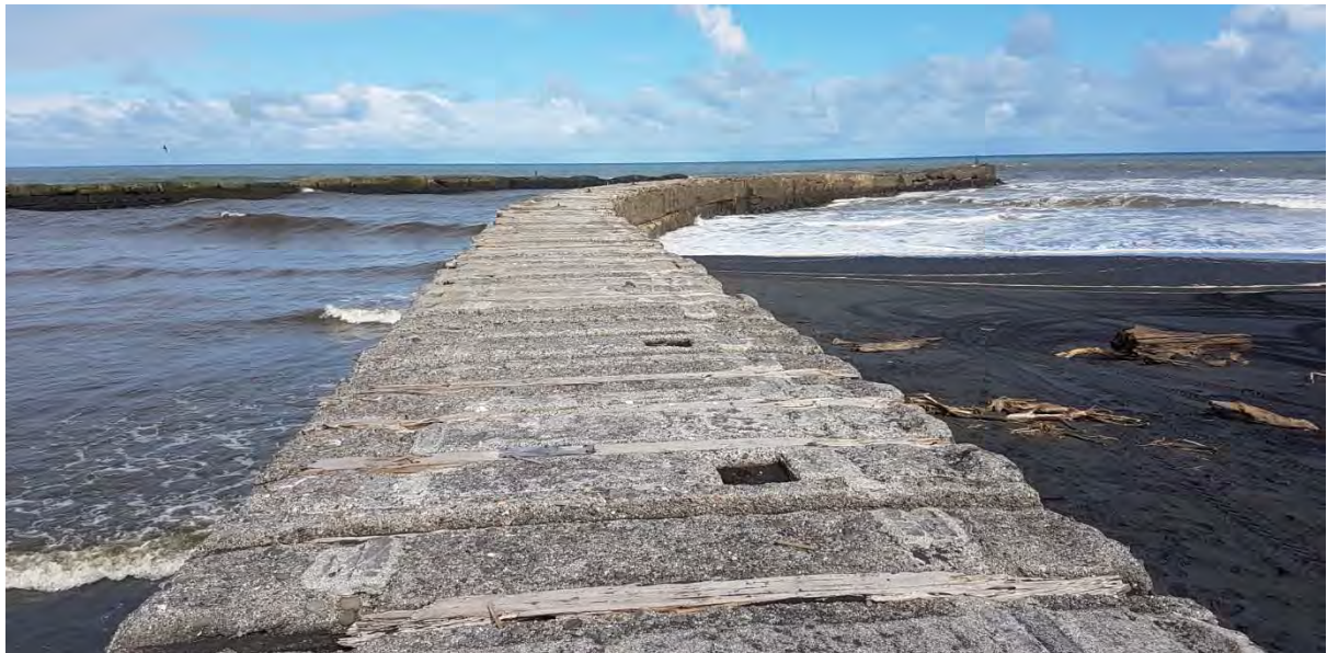
Photo 5 Patea groynes (April 2017)
