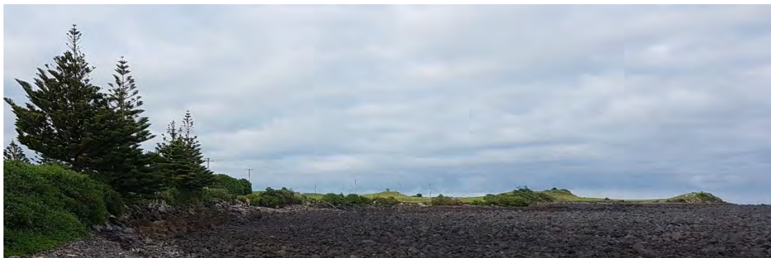
Photo 1 Bayly Road seawall (April 2017)
