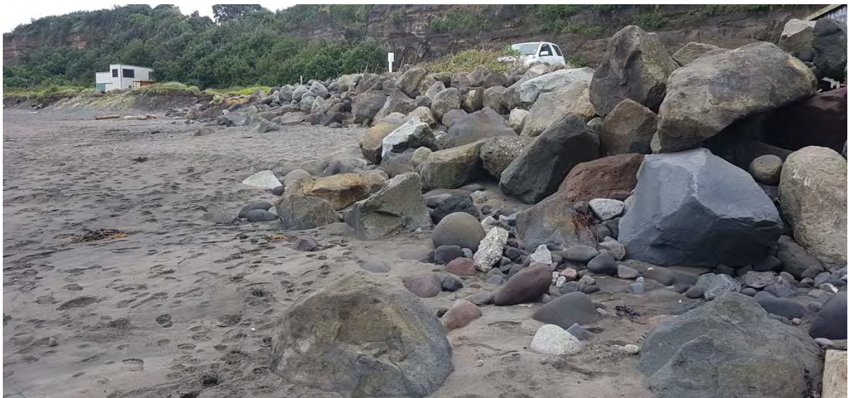
Photo 2 Rip-rap seawall, Middleton Bay (April 2017)
