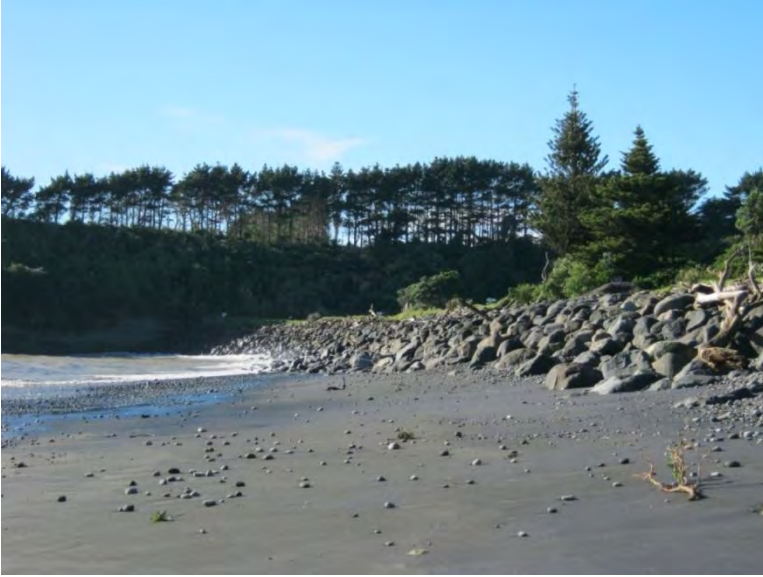
Photo 17 Urenui rip rap protection seawall (June 2013)
