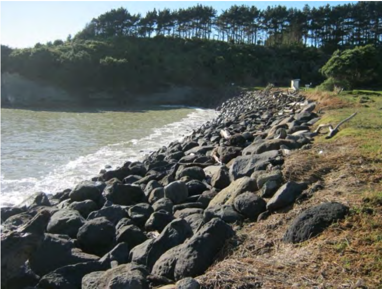
Photo 18 Urenui Rip rap protection seawall (May 2014)
