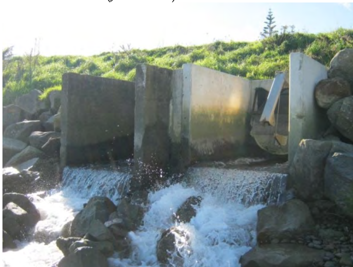
Photo 24 Stormwater outlet structure downstream of Atkinson Street (June 2013)
