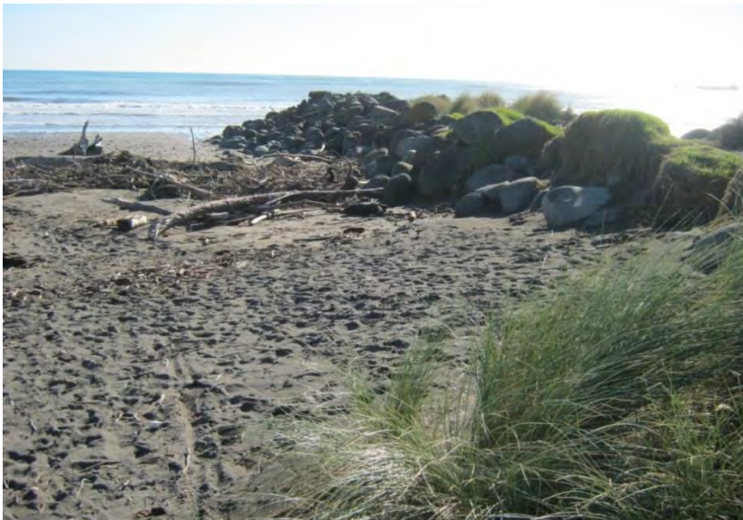
Photo 29 Waiwhakaiho groyne (May 2014)
