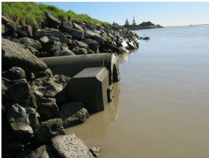
Photo 12 Stormwater outlet structure McNaughton Street, Waitara (June 2013 and May 2014)
