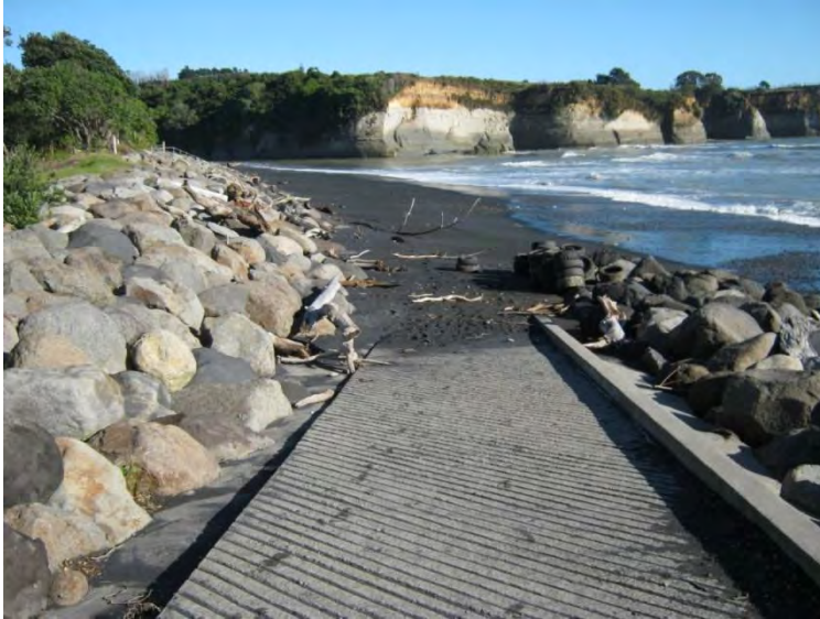
Photo 4 Urenui beach access and rip rap wall (May 2014)
