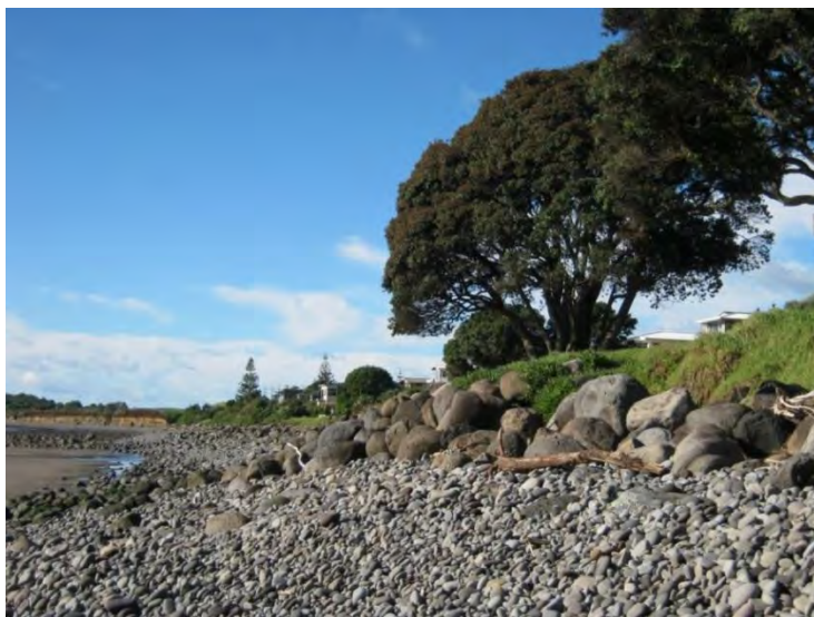
Photo 28 Bell Block seawall (June 2013)
