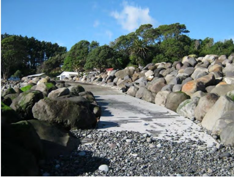
Photo 23 Onaero boat ramp and seawall (June 2013)
