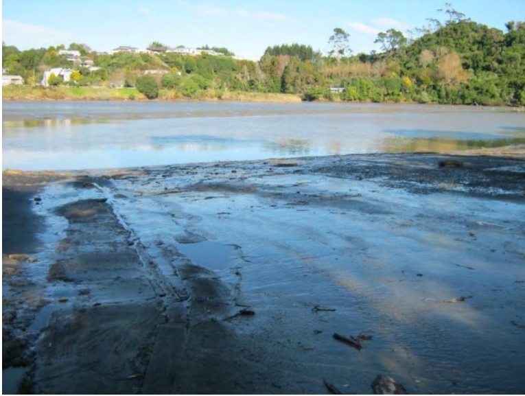
Photo 15 The Urenui boat ramp (June 2013)
