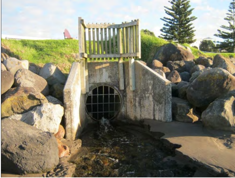
Photo 36 The Bayly road stormwater outfall on Ngamotu Beach (May 2014)
