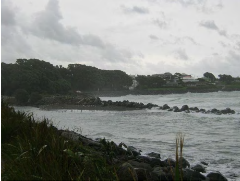
Photo 10 The Te Henui groyne (April 2012)
