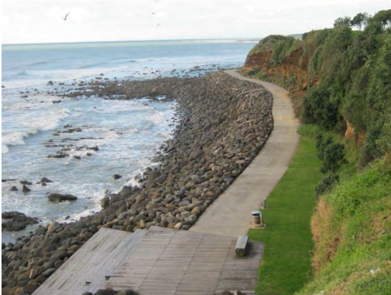
Photo 11 New Plymouth coastal walkway with rip rap seawall protection (June 2014)
