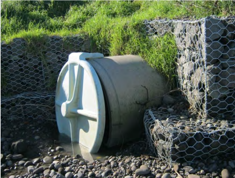
Photo 25 The stormwater outlet by the Atkinson Street/East Quay intersection (June 2013)
