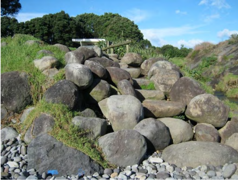
Photo 7 Rock step access to Bell Block Beach (2014)
