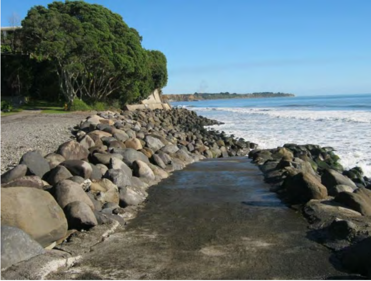
Photo 5 Onaero Beach seawall (May 2014)
