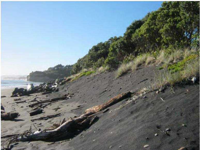
Photo 20 Urenui Rip rap protection wall extension (May 2014)
