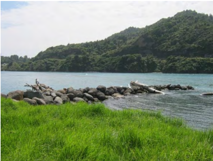
Photo 1 Rock groyne at Tongaporutu (May 2014)
