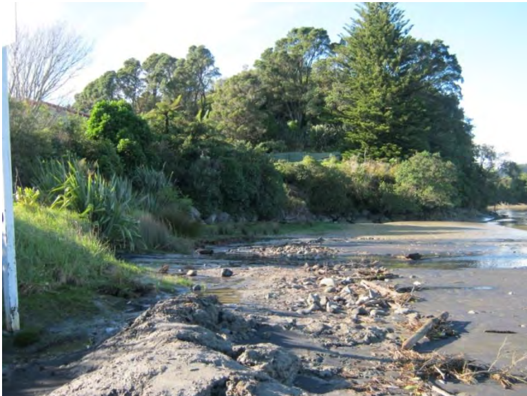
Photo 16 The riverbank protection works around the Manager's residence (June 2013)
