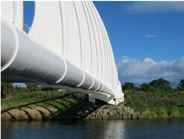
Photo 31 Te Rewarewa bridge over the Waiwhakaiho River (June 2013)
