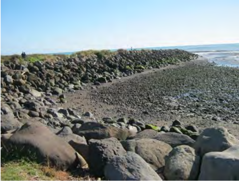
Photo 8 Waiwhakaiho groyne (May 2014)
