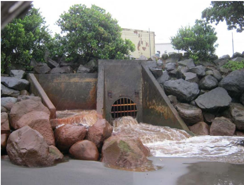
Photo 13 Hongihongi Stream outlet structure (April 2012)
