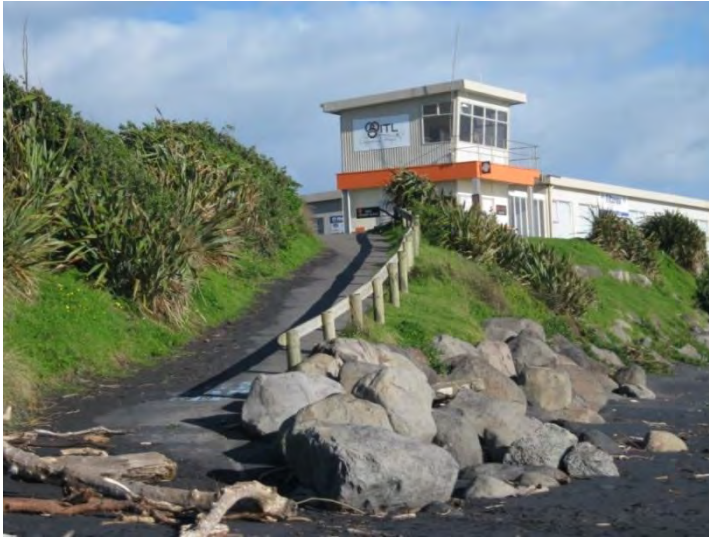
Photo 32 Boat ramp and rock protection works in front of Fitzroy Surf Lifesaving Club (June 2013)
