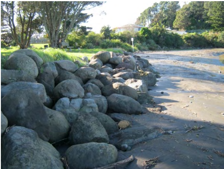
Photo 14 The riverbank protection works by the boat ramp (June 2013)
