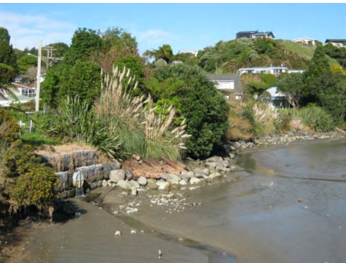
Photo 22 Urenui rip rap in the June 2013, May 2014)
