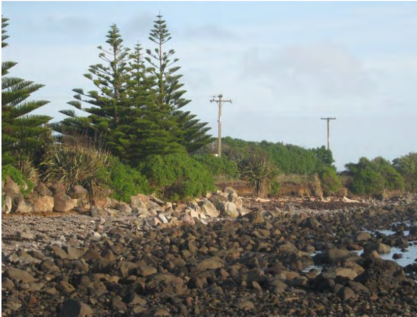
Photo 1 Bayly Road seawall (May, 2014)
