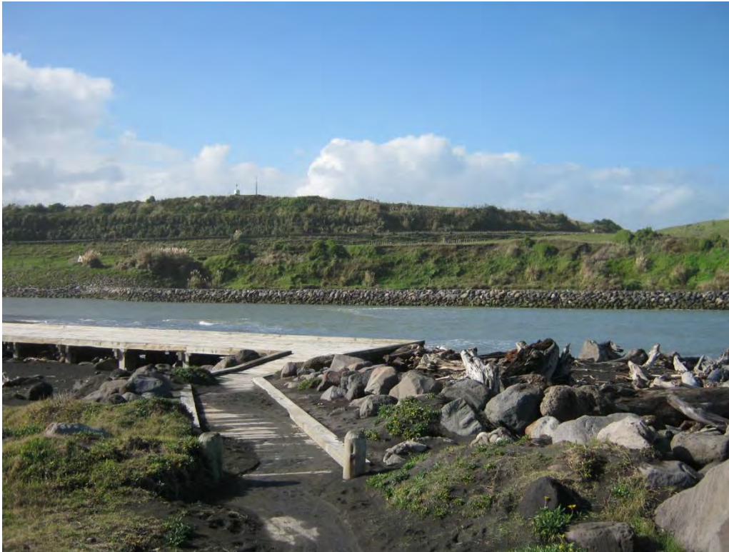
Photo 13 Training wall at Patea (May, 2014)
