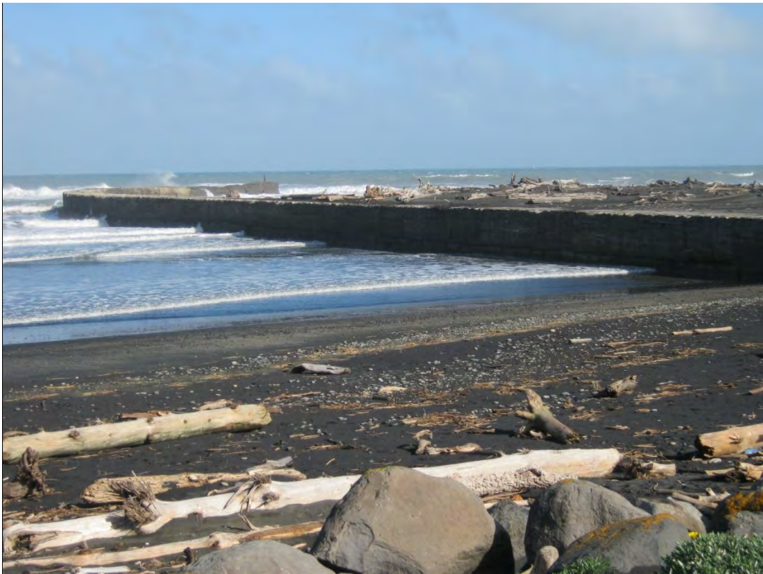
Photo 5 Patea groynes (May 2014)
