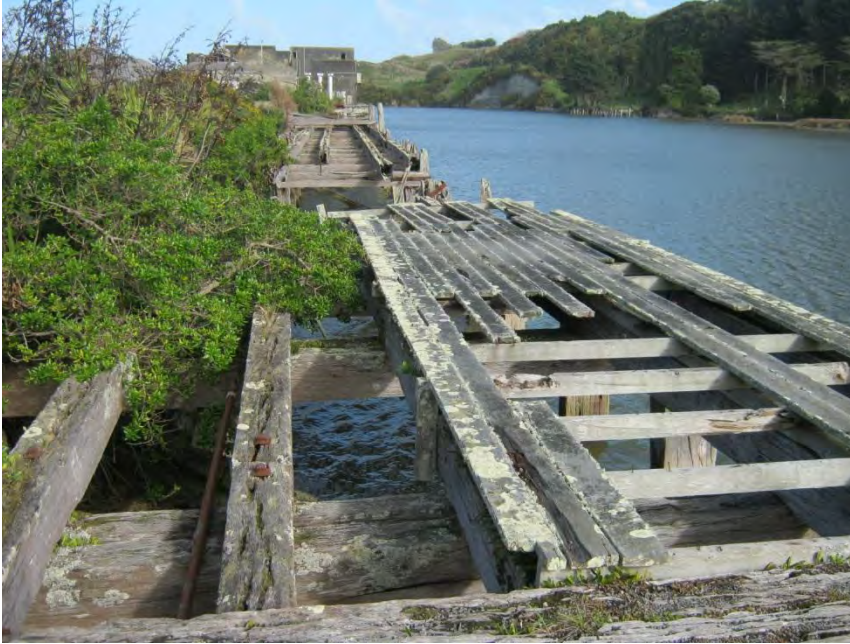
Photo 14 Old Patea wharf (March 2013)
