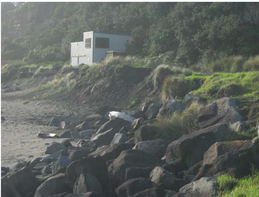
Photo 2 Rip rap seawall, Middleton Bay (May, 2014)
