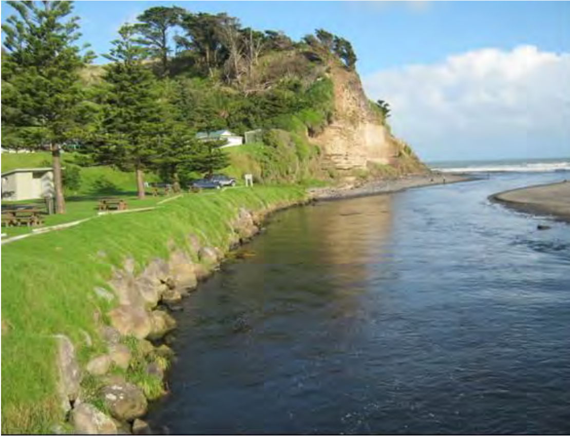
Photo 3 Looking upstream along rock protection works in the Kaupokonui Stream (May 2014)
