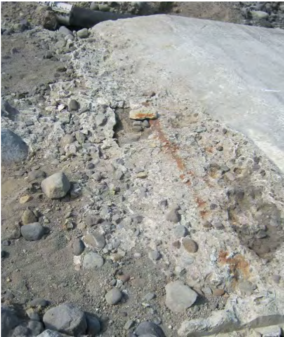
Photo 10 Top section of the Opunake Beach boat ramp (March 2012)
