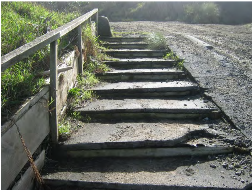
Photo 15 Access to Caves Beach, Waverley (May 2014)
