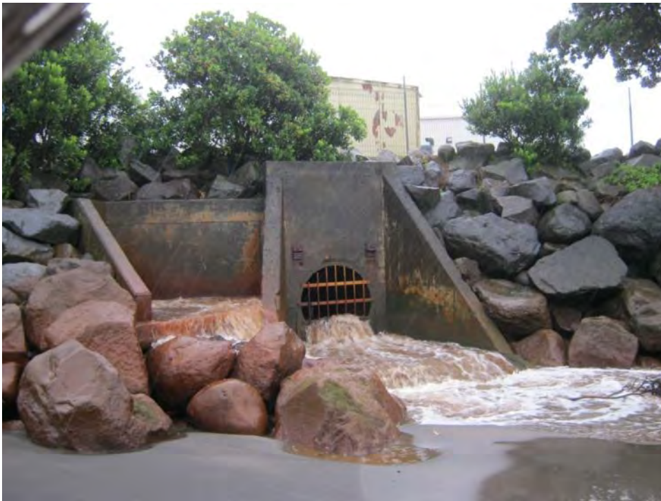
Photo 15 Hongihongi Stream outlet structure (April 2012)
