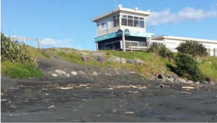
Photo 34 Rock protection works in front of Fitzroy Surf Lifesaving Club (top May 2014, bottom May 2015)
