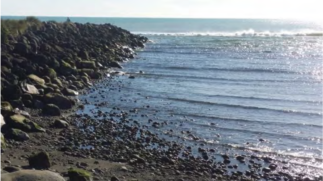
Photo 10 Waiwhakaiho groyne (May 2015)
