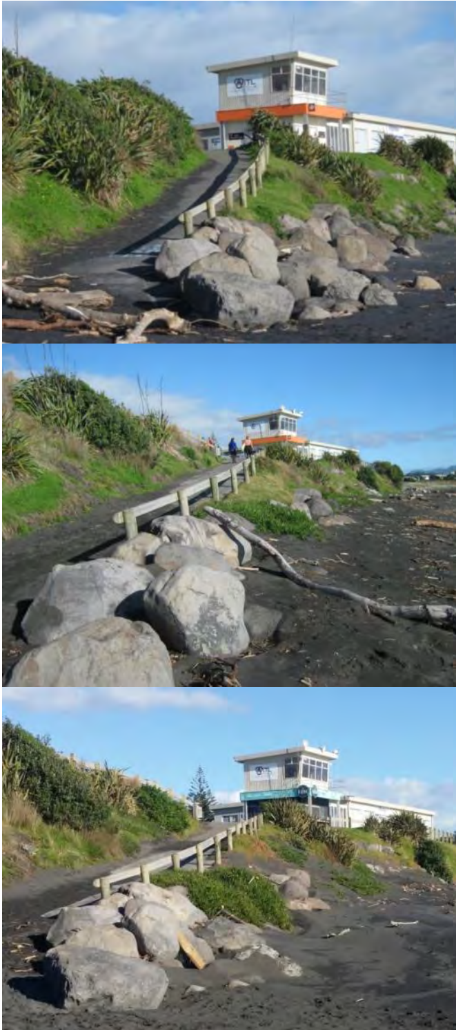
Photo 33 Boat ramp and rock protection works in front of Fitzroy Surf Lifesaving Club (top June 2013, middle May 2014, bottom May 2015)
