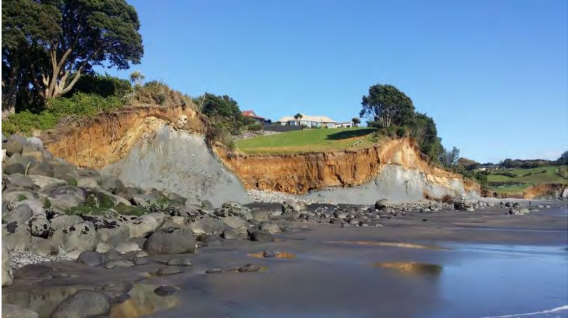
Photo 7 Eroding cliffs to the west of the seawall at Onaero (May 2015)
