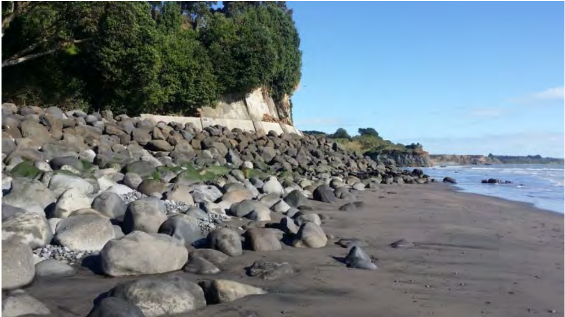
Photo 23 Onaero seawall (May 2015)
