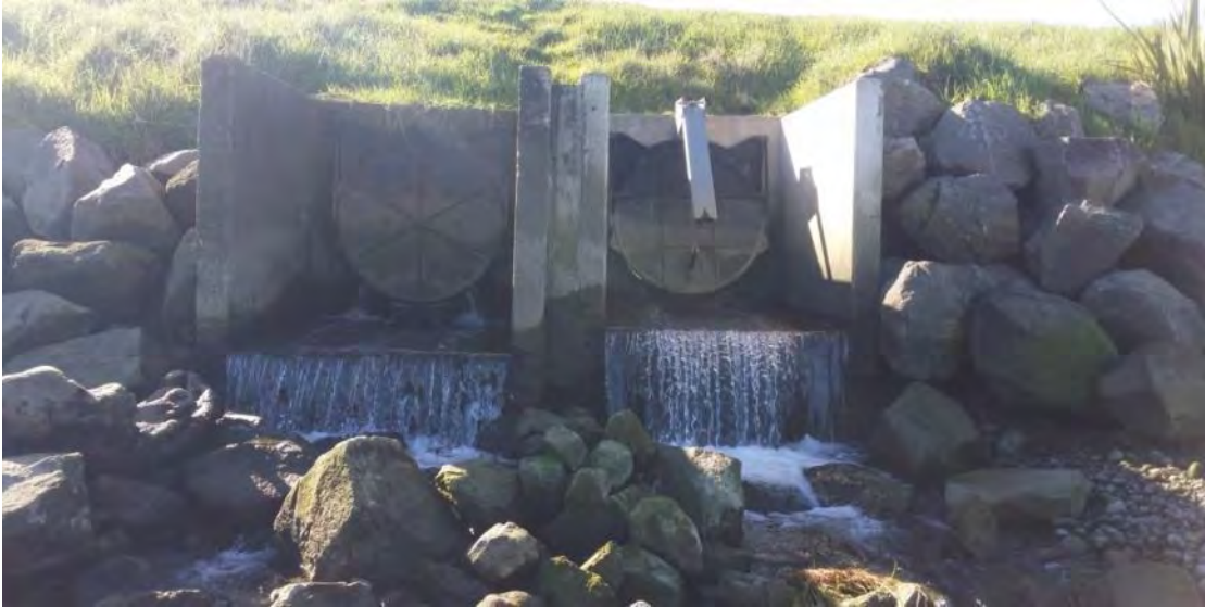
Photo 24 Stormwater outlet structure downstream of Atkinson Street (May 2015)
