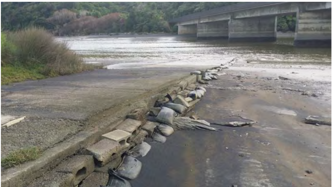
Photo 2 Boat ramp at Tongaporutu (May 2015)
