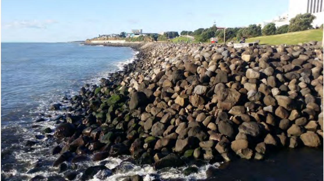
Photo 39 Foreshore rip rap protection between Te Henui and Kawaroa (May 2015)
