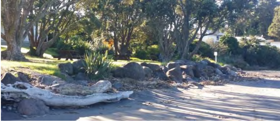
Photo 17 Riverbank protection works by the boat ramp (May 2015)
