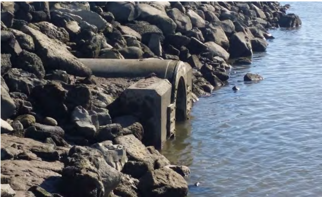
Photo 14 Stormwater outlet structure McNaughton Street, Waitara (May 2015)
