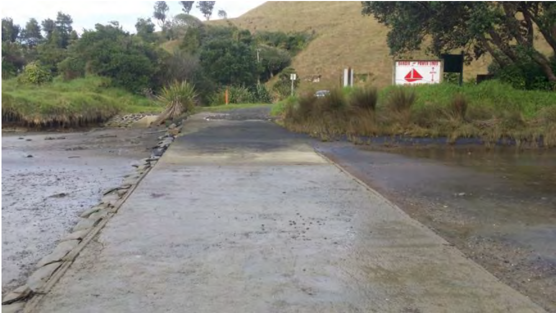
Photo 16 Boat ramp at Tongaporutu (May 2015)
