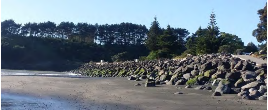
Photo 20 Urenui Beach rip rap protection east seawall (May 2015)
