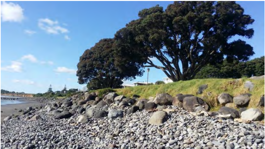
Photo 28 Bell Block seawall (May 2015)
