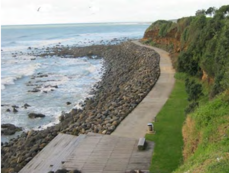
Photo 13 New Plymouth coastal walkway with rip rap seawall protection (May 2014)
