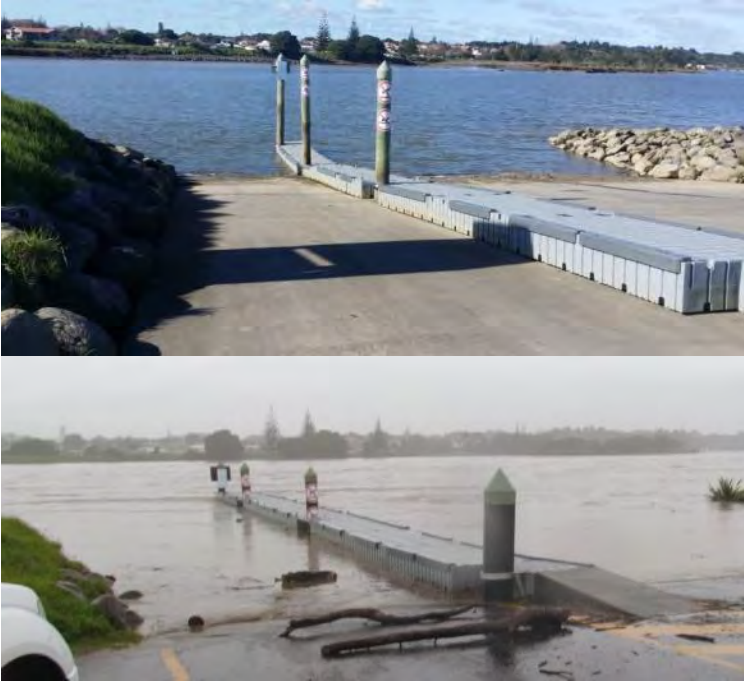
Photo 26 Boat ramp at Waitara (May 2015 and June 2015)
