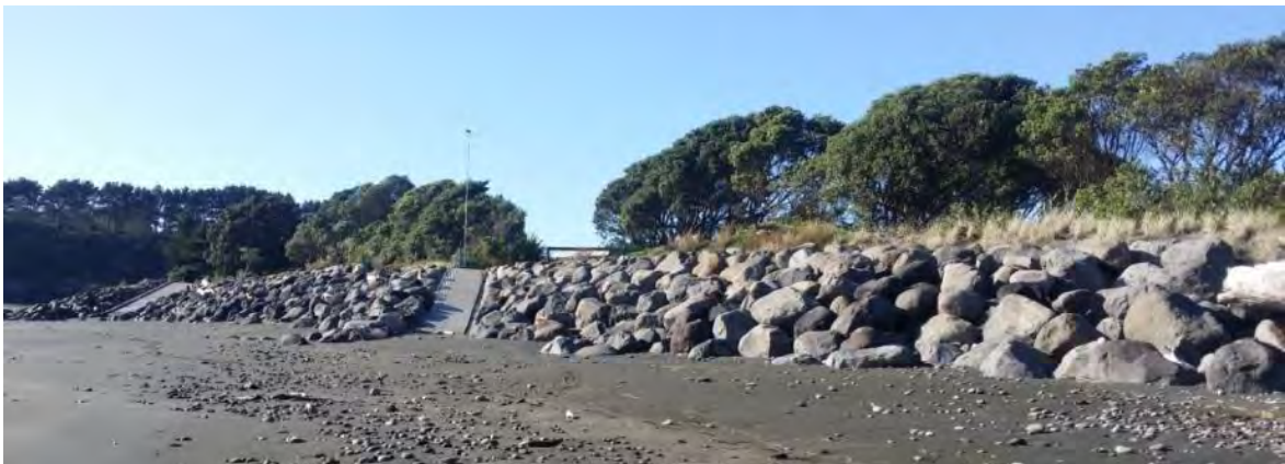
Photo 5 Urenui beach access and rip rap wall (May 2015)
