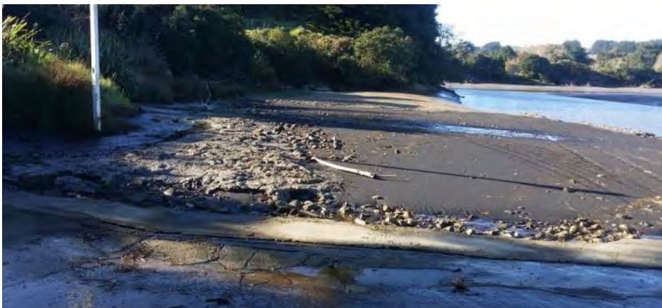
Photo 19 Riverbank protection works around the Manager's residence (May 2015)
