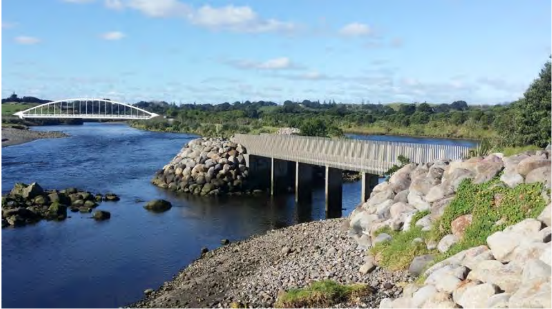
Photo 31 Footbridge over the Waiwhakaiho River (May 2015)
