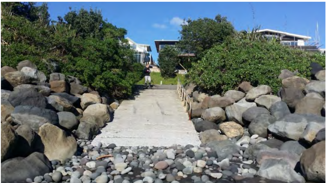
Photo 29 Bell Block access ramp to beach (May 2015)
