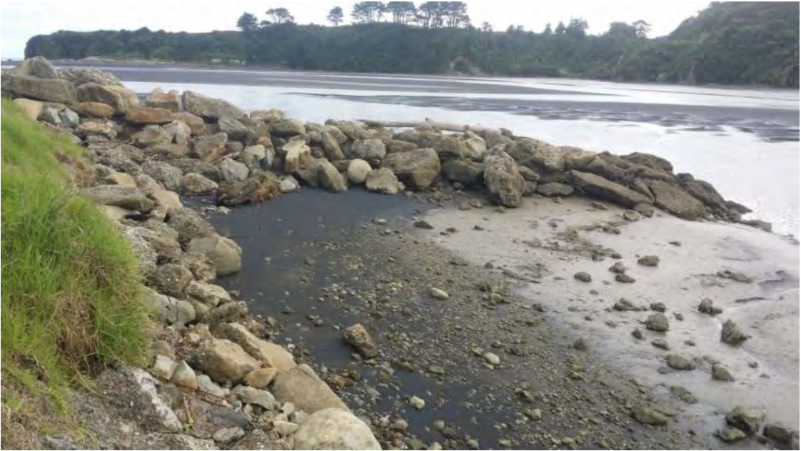
Photo 1 Rock groyne at Tongaporutu (May 2015)
