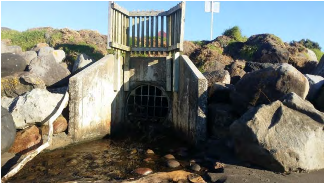
Photo 40 The Bayly road stormwater outfall on Ngamotu Beach (May 2015)
