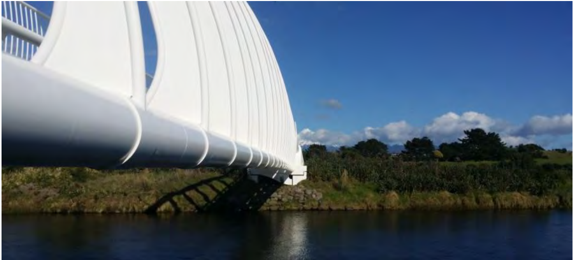
Photo 32 Te Rewarewa bridge over the Waiwhakaiho River (May 2015)
