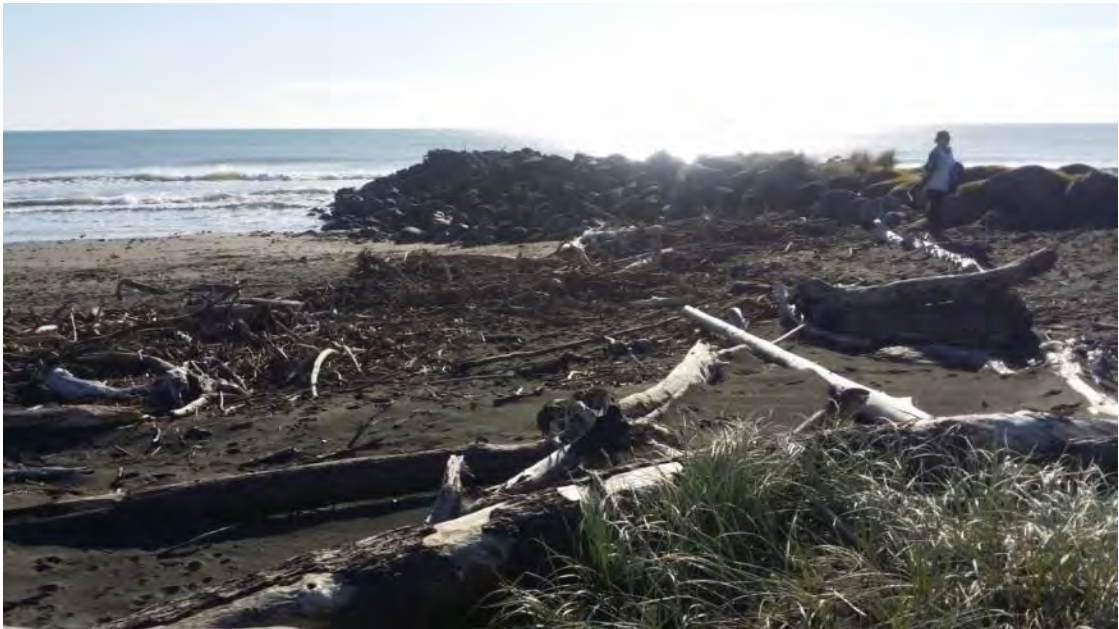
Photo 30 Waiwhakaiho groyne (May 2015)
