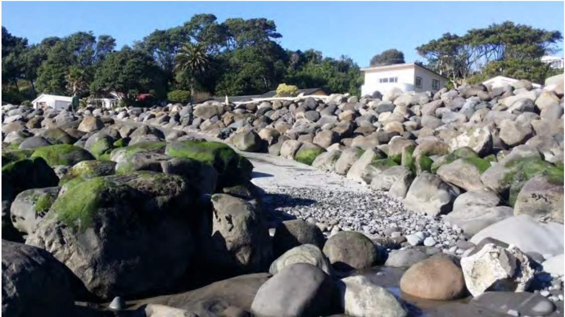
Photo 6 Onaero Beach seawall and boat ramp (May 2015)
