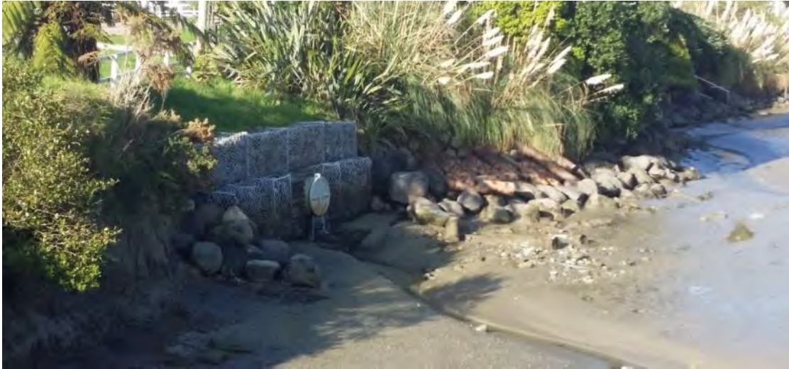
Photo 22 Urenui rip rap (May 2015)
