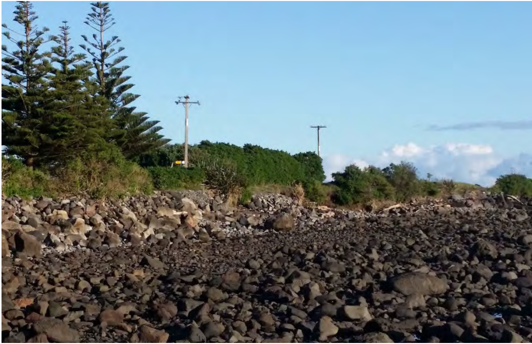
Photo 1 Bayly Road seawall (May, 2015)
