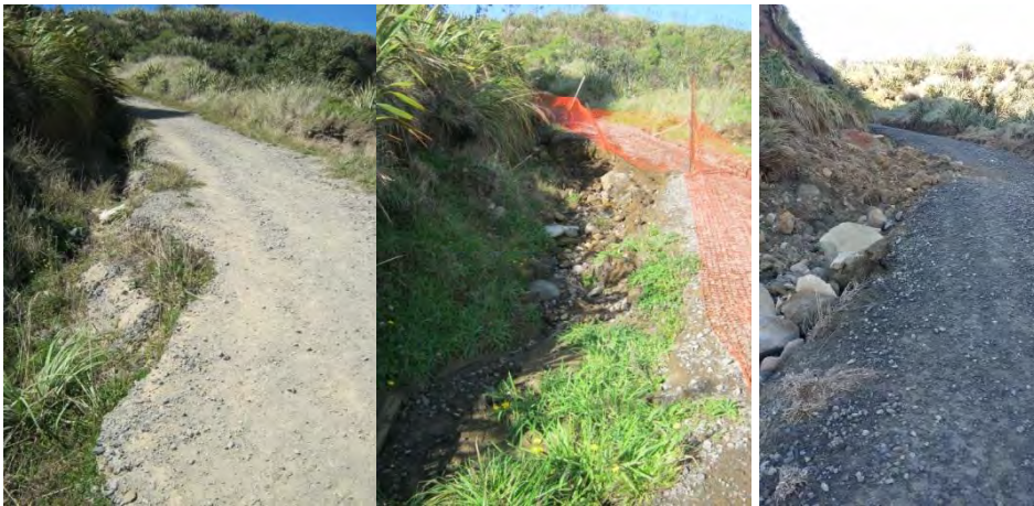
Photo 12 Erosion of beach track at the end of Denby Road left March 2013, centre May 2014, right May 2015
