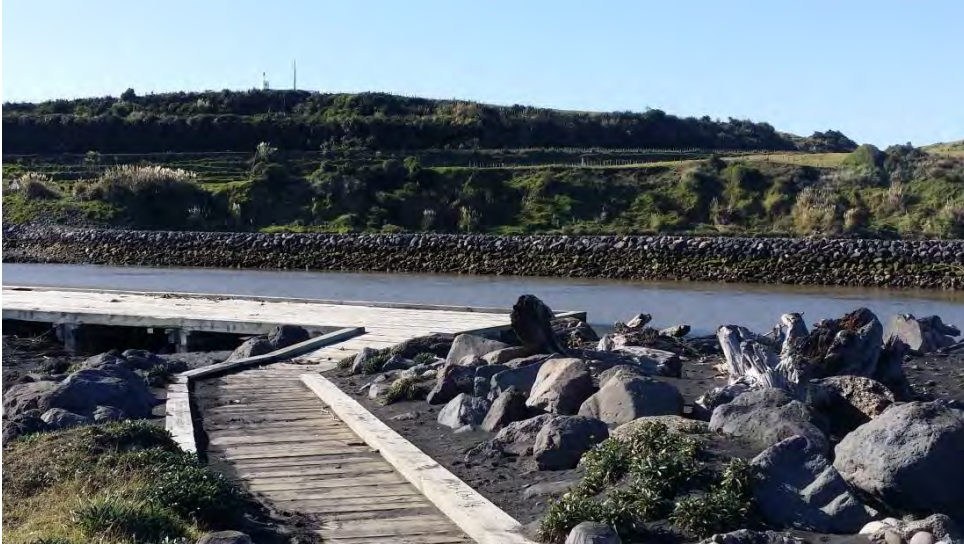
Photo 13 Training wall at Patea (May, 2015)
