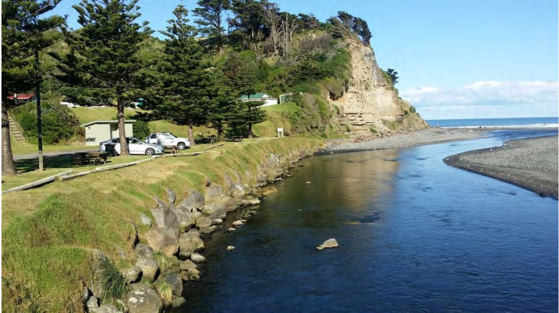
Photo 3 Looking upstream along rock protection works in the Kaupokonui Stream (May 2015)
