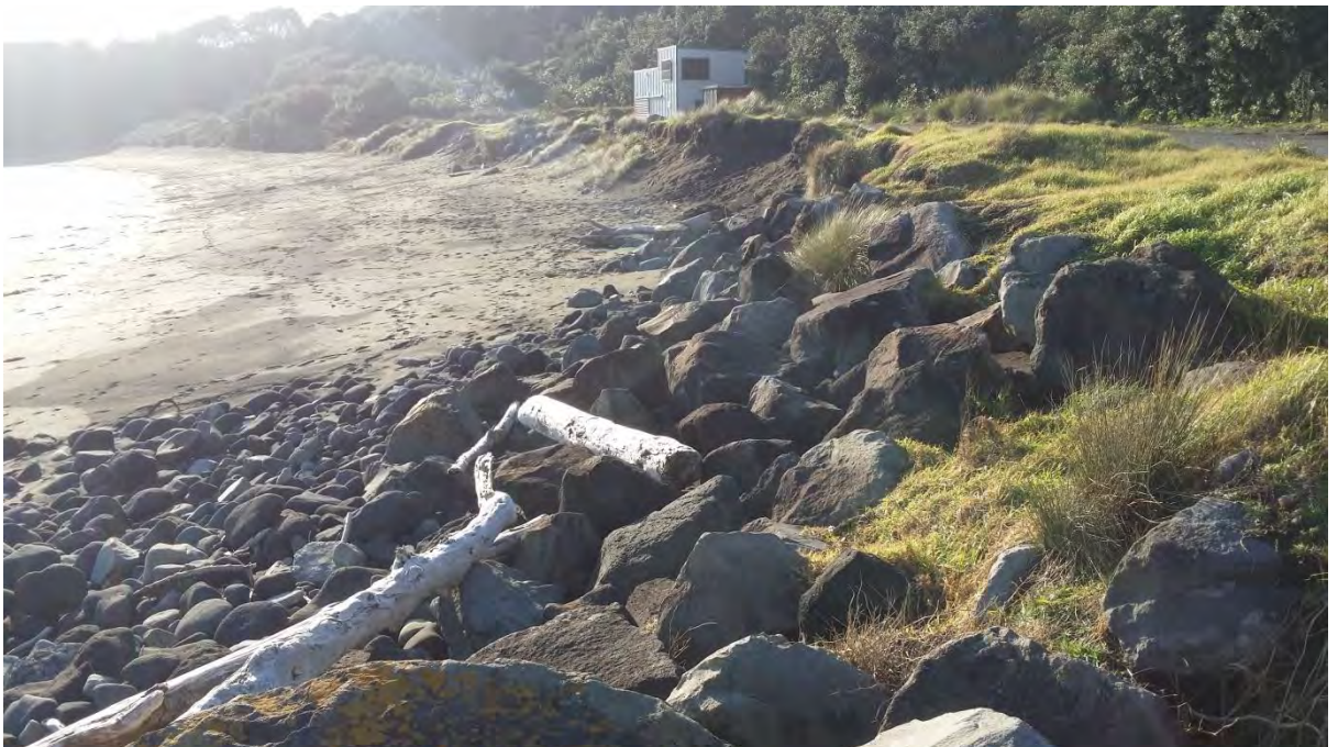
Photo 2 Rip rap seawall, Middleton Bay (May, 2015)
