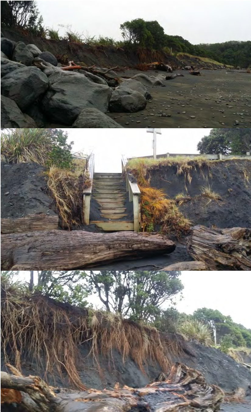
Photo 43 Erosion at the west end of Urenui Beach June 2016
