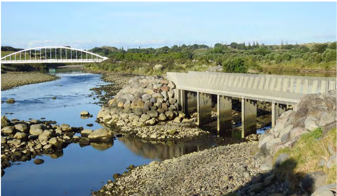
Photo 31 Footbridge over the Waiwhakaiho River (April 2016)
