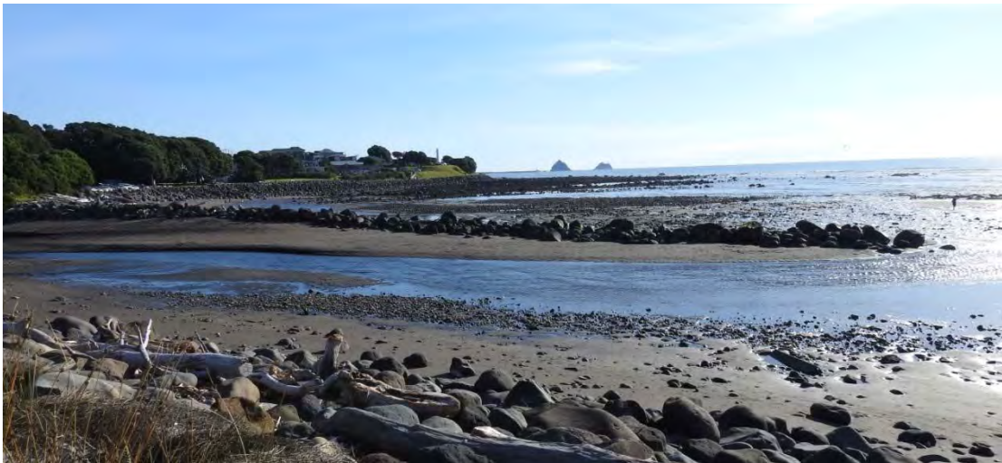
Photo 12 The Te Henui groyne (April 2016)
