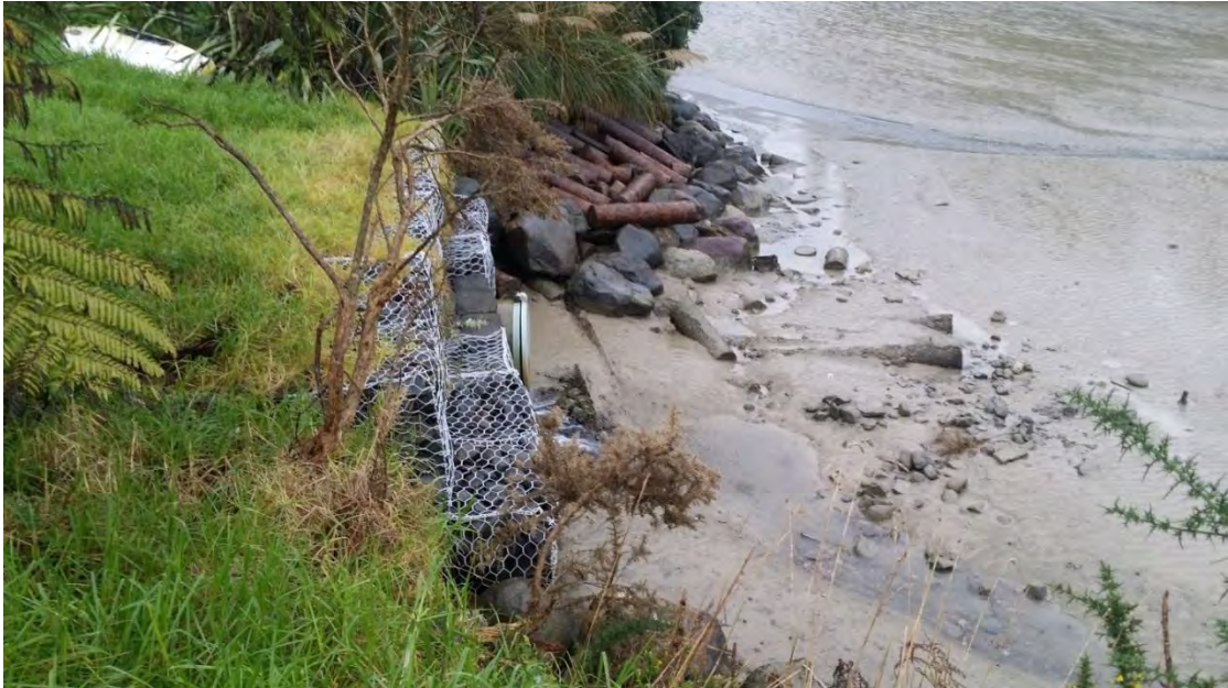
Photo 22 Urenui rip rap (June 2016)
