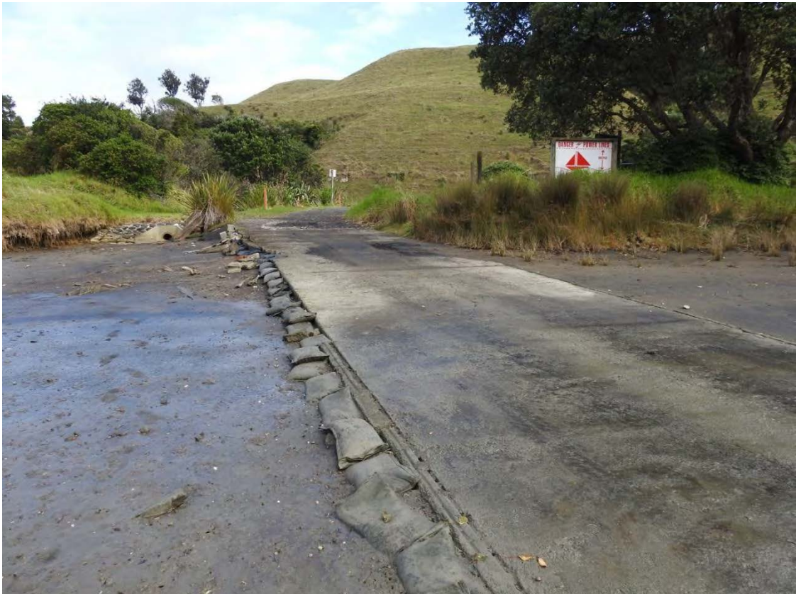
Photo 16 Boat ramp at Tongaporutu (May 2016)
