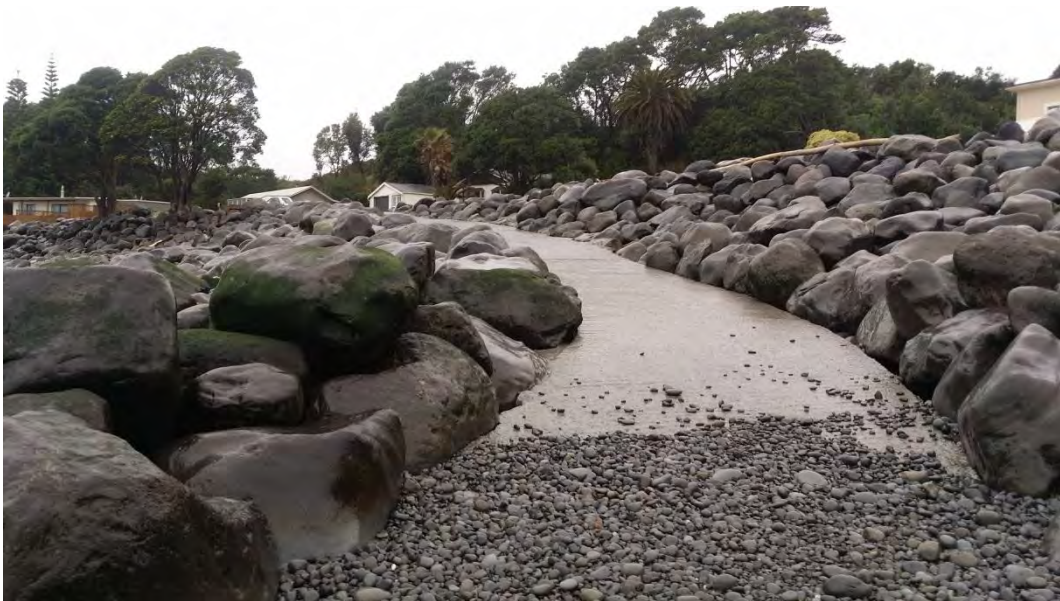
Photo 6 Onaero Beach seawall and boat ramp (June 2016)
