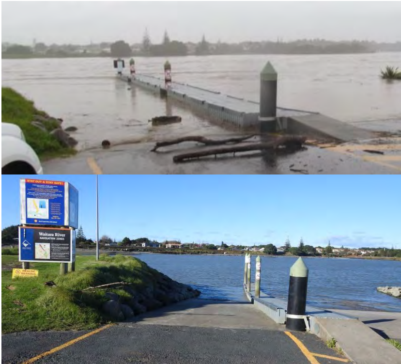
Photo 26 Boat ramp at Waitara (top June 2015, bottom June 2016)
