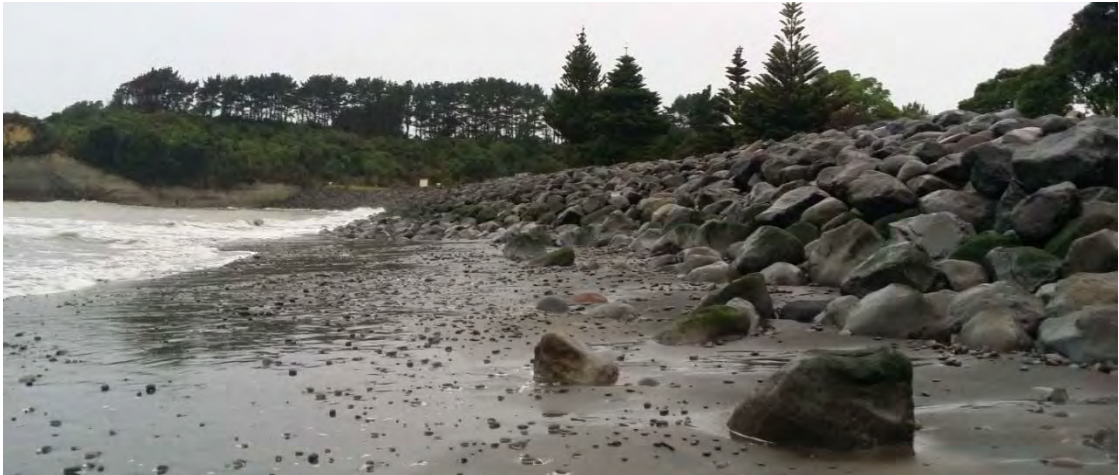
Photo 20 Urenui Beach rip rap protection east seawall (June 2016)
