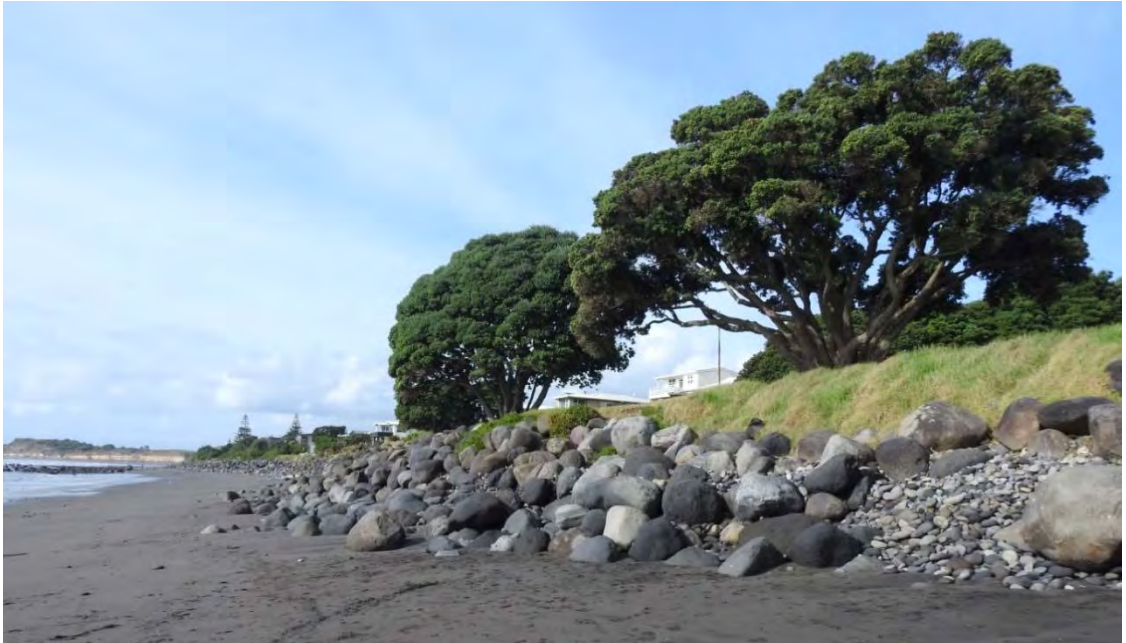
Photo 28 Bell Block seawall (May 2016)
