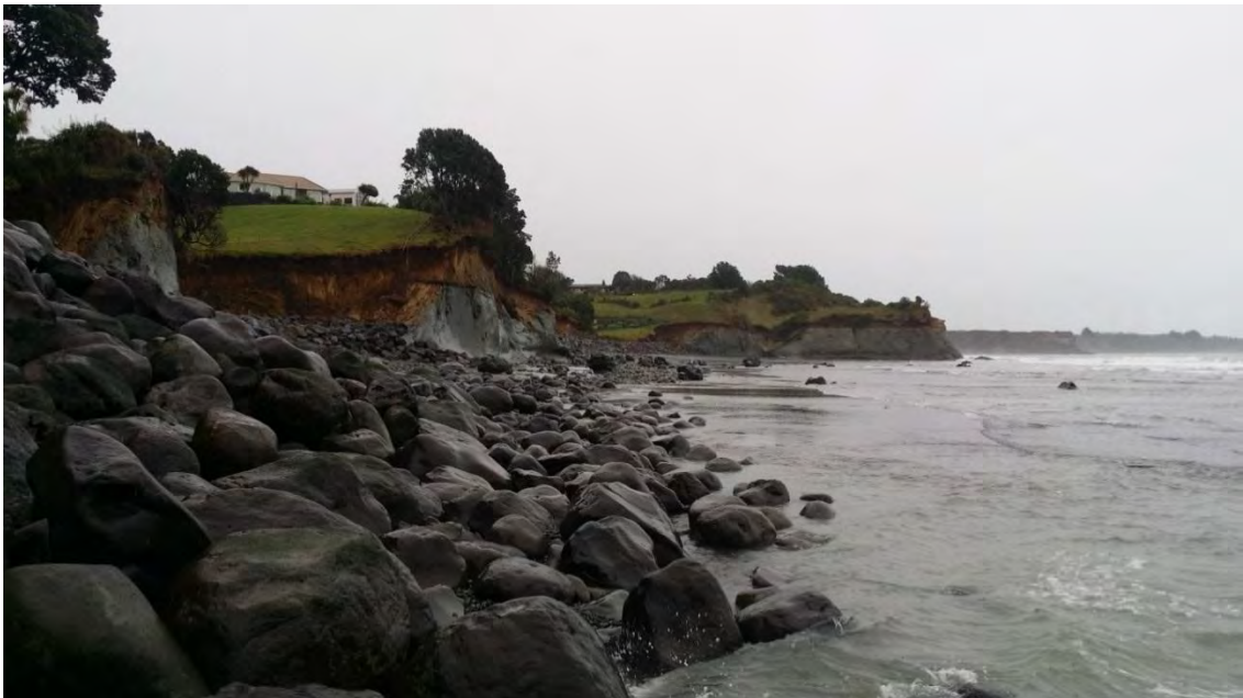
Photo 23 Onaero seawall (June 2016)
