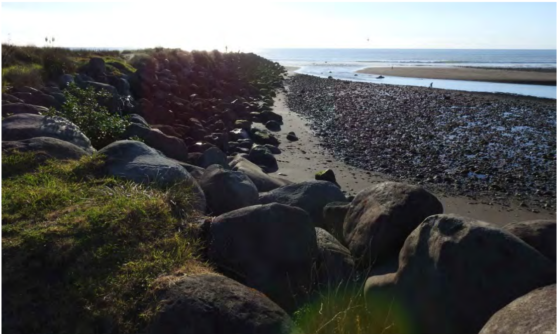
Photo 10 Waiwhakaiho groyne (April 2016)
