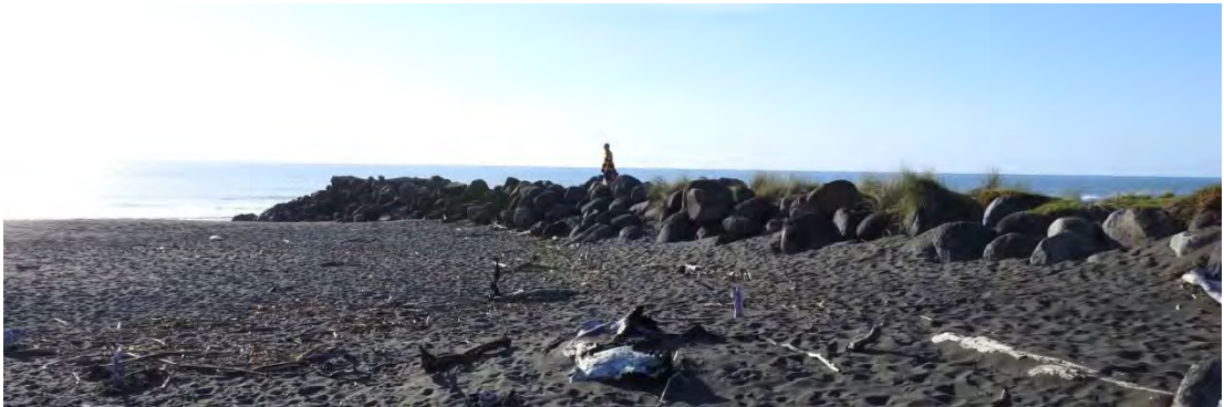
Photo 30 Waiwhakaiho groyne (April 2016)
