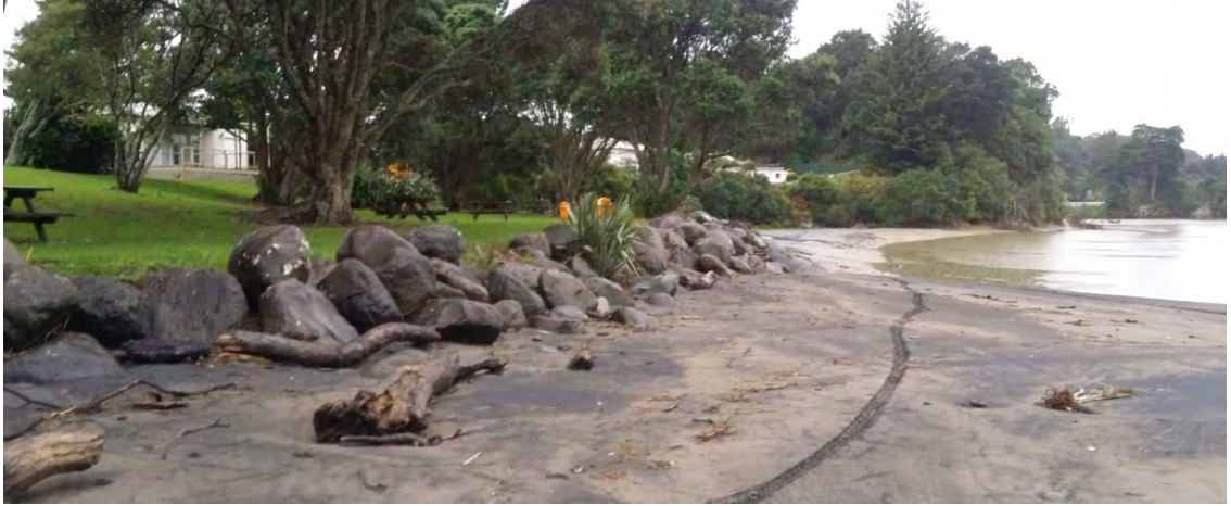
Photo 17 Riverbank protection works by the boat ramp (June 2016)
