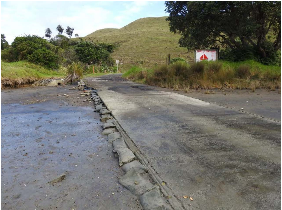
Photo 2 Boat ramp at Tongaporutu (May 2016)
