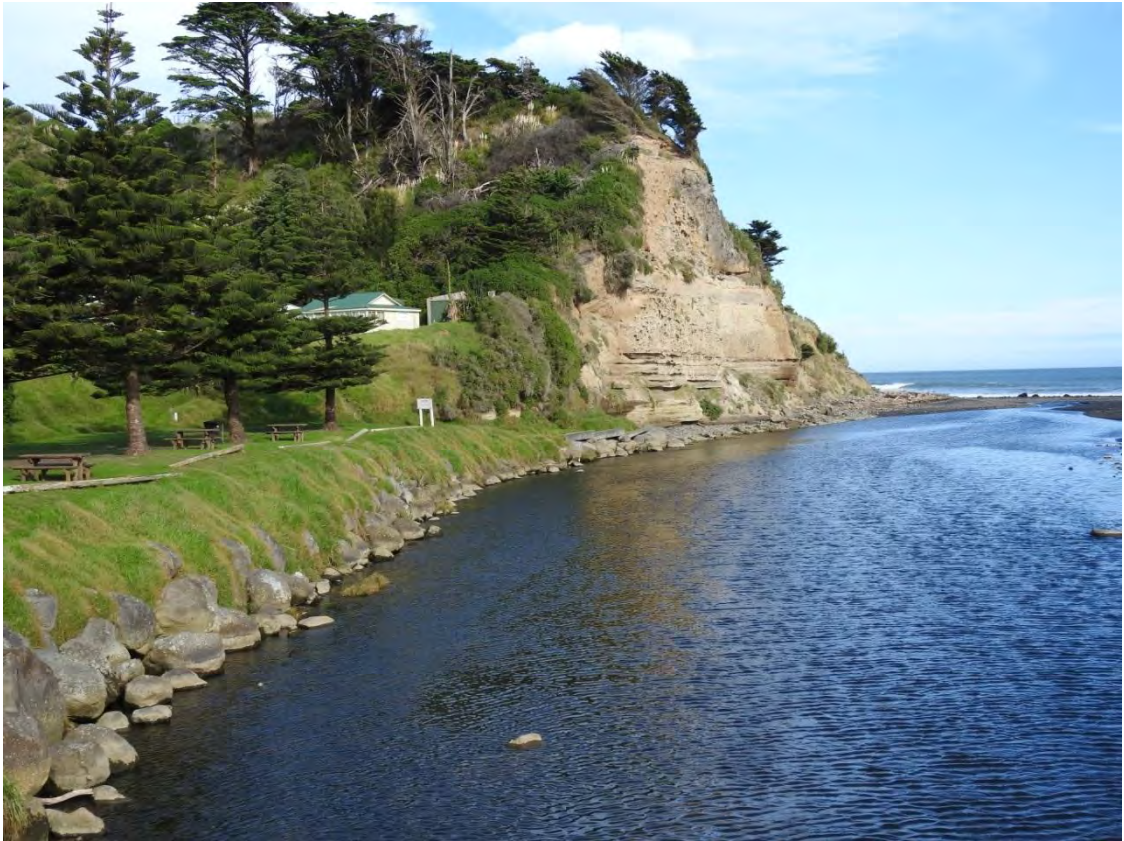
Photo 3 Looking upstream along rock protection works in the Kaupokonui Stream (May 2015)
