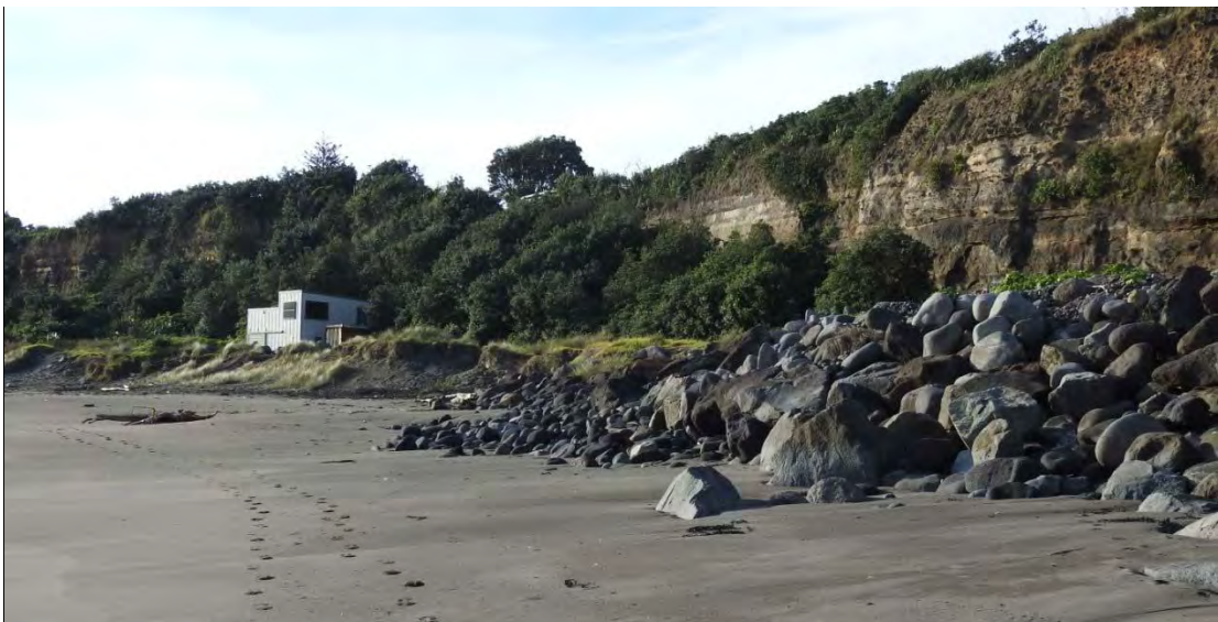
Photo 2 Rip rap seawall, Middleton Bay (May, 2015)
