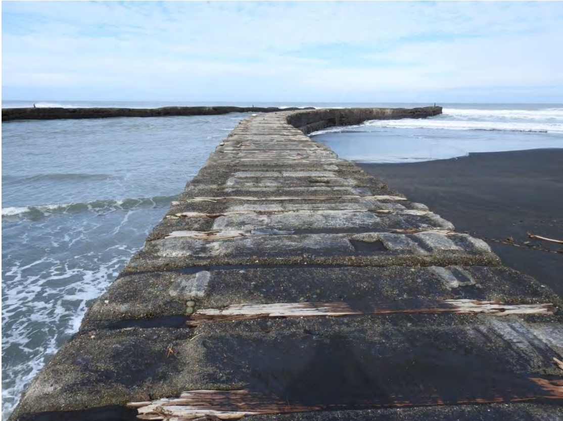
Photo 5 Patea groynes (May 2016)
