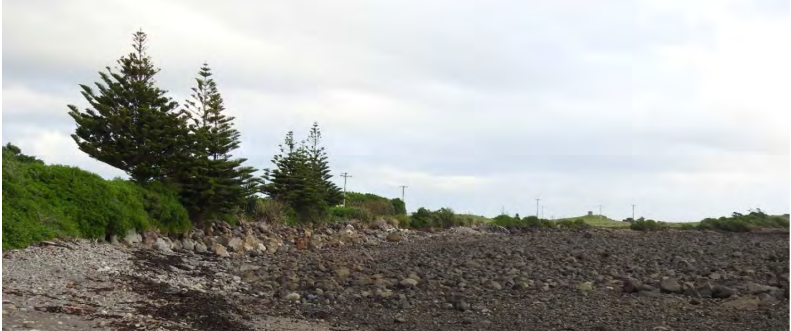
Photo 1 Bayly Road seawall (May, 2016)
