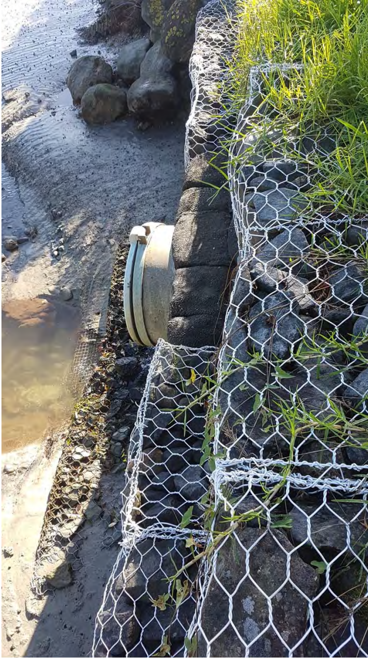
Photo 22 Urenui rip rap (May 2017)
