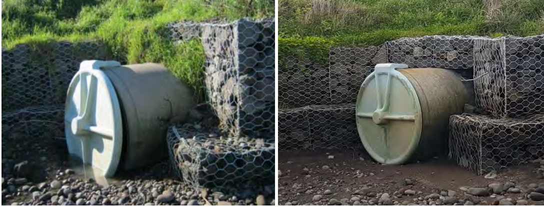
Photo 25 The stormwater outlet by the Atkinson Street/East Quay intersection (June 2013 and May 2017)
