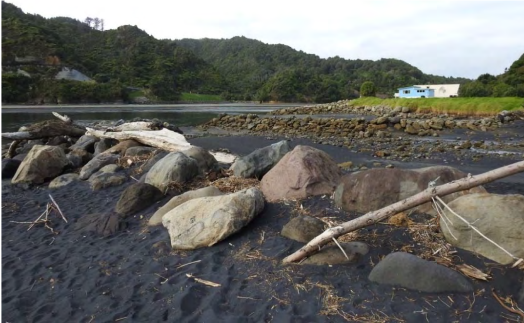
Photo 1 Rock groyne at Tongaporutu (May 2016)
