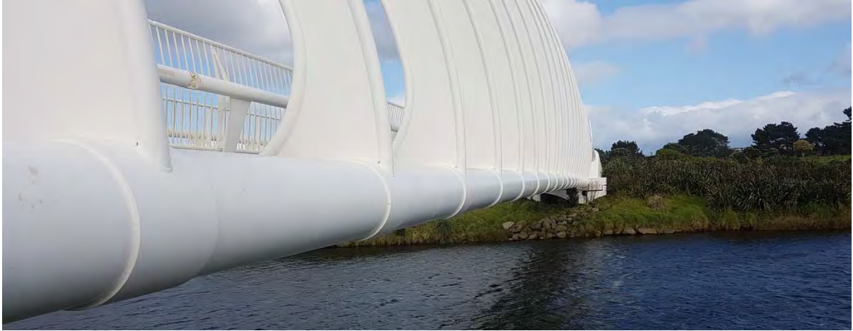
Photo 32 Te Rewarewa bridge over the Waiwhakaiho River (May 2017)
