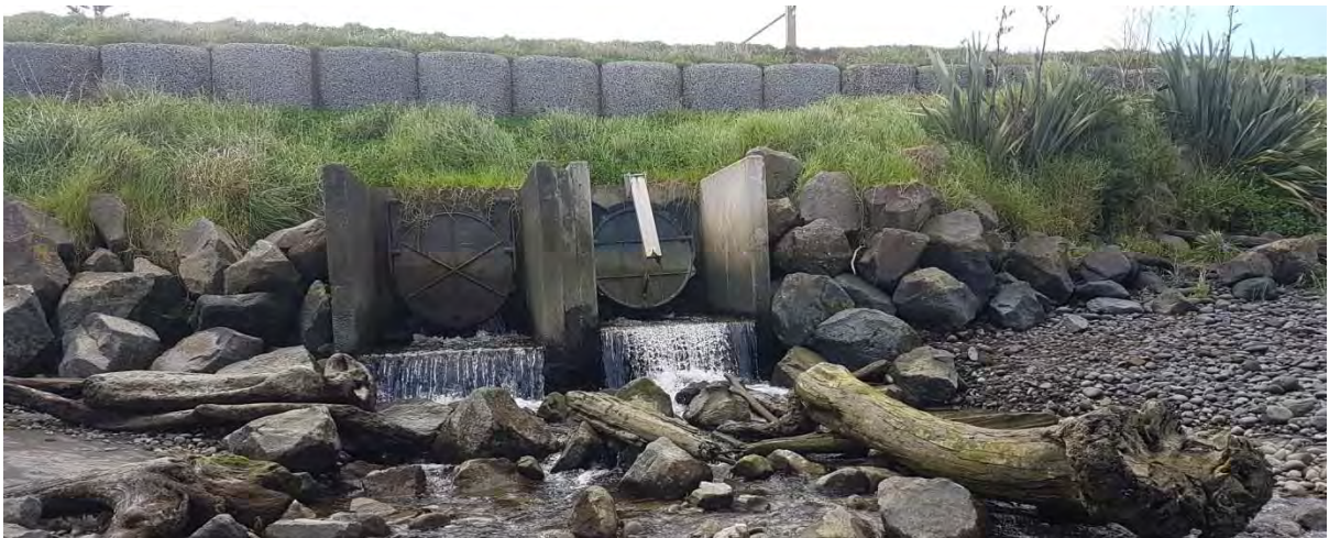
Photo 24 Stormwater outlet structure downstream of Atkinson Street (May 2017)
