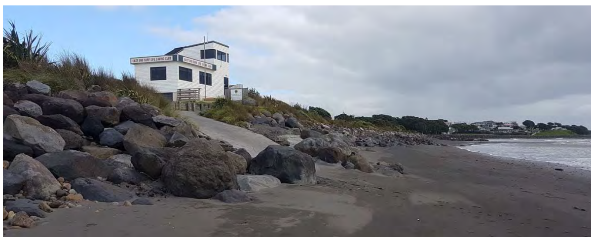
Photo 11 Rip rap seawall in front of East End Surf Life Saving Club (May 2017)
