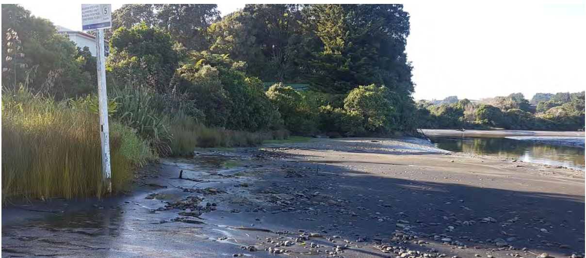
Photo 19 Riverbank protection works around the Manager's residence (May 2017)
