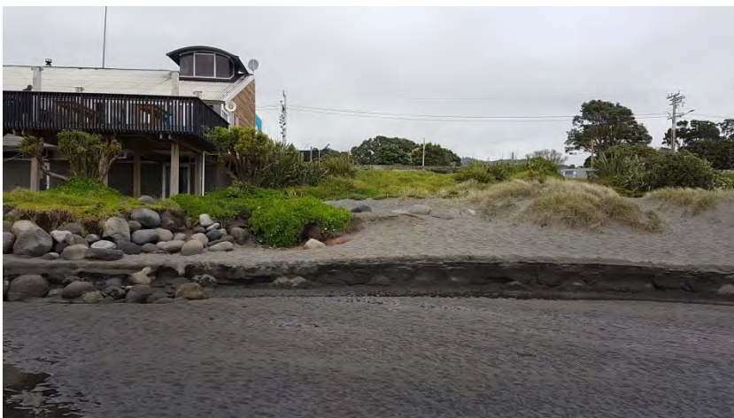
Photo 42 Protection works in front of Oakura Surf Life Saving Club showing erosion of the bank/dunes to the west of the club (top June 2015, middle April 2016, bottom May 2017)
