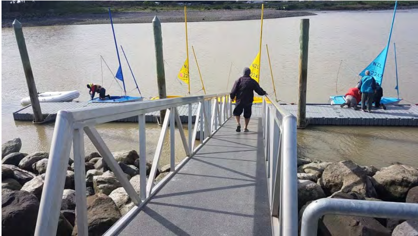
Photo 27 Jetty at Waitara (top June 2015, bottom May 2017)
