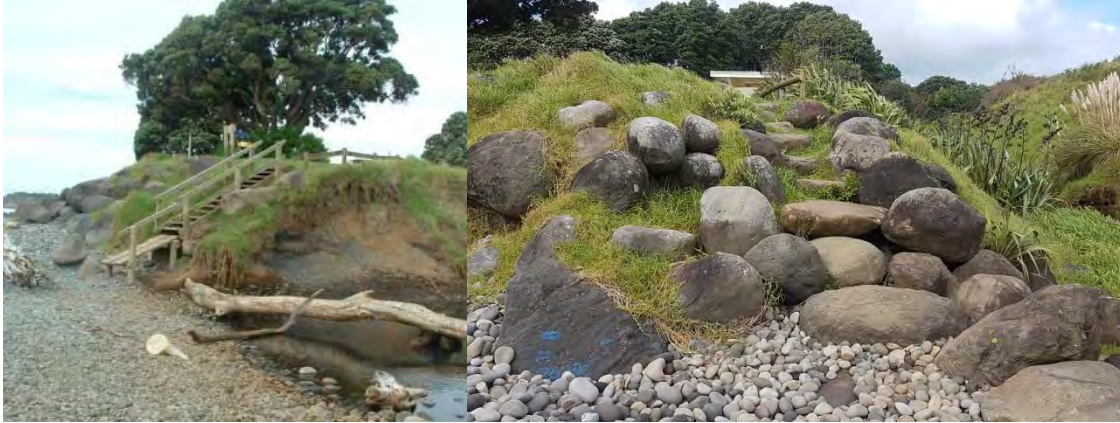
Photo 9 Step access to Bell Block Beach (previous wooden steps July 2005 and current rock steps May 2017)
