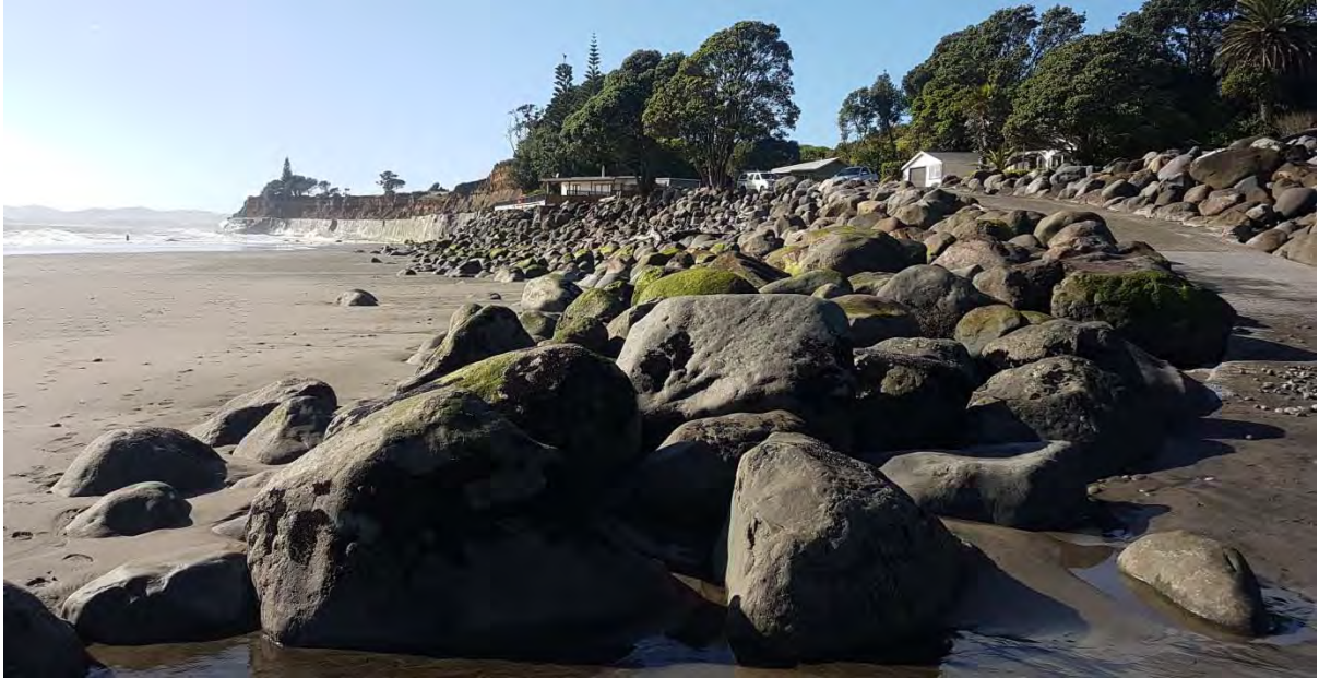
Photo 23 Onaero seawall (May 2017)
