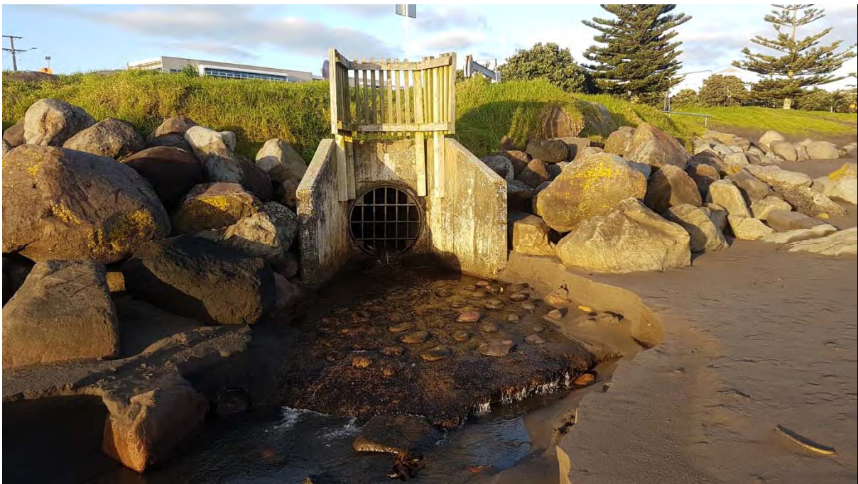
Photo 40 The Bayly Road stormwater outfall on Ngamotu Beach (May 2017)
