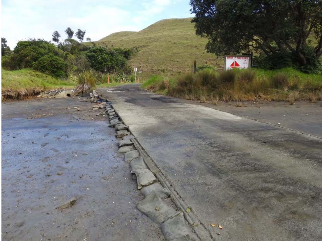
Photo 16 Boat ramp at Tongaporutu (May 2016)
