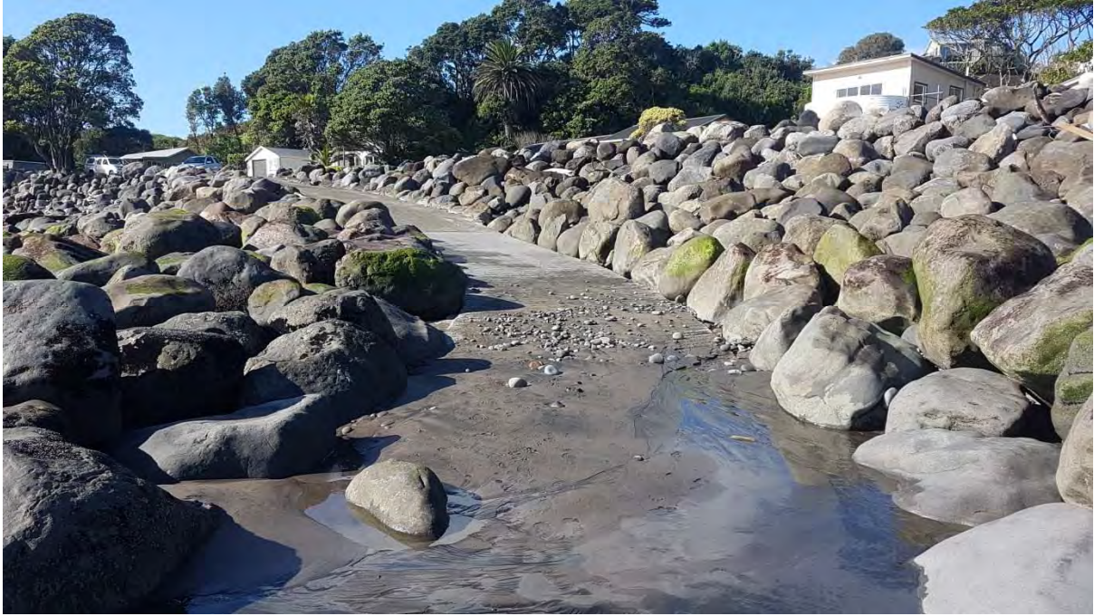
Photo 6 Onaero Beach seawall and boat ramp (May 2017)
