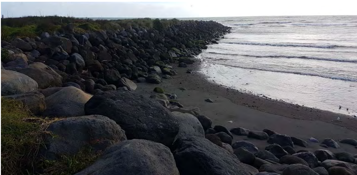
Photo 10 Waiwhakaiho groyne (May 2017)
