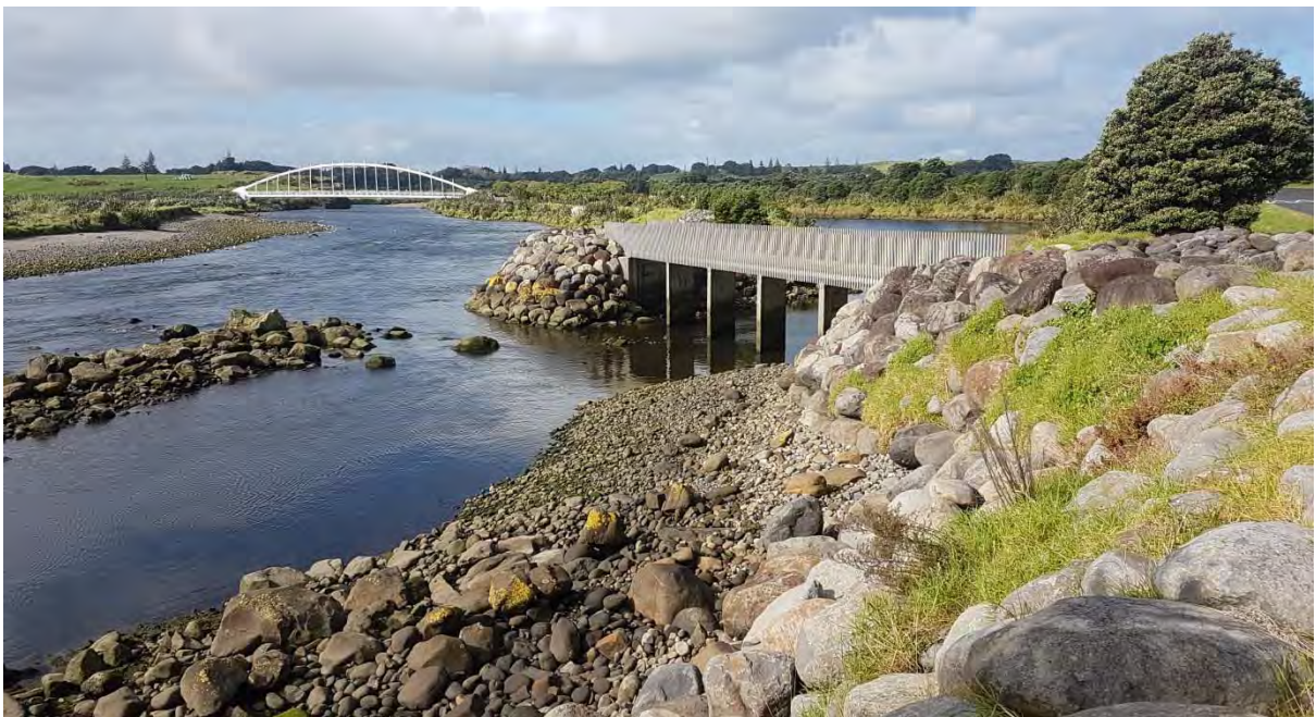
Photo 31 Footbridge over the Waiwhakaiho River (May 2017)
