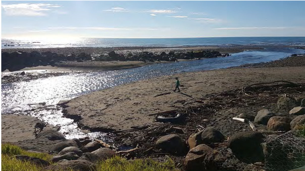
Photo 12 The Te Henui groyne (April 2017)
