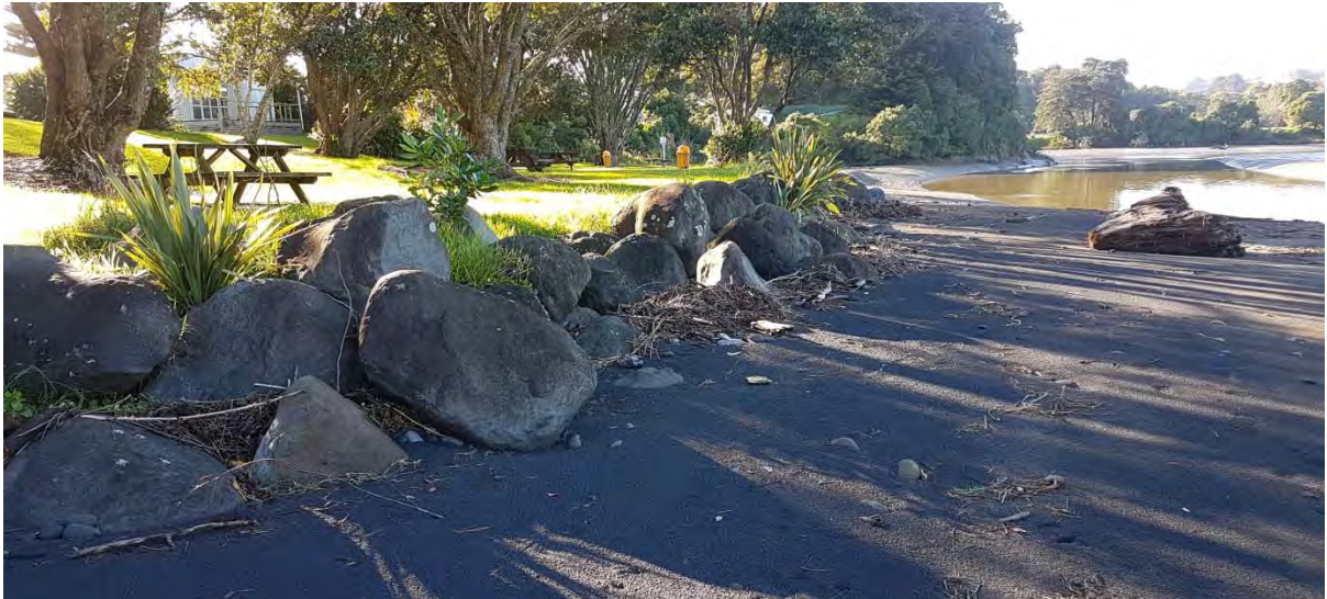
Photo 17 Riverbank protection works by the boat ramp (May 2017)
