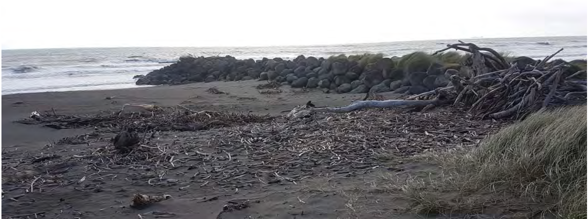
Photo 30 Waiwhakaiho groyne (May 2017)
