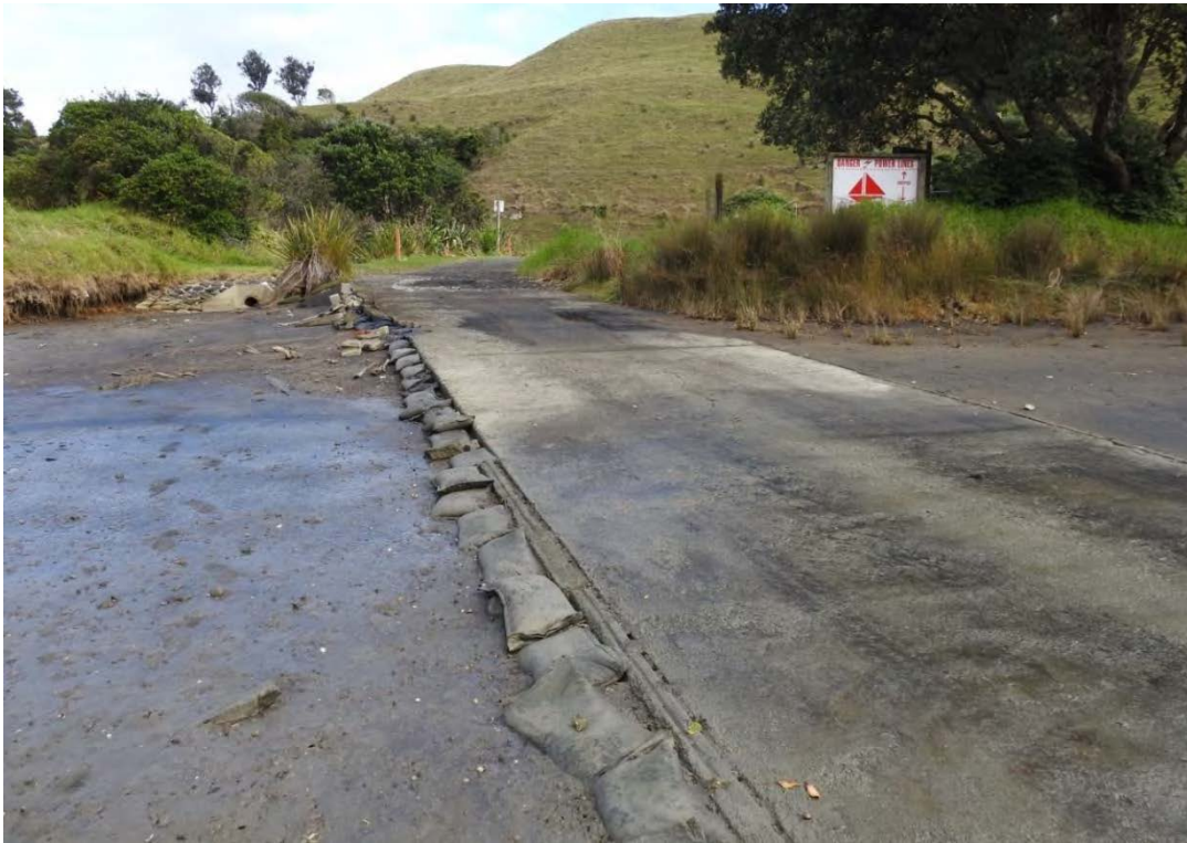
Photo 2 Boat ramp at Tongaporutu (May 2016)
