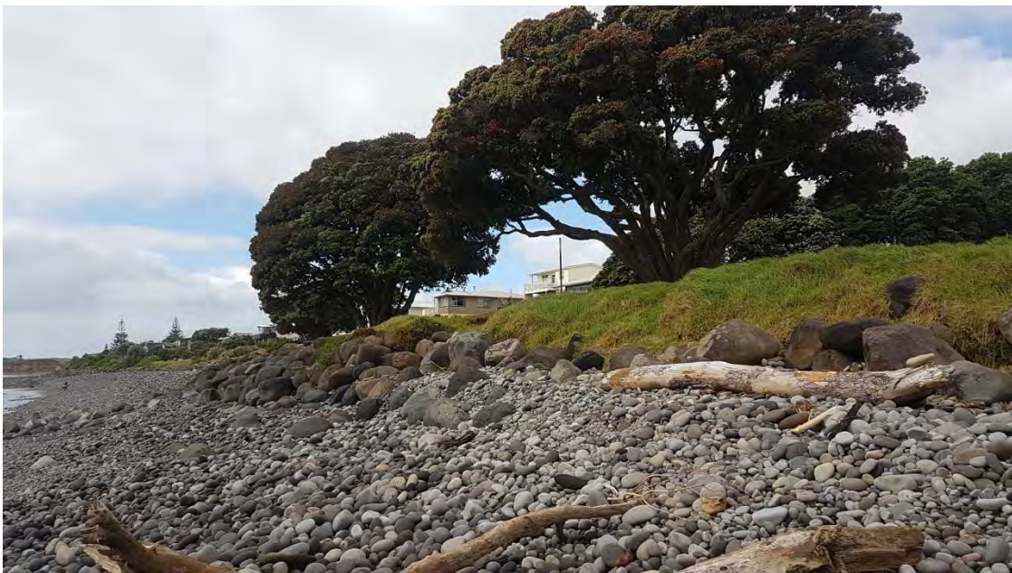
Photo 28 Bell Block seawall (May 2016 showing sandy beach, May 2017 showing cobble beach)
