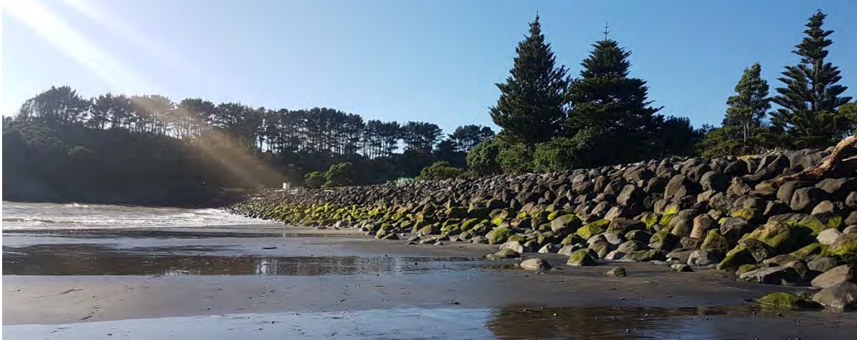
Photo 20 Urenui Beach rip rap protection east seawall (May 2017)
