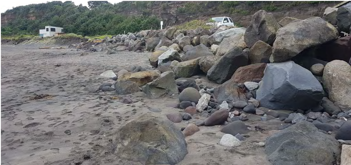
Photo 2 Rip rap seawall, Middleton Bay (April 2017)
