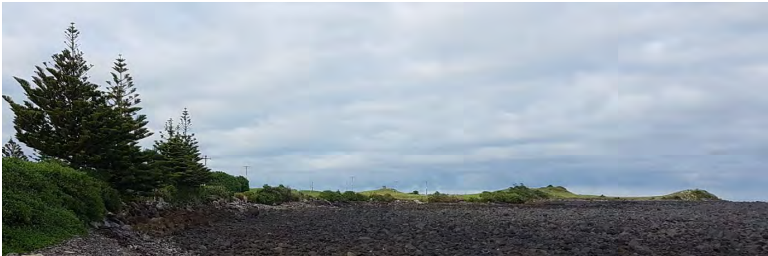
Photo 1 Bayly Road seawall (April 2017)
