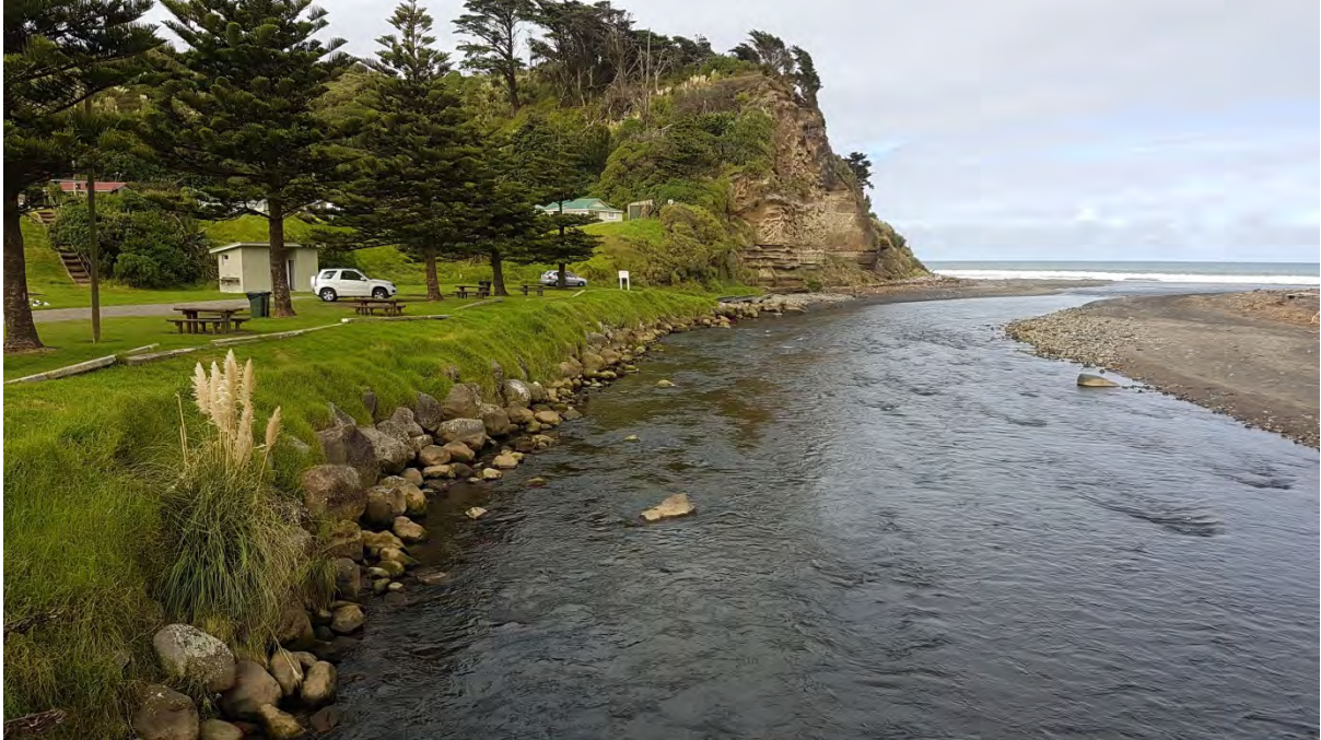
Photo 3 Looking upstream along rock protection works in the Kaupokonui Stream (April 2017)
