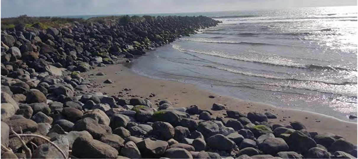
Photo 27 Waiwhakaiho groyne (May 2018)
