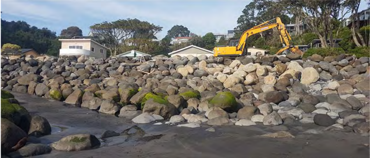
Photo 21 Onaero seawall repairs (May 2018)
