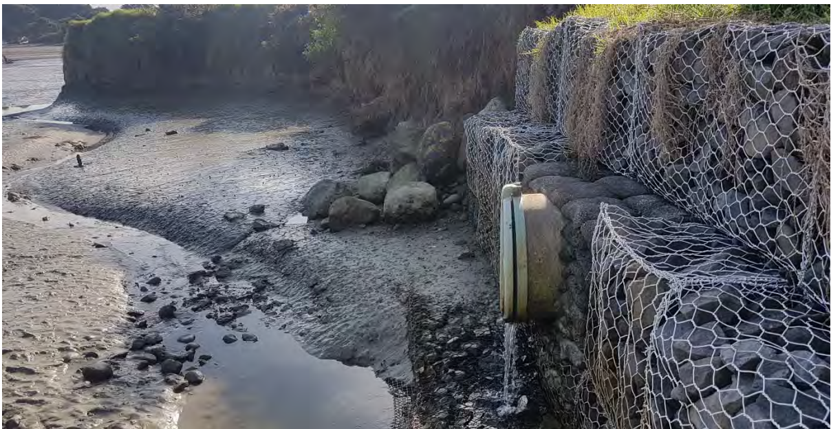
Photo 20 Urenui gabion basket (May 2018)
