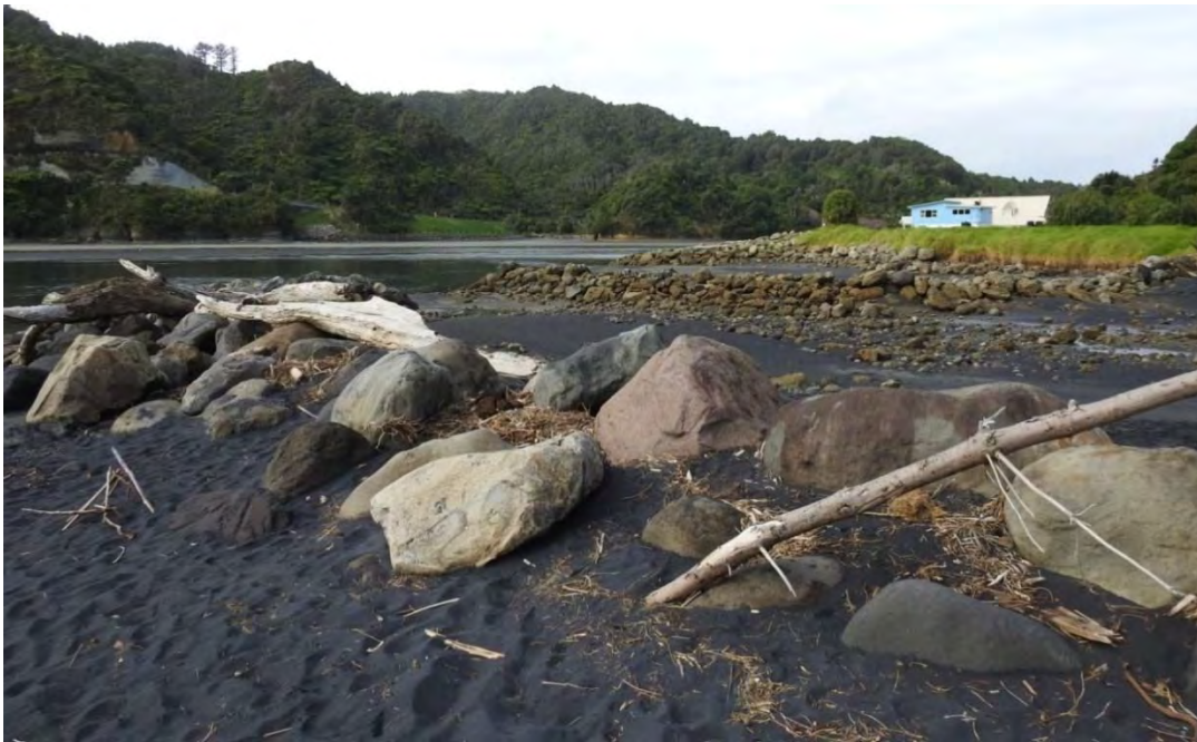
Photo 1 Rock groyne at Tongaporutu (May 2016)
