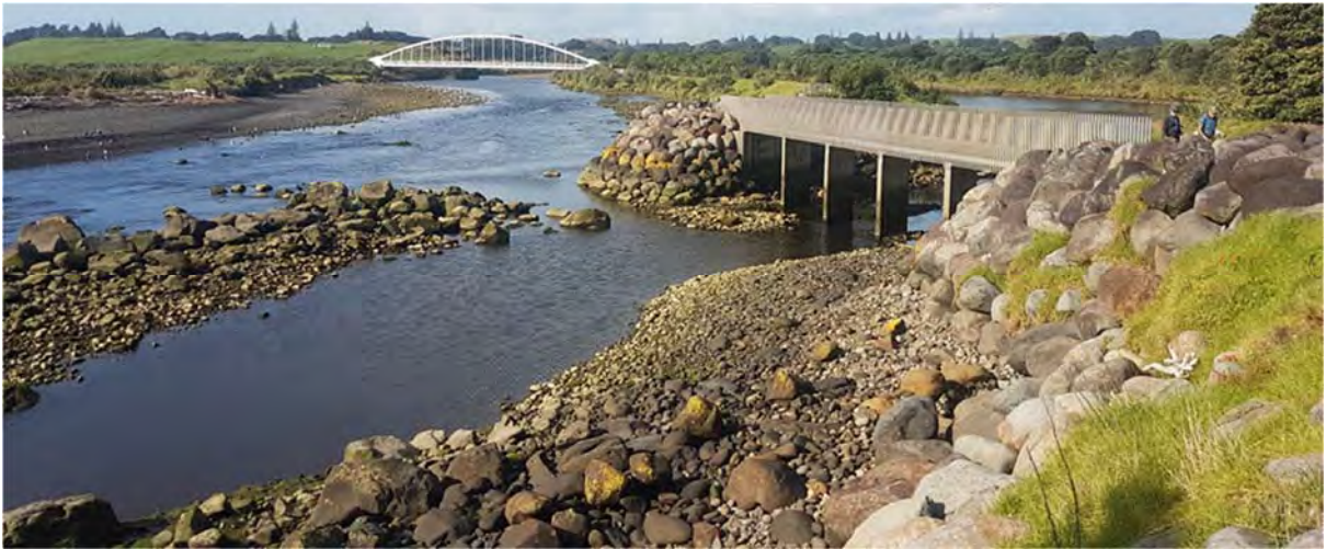
Photo 28 Footbridge over the Waiwhakaiho River (May 2018)
