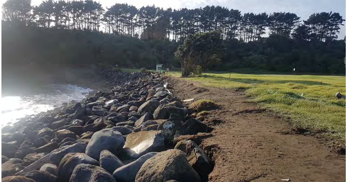
Photo 18 Urenui Beach rip rap protection east seawall (May 2018)
