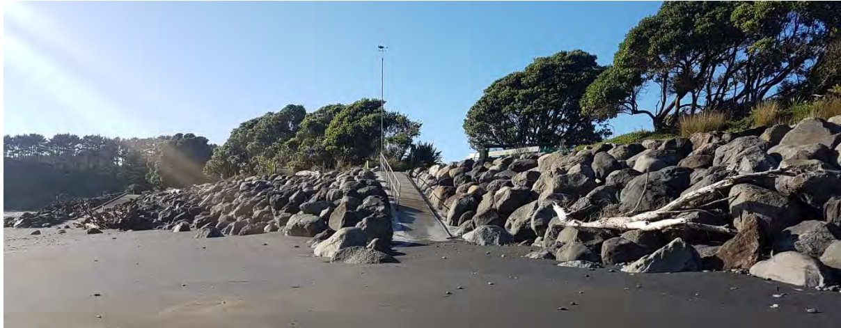
Photo 5 Urenui beach access and rip rap wall (May 2017)
