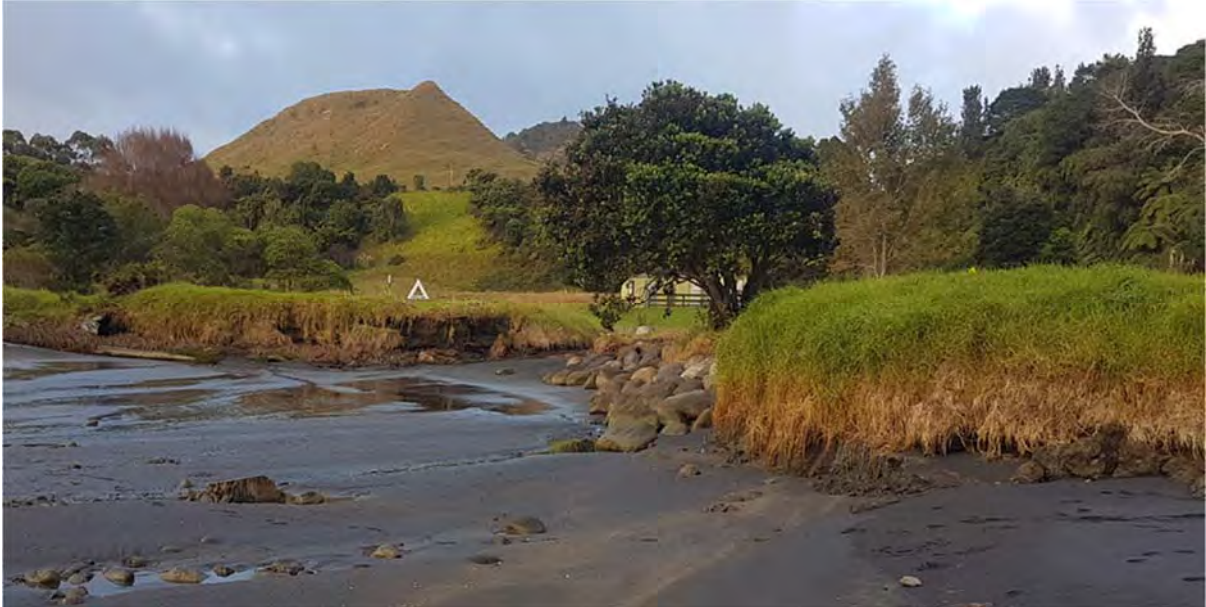
Photo 16 Undercut banks between groynes at Tongaporutu (May 2018)
