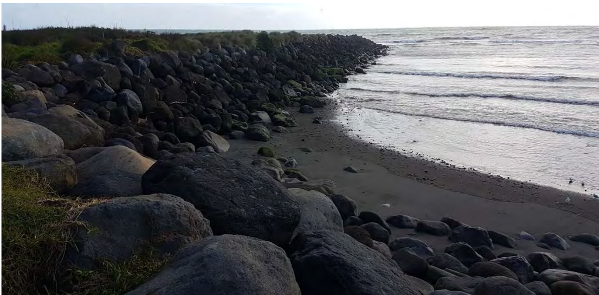
Photo 10 Waiwhakaiho groyne (May 2017)
