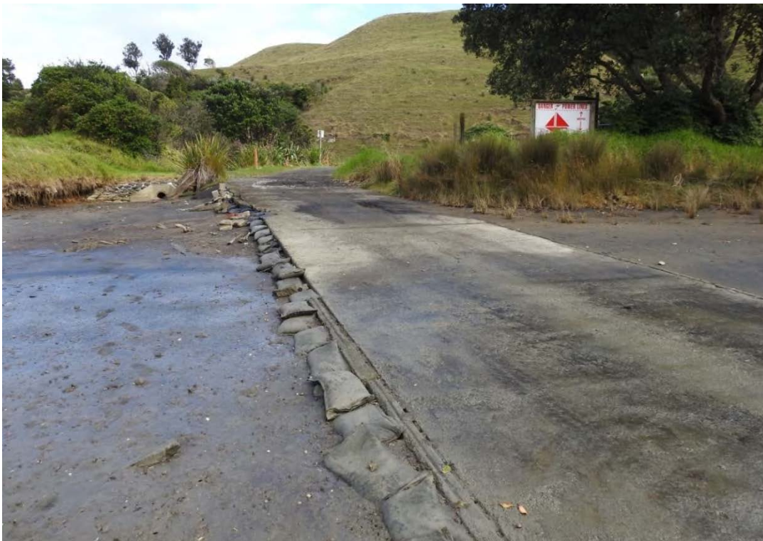
Photo 2 Boat ramp at Tongaporutu (May 2016)
