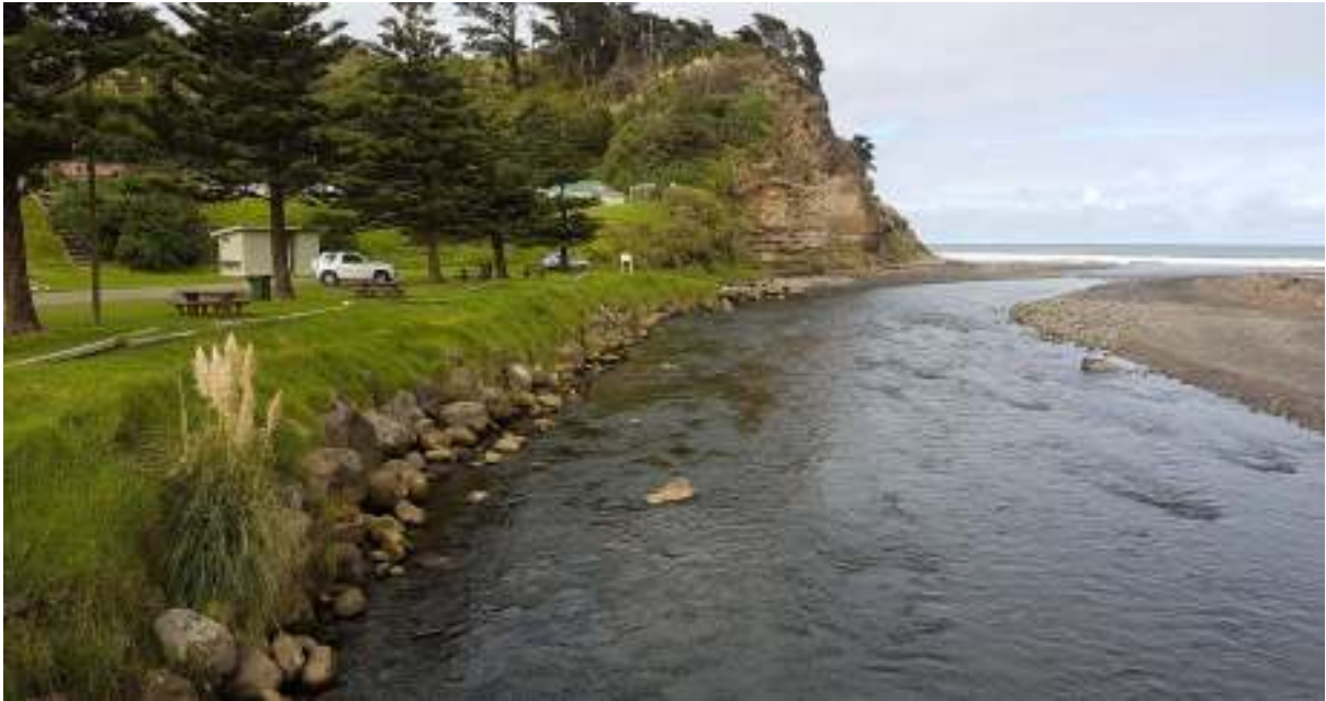
Photo 3 Looking downstream along rock protection works in the Kaipokonui Stream (April 2017)
