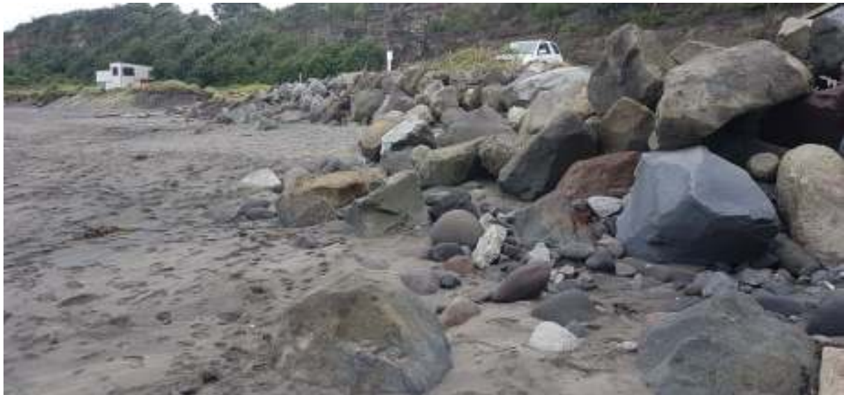
Photo 2 Rip rap seawall, Middleton Bay (April 2017)
