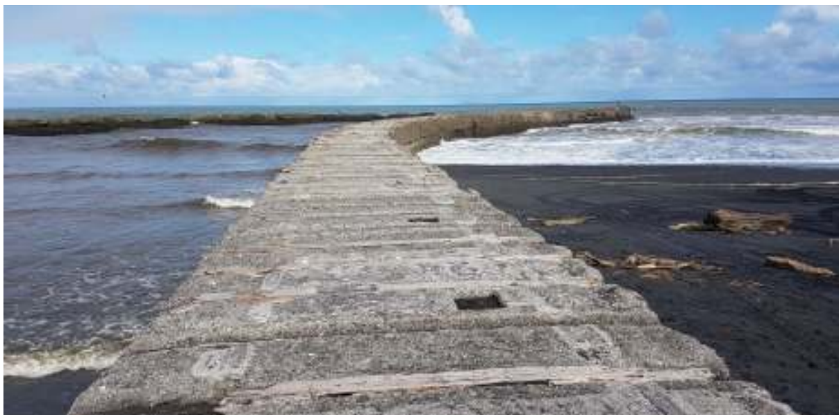
Photo 5 Patea groynes (April 2017)
