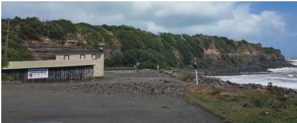
Photo 17 Rocks and gravel washed onto Middleton Bay car park by Ex-Cyclone Fehi.
