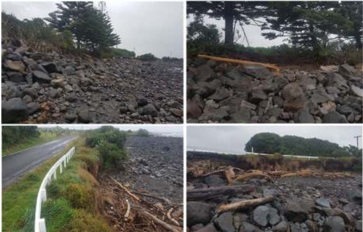
Photo 8 Bayly Road seawall, 11 May 2018
