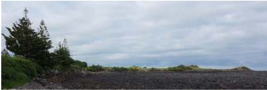
Photo 1 Bayly Road seawall (April 2017)
