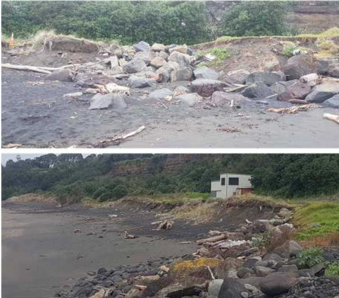
Photo 9 Middleton Bay seawall and dunes, 11 May 2018
