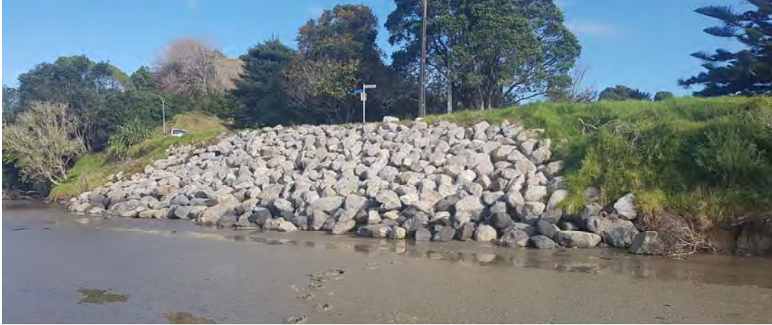
Photo 2 Urenui Estuary rock rip rap, May 2019
