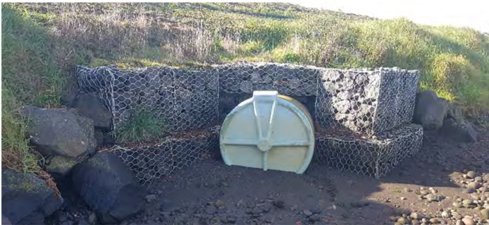
Photo 7 The stormwater outlet by the Atkinson Street/East Quay intersection (May 2018)
