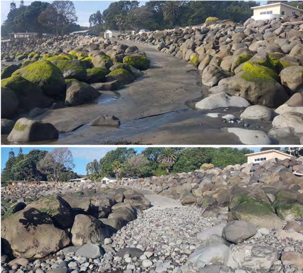
Photo 4 Onaero Beach settlement seawall (top: May 2018, bottom: May 2019)
