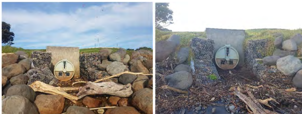
Photo 15 Te Henui stormwater outlet (left: May 2018, right: May 2019)
