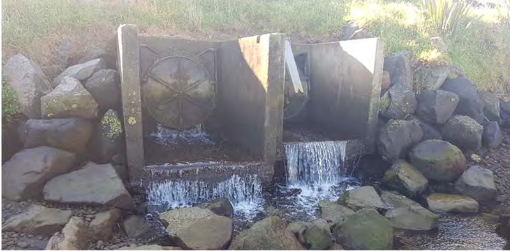
Photo 6 Outlet structure downstream of Atkinson Street (May 2019)
