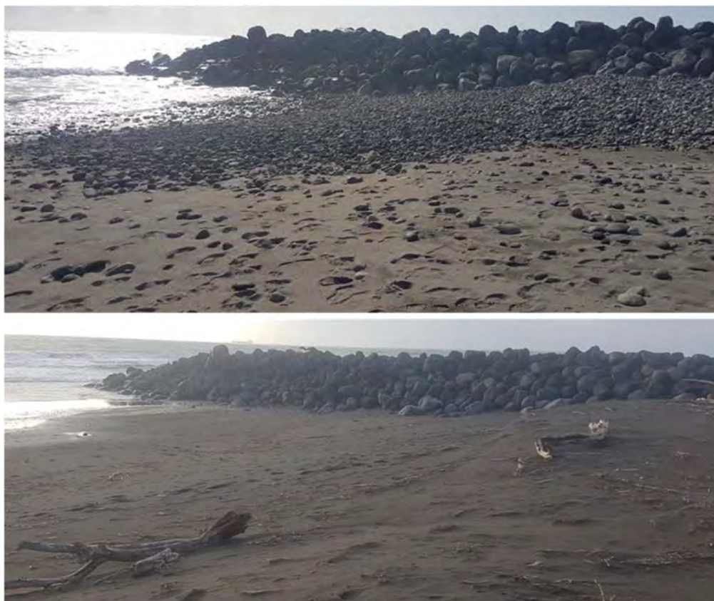
Photo 11 Waiwhakaiho groyne (top: May 2018, bottom: May 2019)
