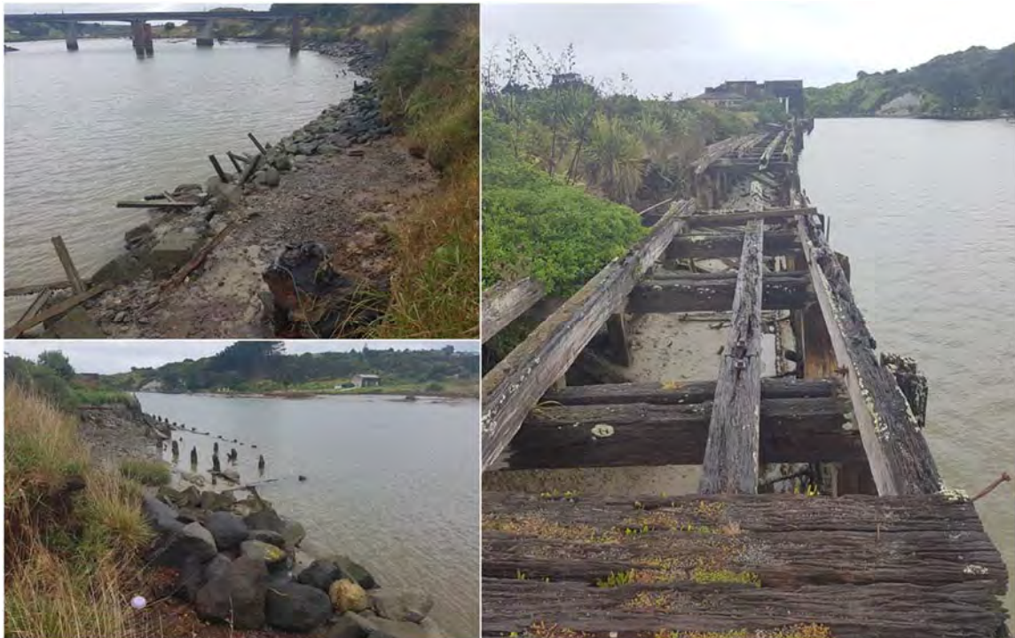
Photo 14 Patea wharf and rock wall, 11 April 2019
