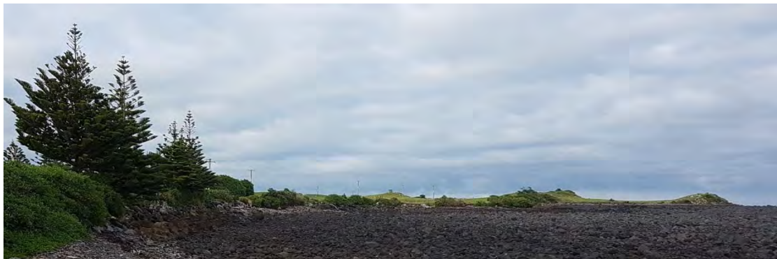
Photo 1 Bayly Road seawall (April 2017)
