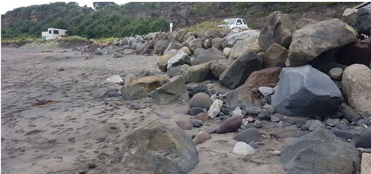
Photo 2 Rip-rap seawall, Middleton Bay (April 2017)
