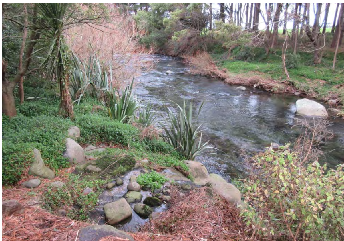
Photo 3 Outfall from the southern stormwater pond to Kaupokonui Stream (STW002078)
