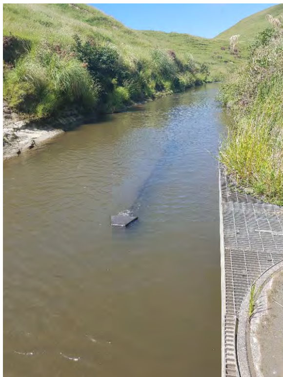
Photo 2 Tangahoe River intake structure
