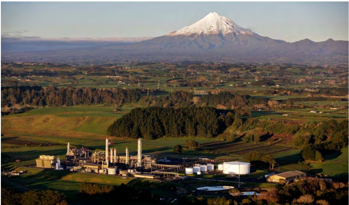
Photo 5 Methanex Waitara Valley site
