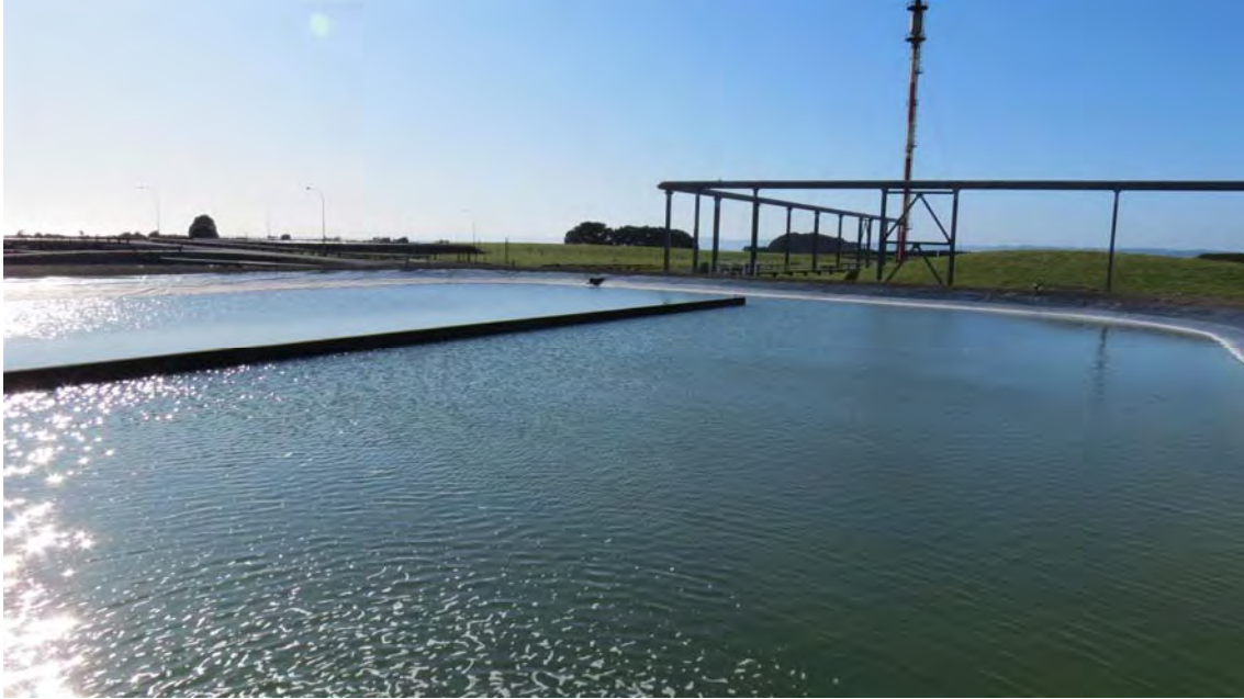
Photo 2 The Motunui site's blow down pond (decommissioned flare 2 can be seen in the background)
