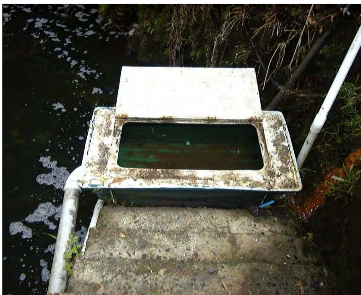
Photo 1 Elver trap at the base of the tail race at the power station, prior to upgrade
