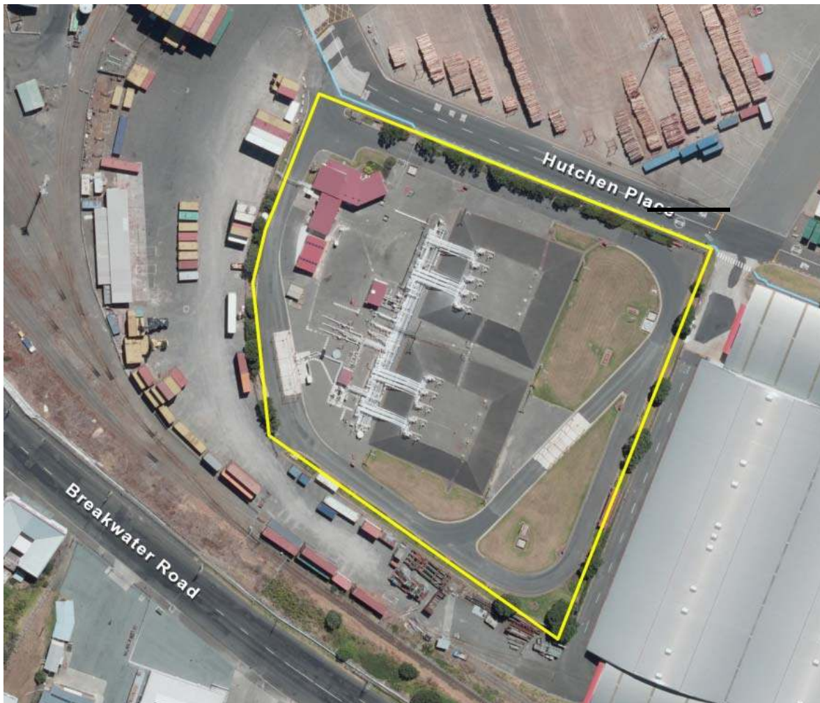
Figure 4 Liquigas site and sampling point
