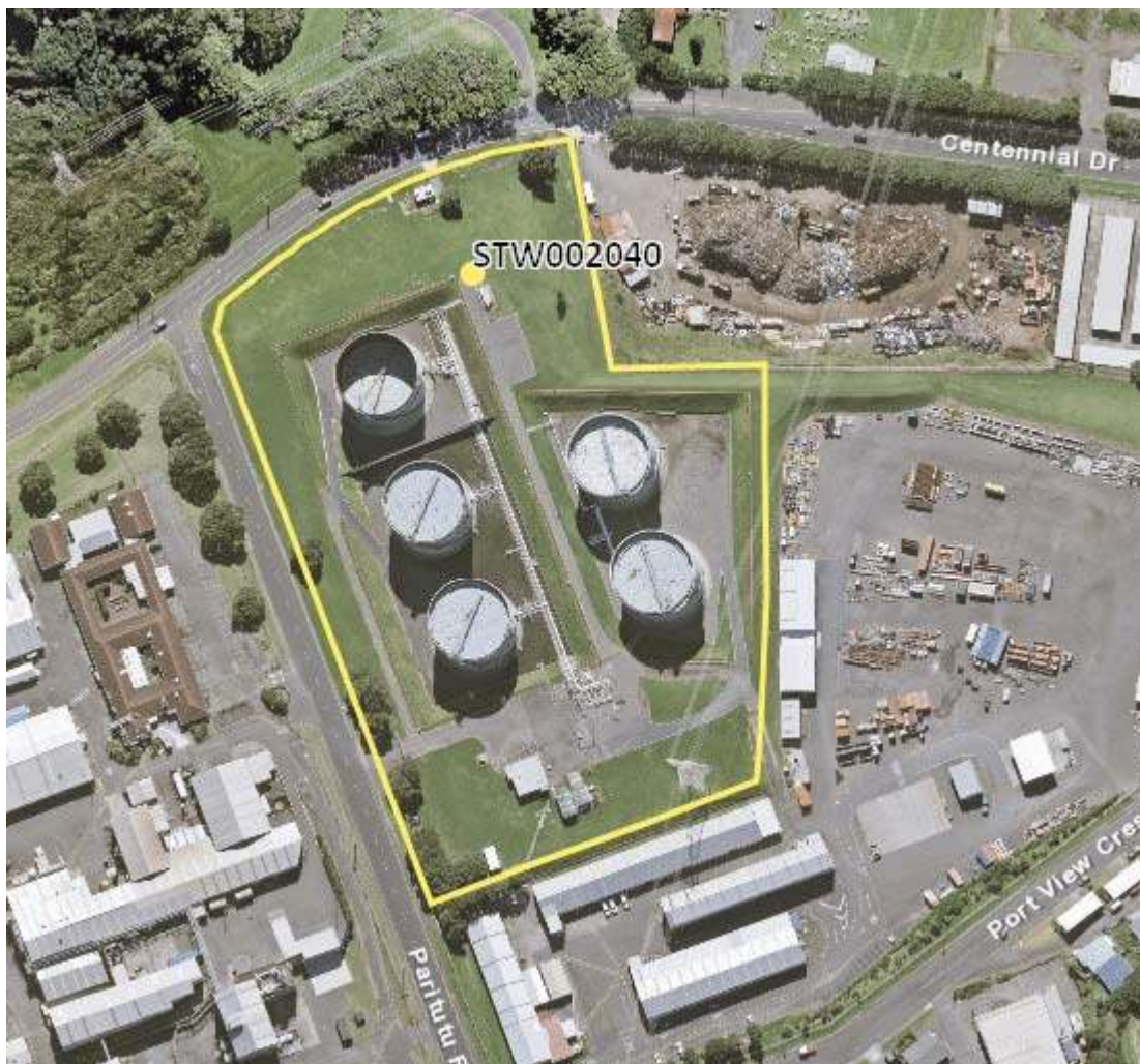
Figure 6 Aerial photograph of the OMV Paritutu Tank Farm
