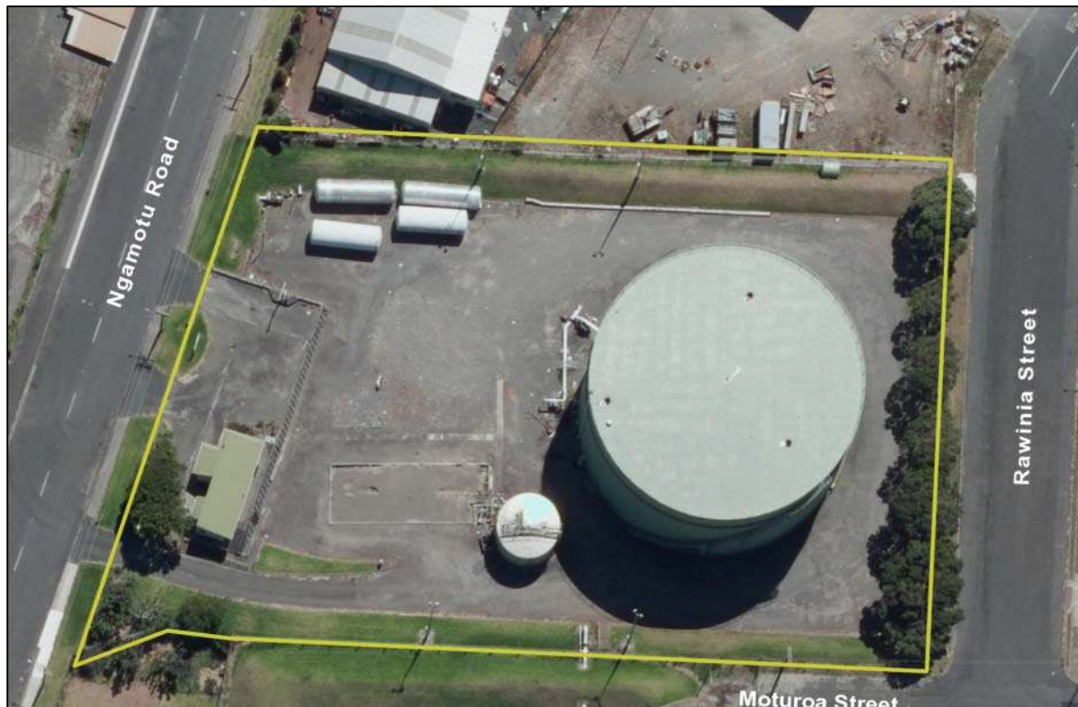
Figure 3 Aerial photograph of the Port Taranaki bulk storage facility
