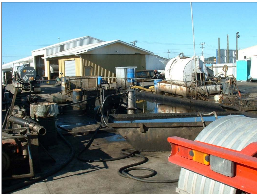
Photo 3 Intergroup Ltd oil treatment facility
