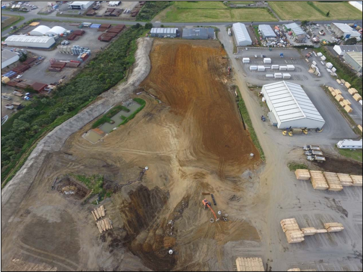
Figure 8 Aerial view of site development at Taranaki Sawmills
