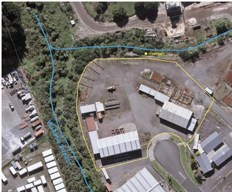
Figure 16 Aerial view of the Pounamu Oilfield Service's site
