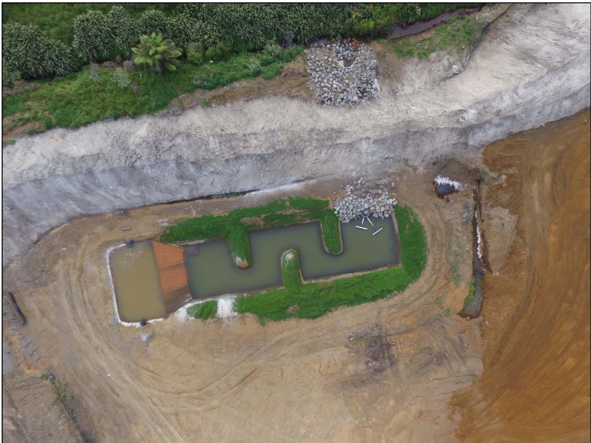
Figure 9 Aerial view of new sediment treatment pond at Taranaki Sawmills
