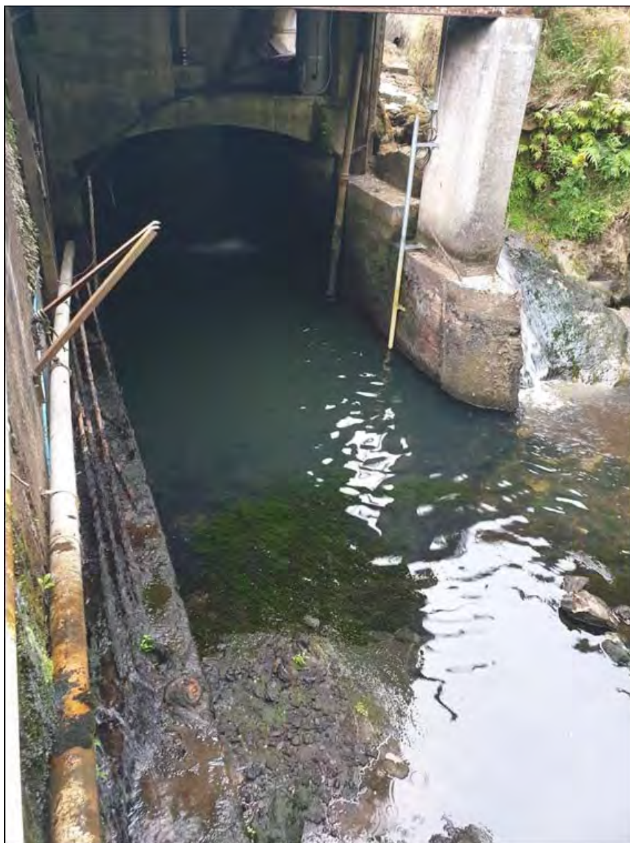
Photo 7 Top photo showing water level during power generation and the bottom two photos show water level when generation ceases. The bottom photo shows that the entrance to the trap appears to be left out of the water, with minimal attractant flow.
