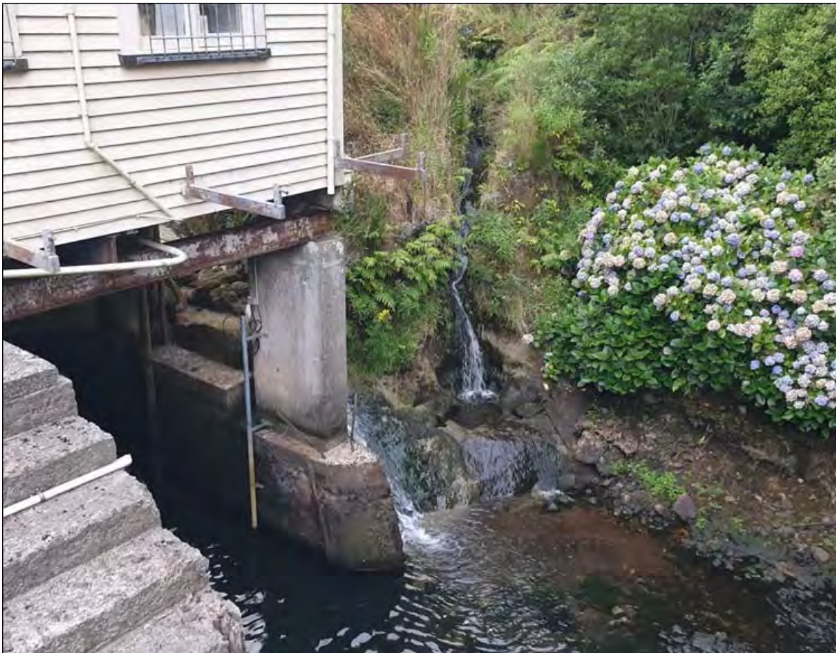
Photo 6 Two attractant flows that direct fish away from the trap. One small tributary (right) and one coming from the station (left beside the concrete pillar). There is a third residual flow from the station outlet pipe directly below the building (seen in Photo 7).
