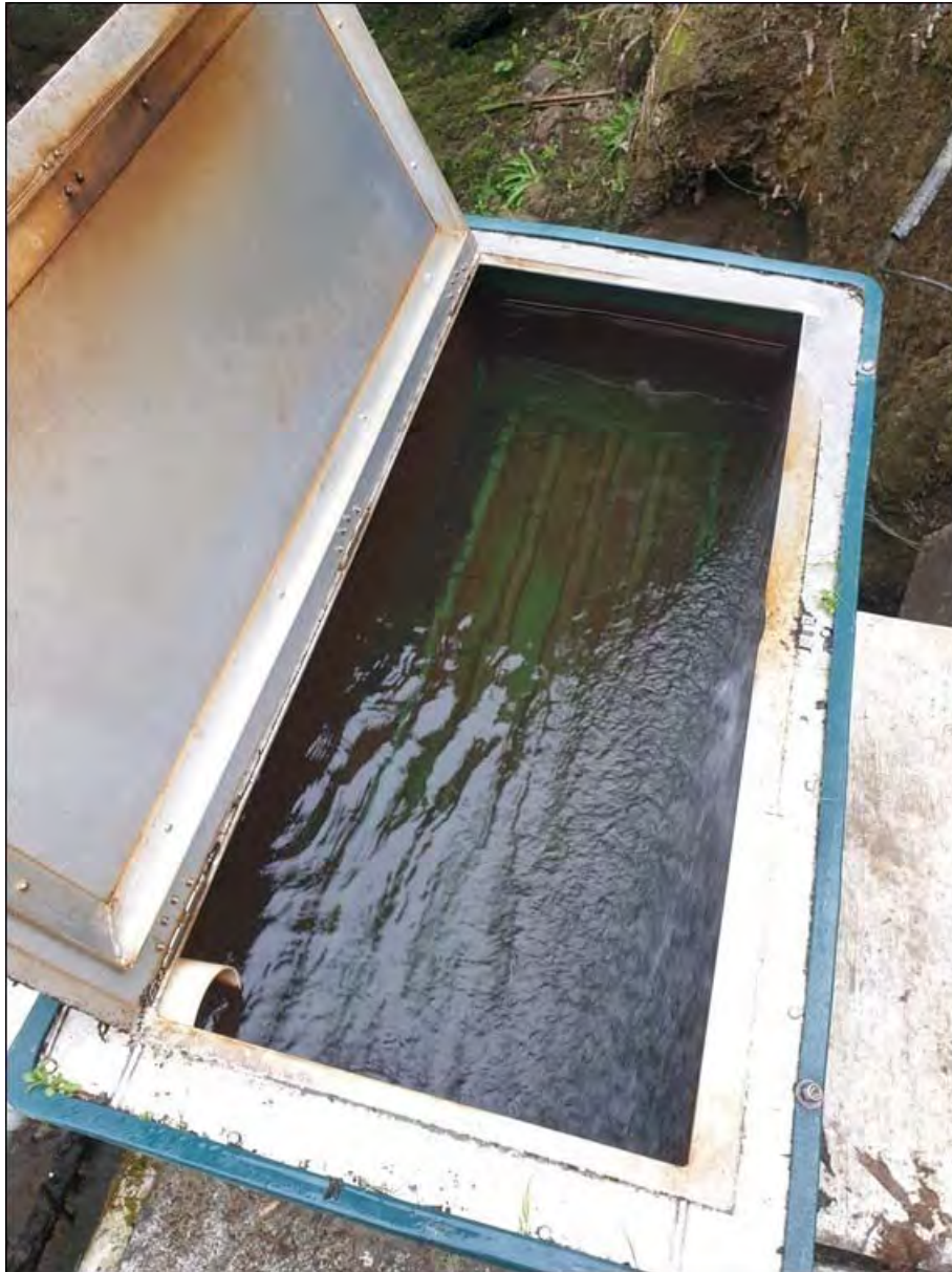
Photo 5 Photo taken of elver in the trap December 2019. Elver enter a pipe carrying the attractant flow, which leads to the trap. These elver are then transferred to an area above the Manganui River head works.
