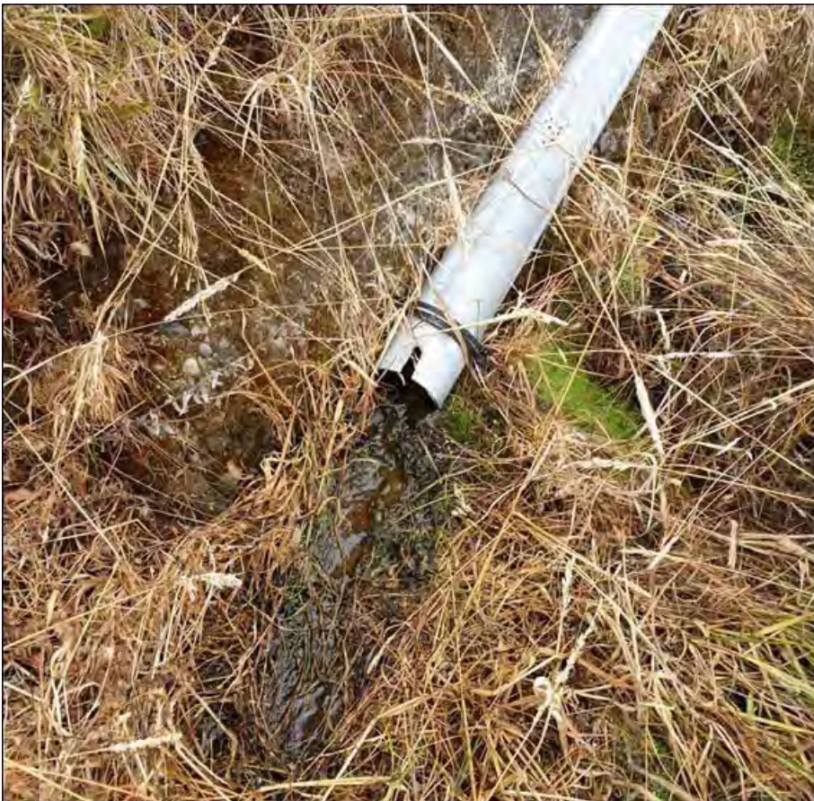
Photo 4 Fish pass at spillway (top). Fish pass inlet (bottom).
