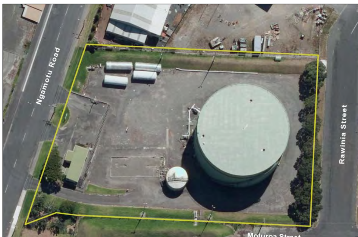
Figure 4 Aerial photograph of the Port Taranaki bulk storage facility
