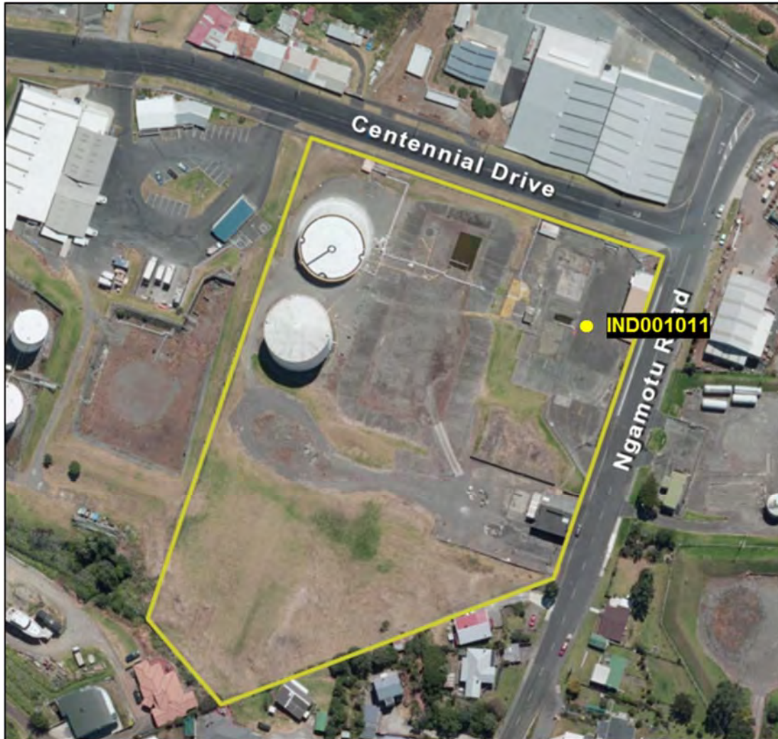
Figure 6 Aerial photograph of the Z Energy Ltd Ngamotu site
