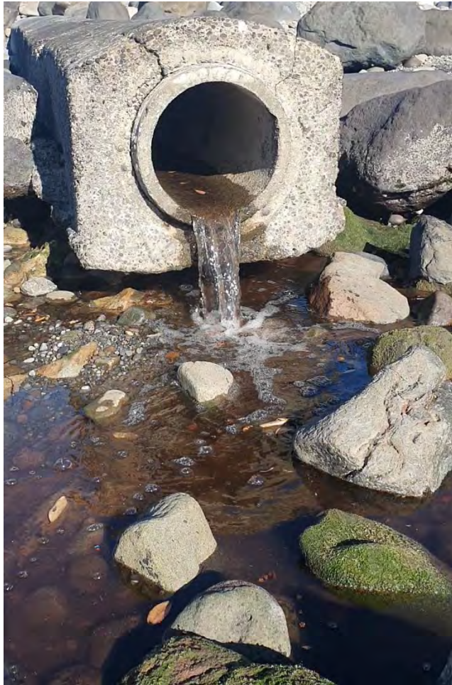
Photo 5 Discharge from outfall (6 May 2020)
