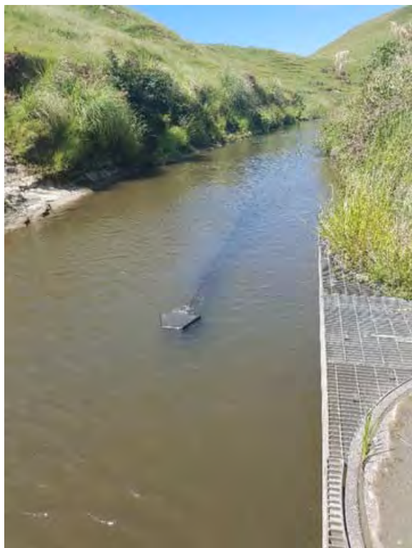
Photo 2 Tangahoe River intake structure
