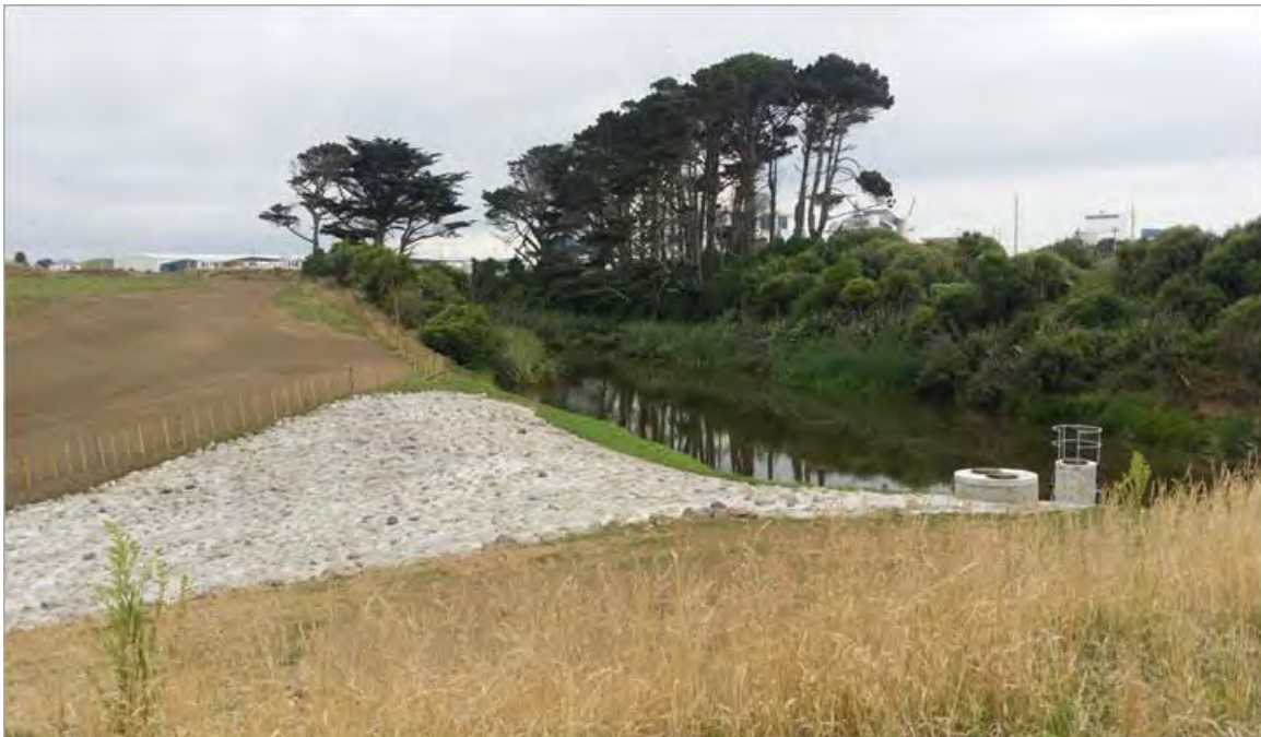
Photo 3 Southern stormwater pond following upgrade (surrounded by native riparian plantings)
