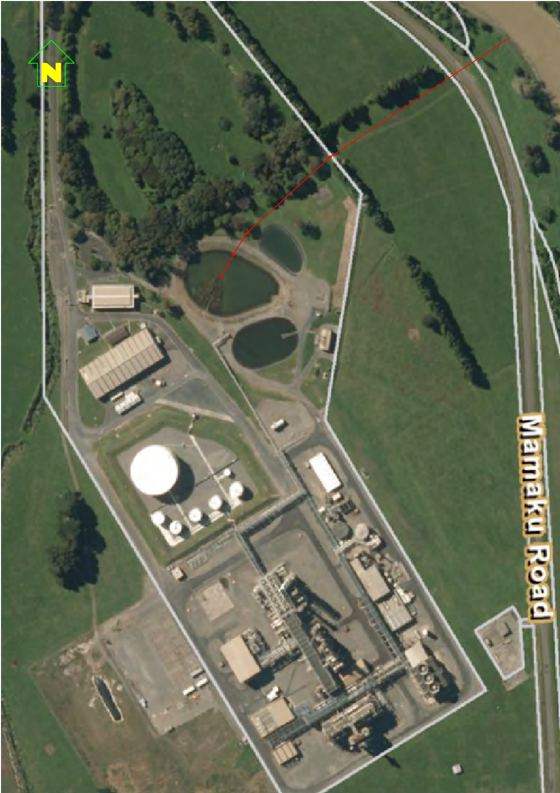
Figure 1: Aerial image of the Waitara Valley Plant showing the pipeline from the stormpond to the Waitara River
