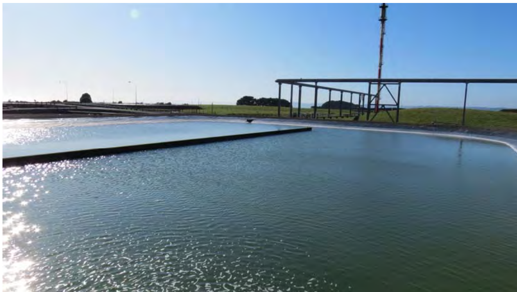
Photo 2 The Motunui site's blow down pond (decommissioned flare 2 can be seen in the background)
