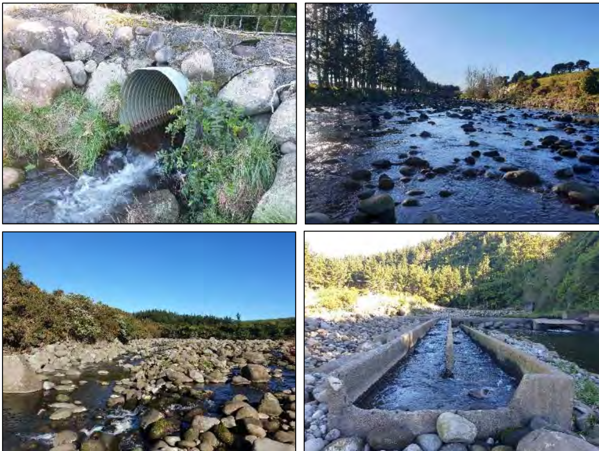
Photo 1 The access culvert licensed by resource consent 6810-1 (top left), the Waiwhakaiho River at Hydro Rd (top right), the Waiwhakaiho River upstream of Mangamahoe Stream outlet (bottom left), and the intake weir (bottom right)
