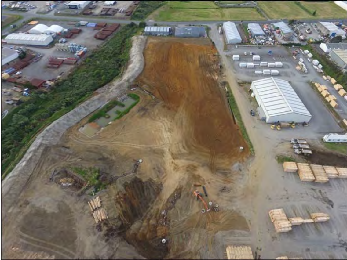
Figure 11 Aerial view of site development at Taranaki Sawmills, c. 2018
