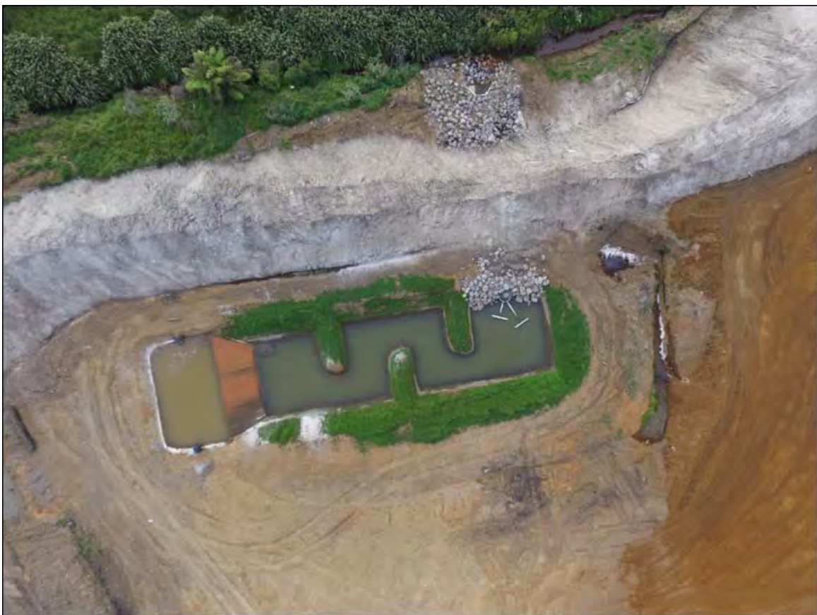
Figure 12 Aerial view of new sediment treatment pond at Taranaki Sawmills
