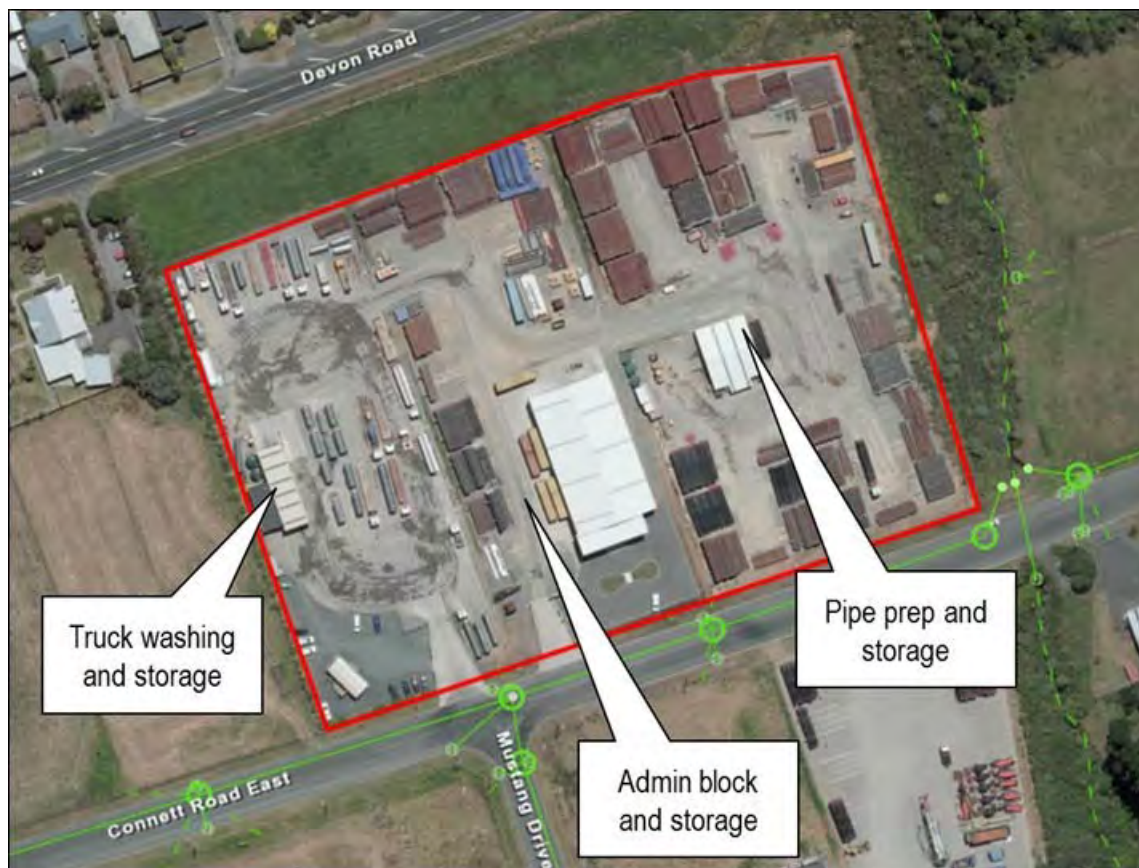
Figure 8 Aerial view of Symons' site with various work areas
