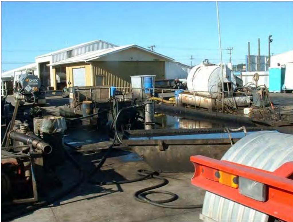
Photo 3 Intergroup Ltd oil treatment facility
