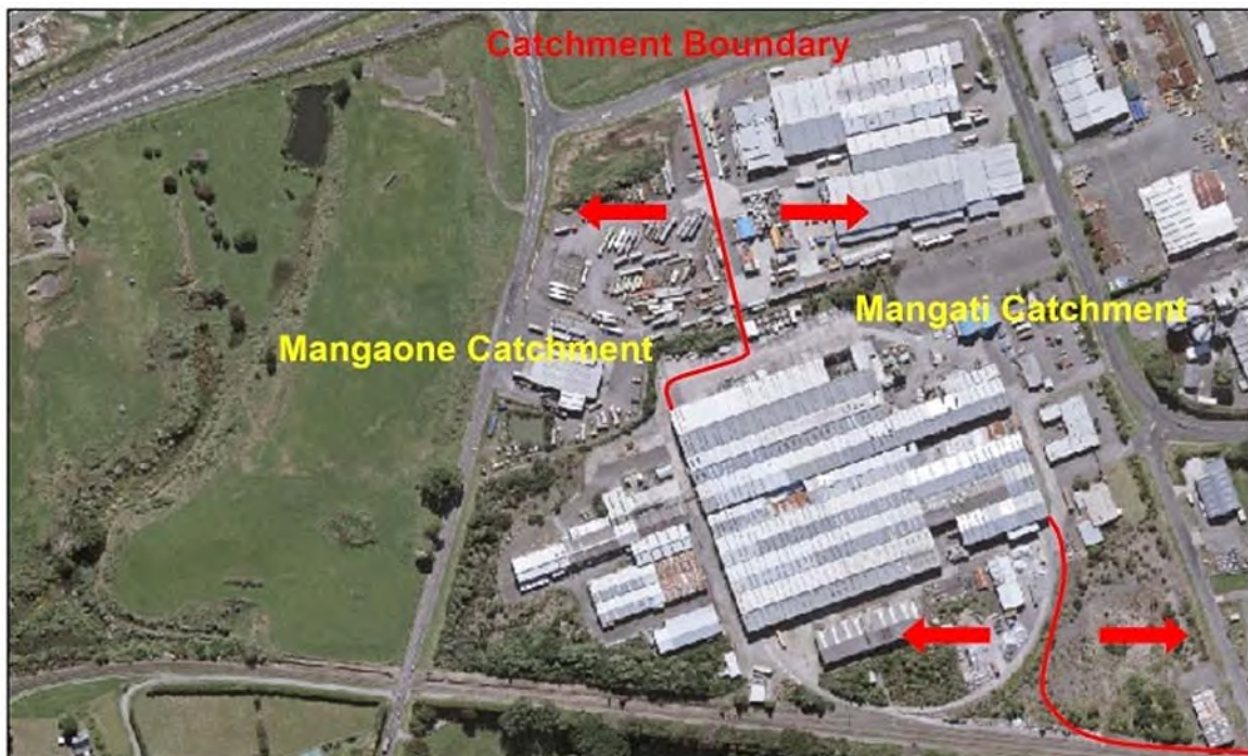
Figure 1 MASL foundry site, showing the boundary between Mangaone and Mangati Stream catchments
