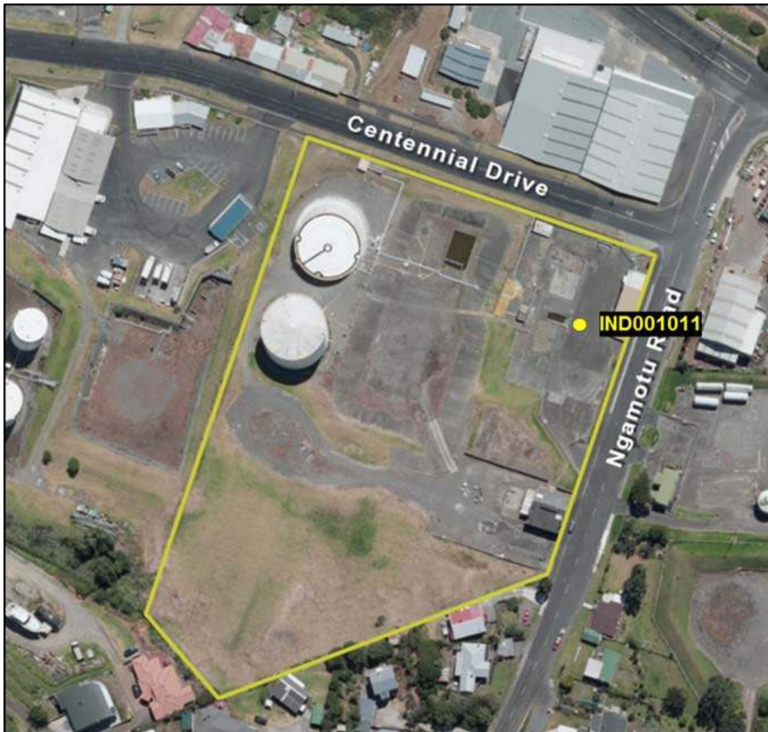
Figure 11 Aerial photograph of the Z Energy Ltd Ngamotu site
