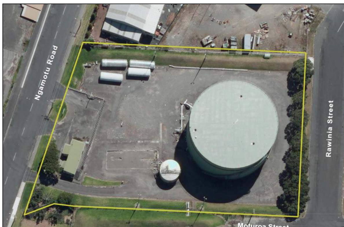
Figure 9 Aerial photograph of the Port Taranaki fire water storage facility
