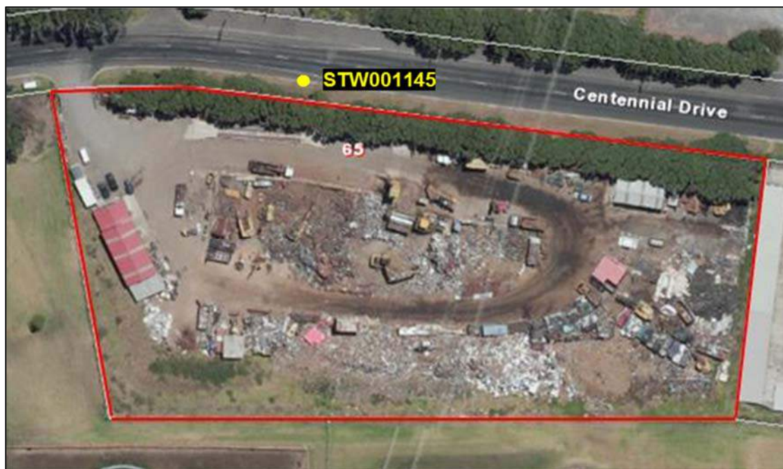
Figure 13 Aerial photograph of the Molten Metals site
