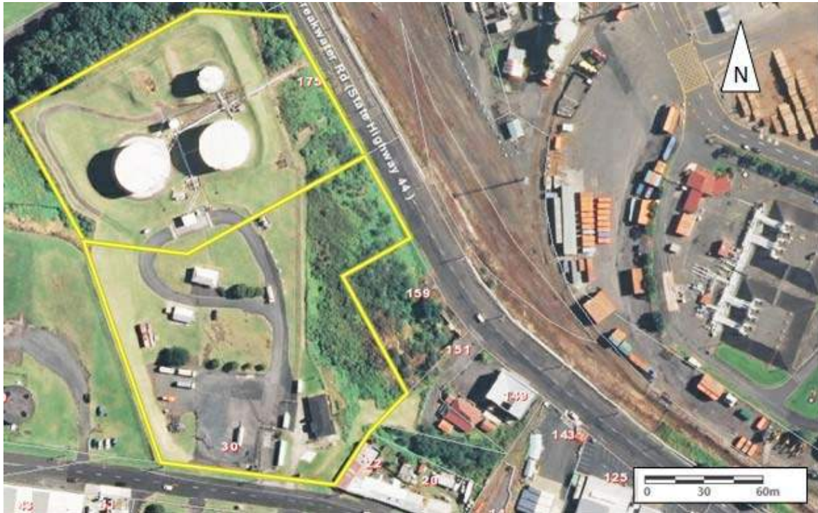
Figure 7 Aerial photograph of the NZOSL Centennial Drive site
