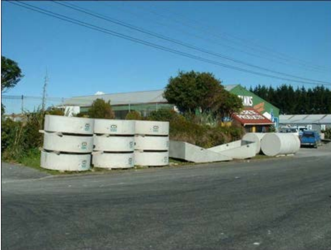
Photo 2 C & O Concrete site
