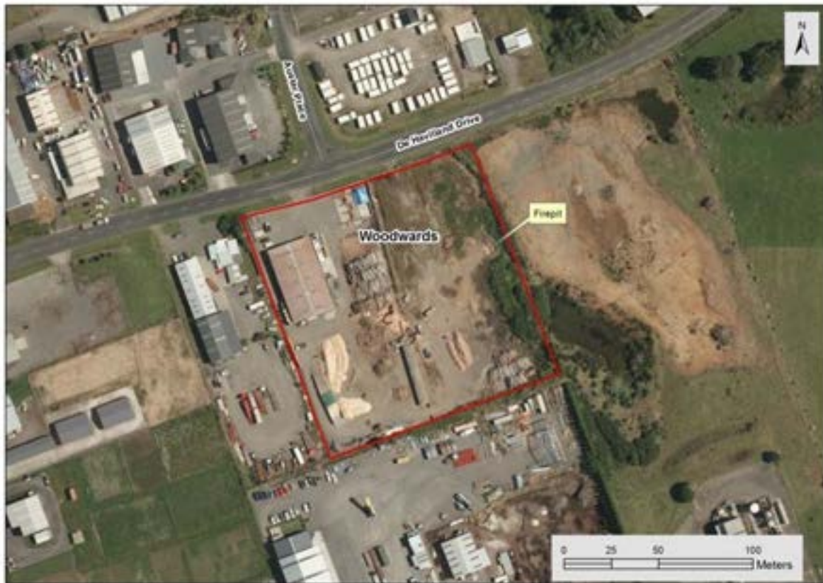
Figure 19 Aerial view of Woodward's site and fire pit location
