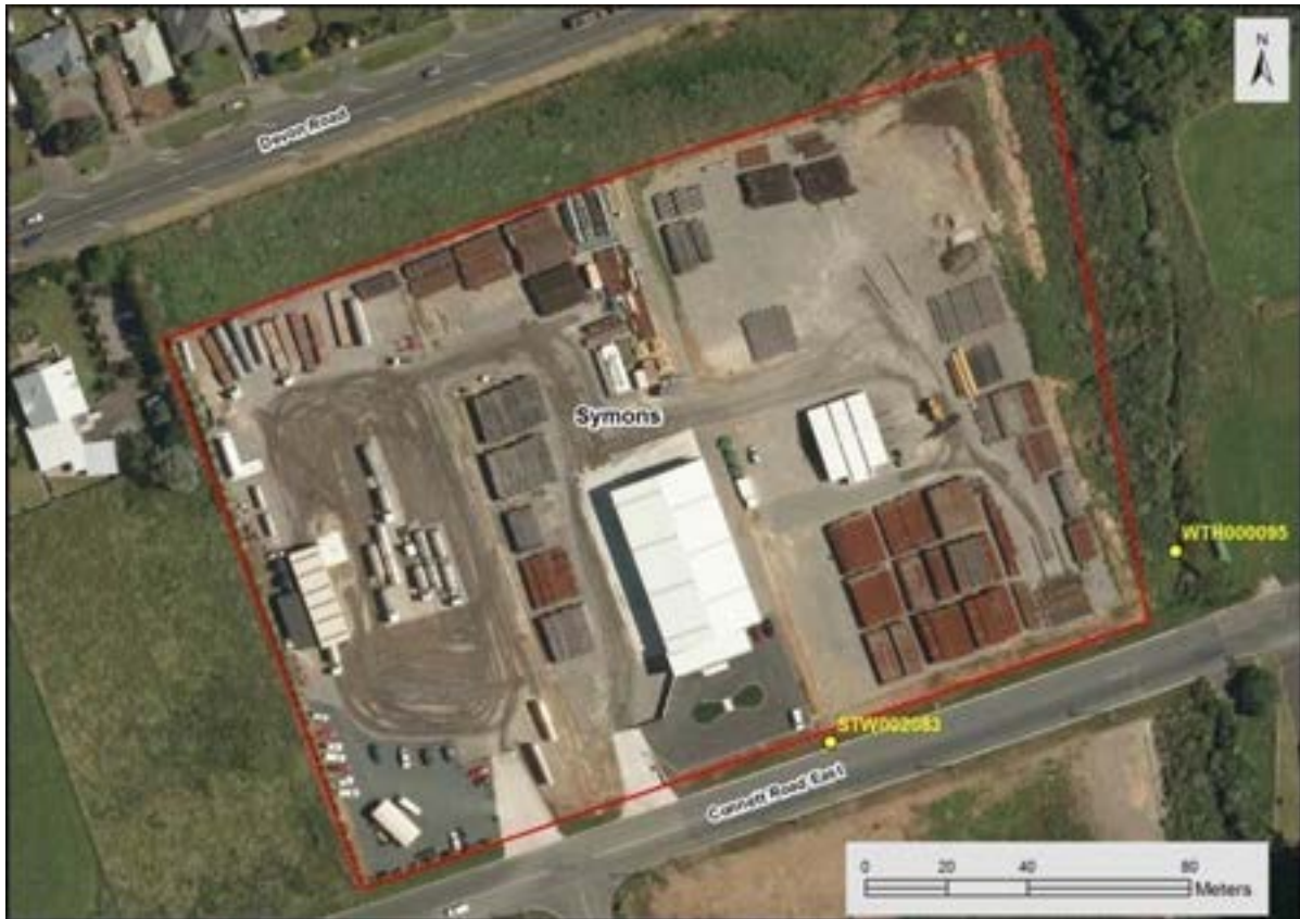
Figure 10 Symons' stormwater discharge sampling point and downstream site
