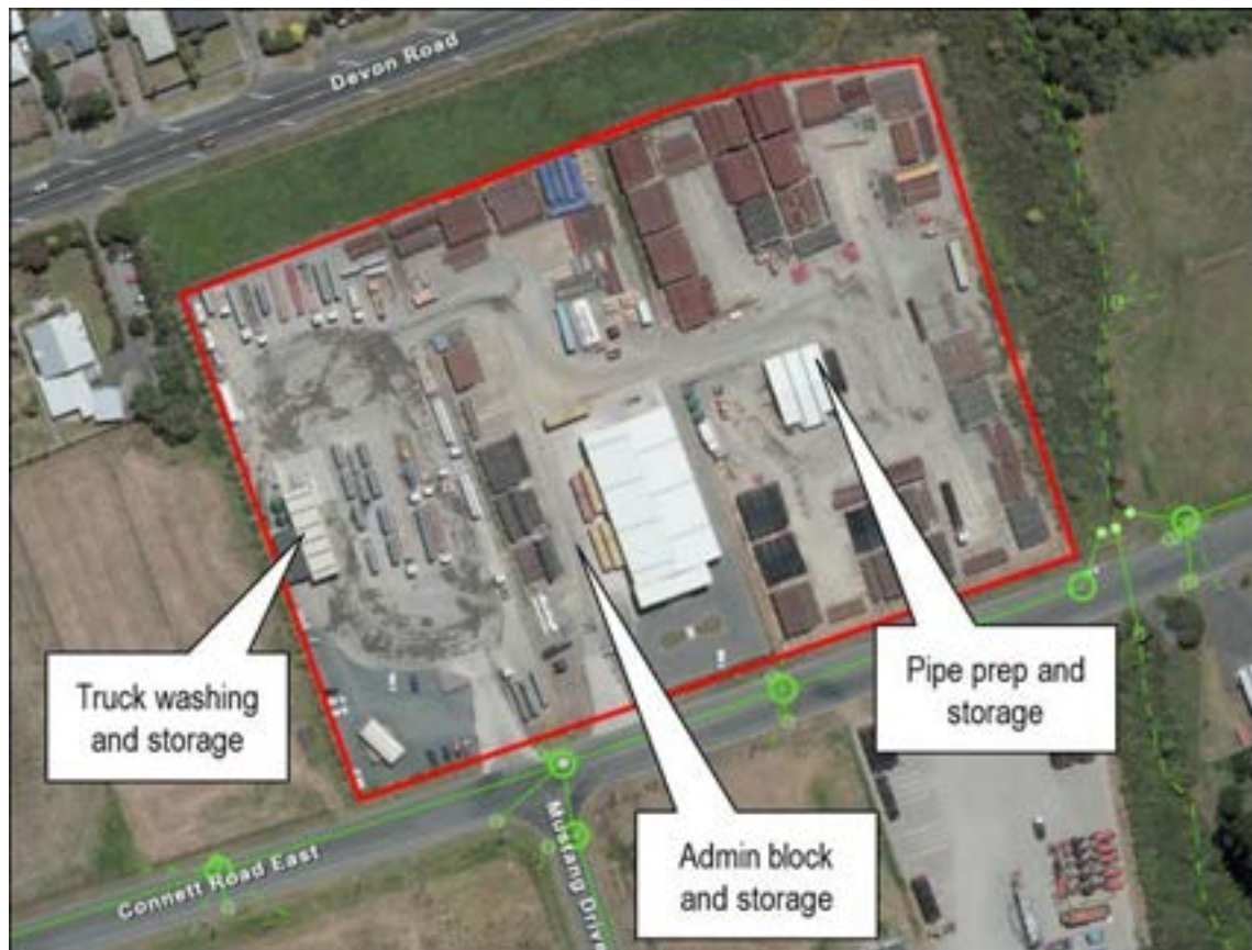
Figure 9 Aerial view of Symons site and various work areas
