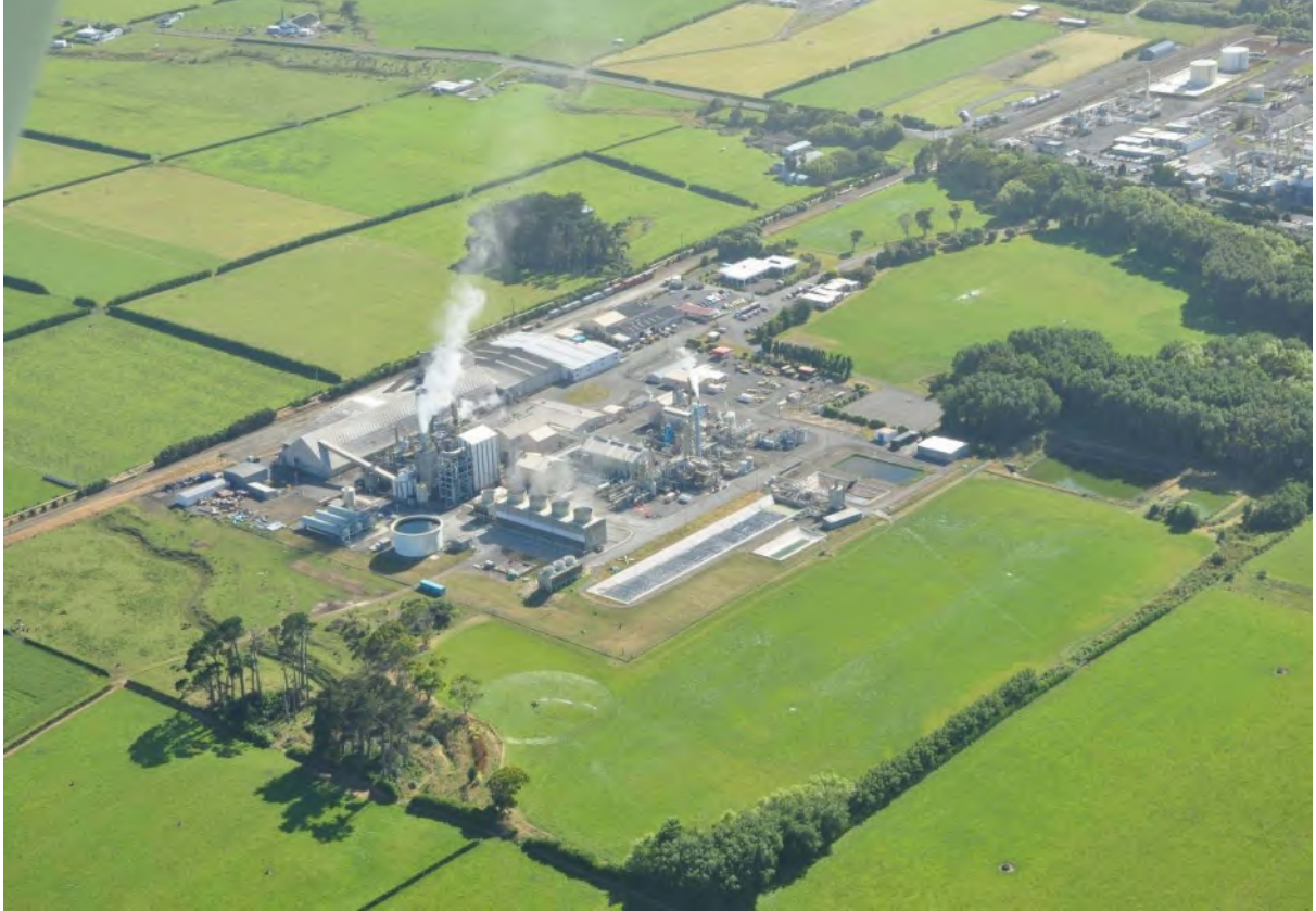
Photo 1 Ballance Agri-Nutrients ammonia urea plant (viewed looking towards the north-west)
