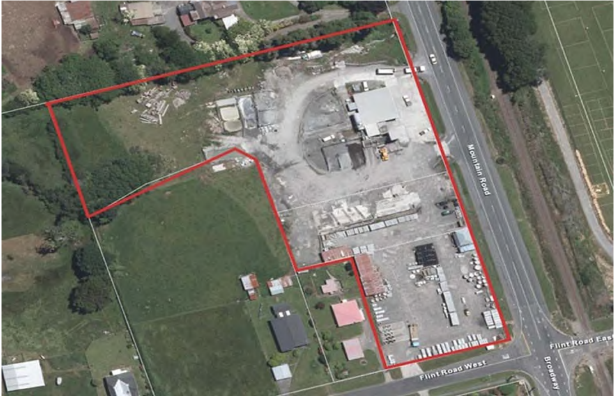
Figure 3 Location of the Fletcher Concrete site (Firth Industries and Humes Pipeline Systems), Stratford
