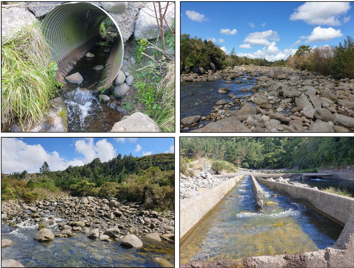
Photo 1 The access culvert licensed by resource consent 6810-1 (top left), the Waiwhakaiho River at Kaipi Rd (top right), the Waiwhakaiho River upstream of Mangamahoe Stream outlet (bottom left), and the intake weir (bottom right)
