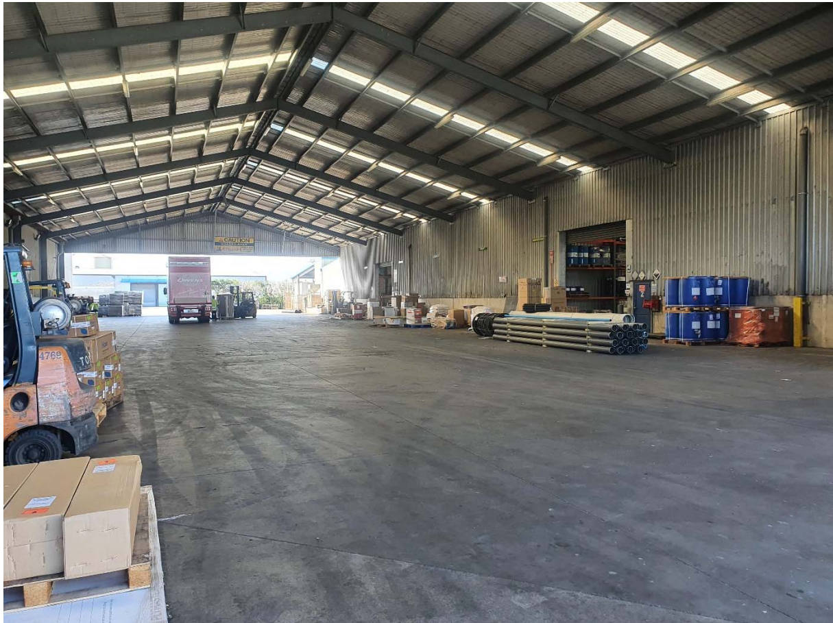
Photo 21 View inside TIL freight loading tunnel, May 2021
