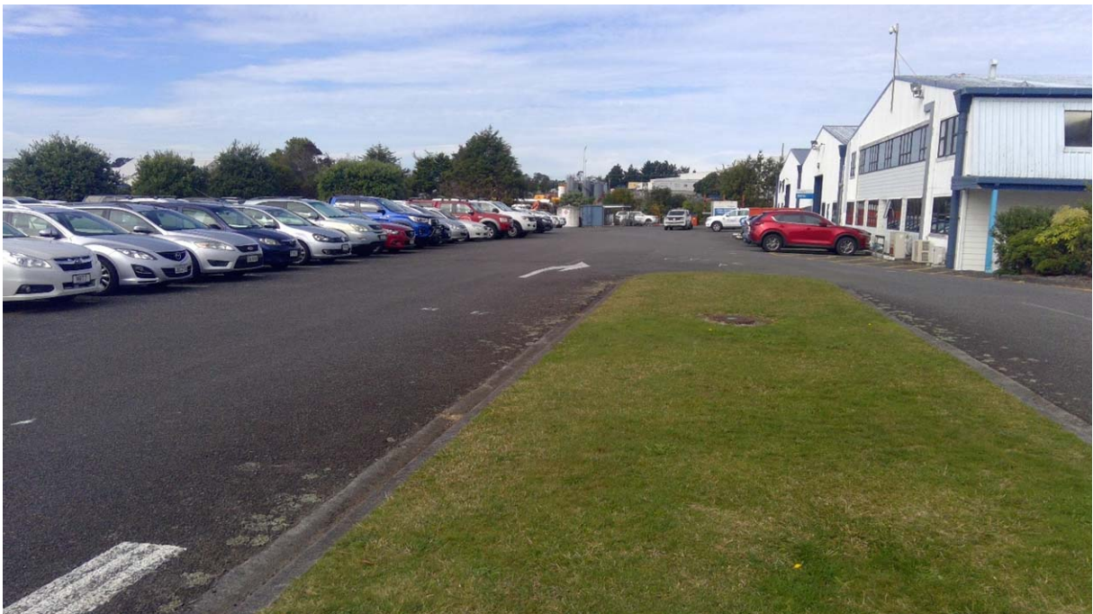
Photo 5 View of stormwater catchment at First Gas site
