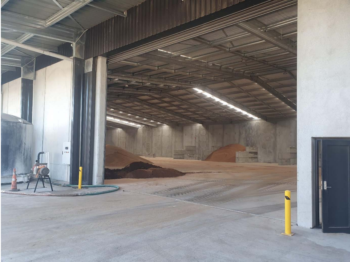
Photo 3 New storage shed at Barton site, June 2021
