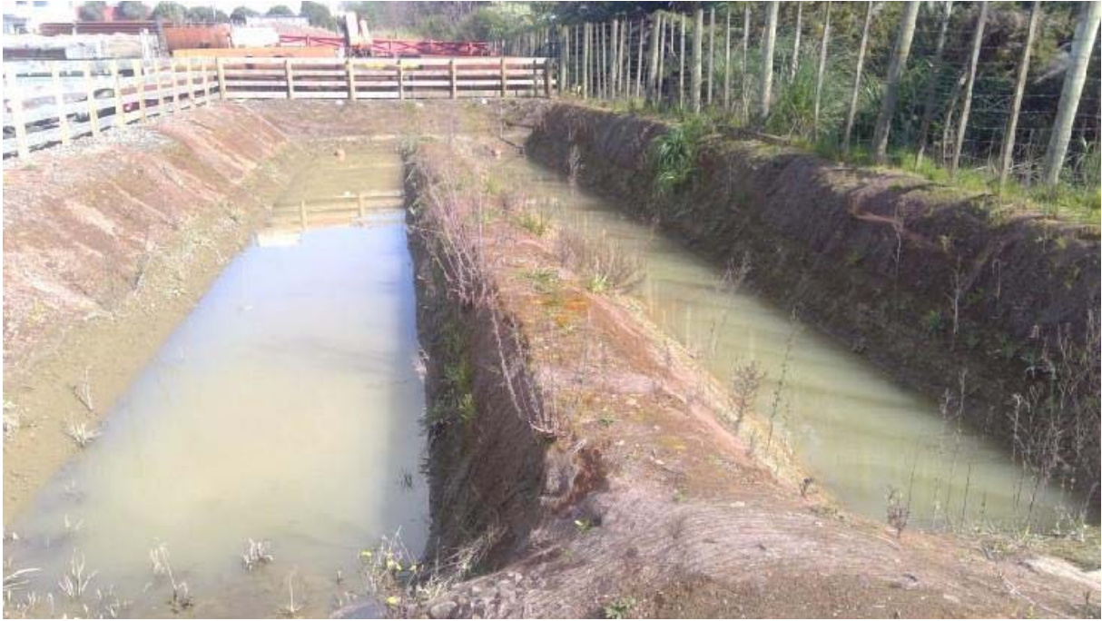
Photo 8 New sediment retention pond, September 2020
