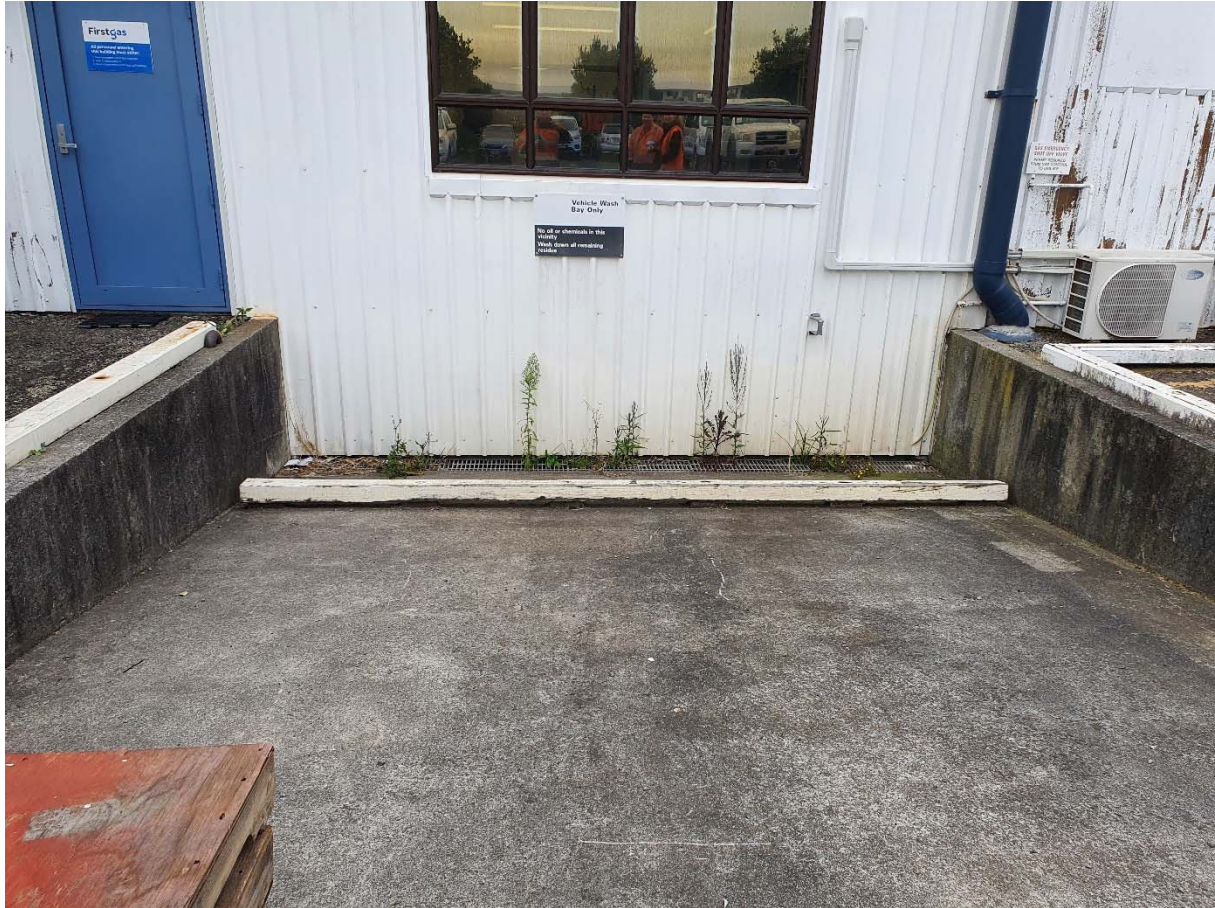
Photo 6 Decommissioned wash bay, August 2020
