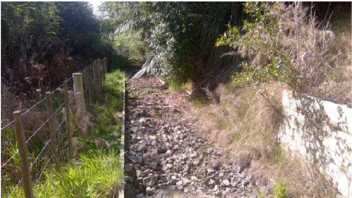
Photo 9 Gravel filter bed installed on GPL pond discharge outlet, September 2020
