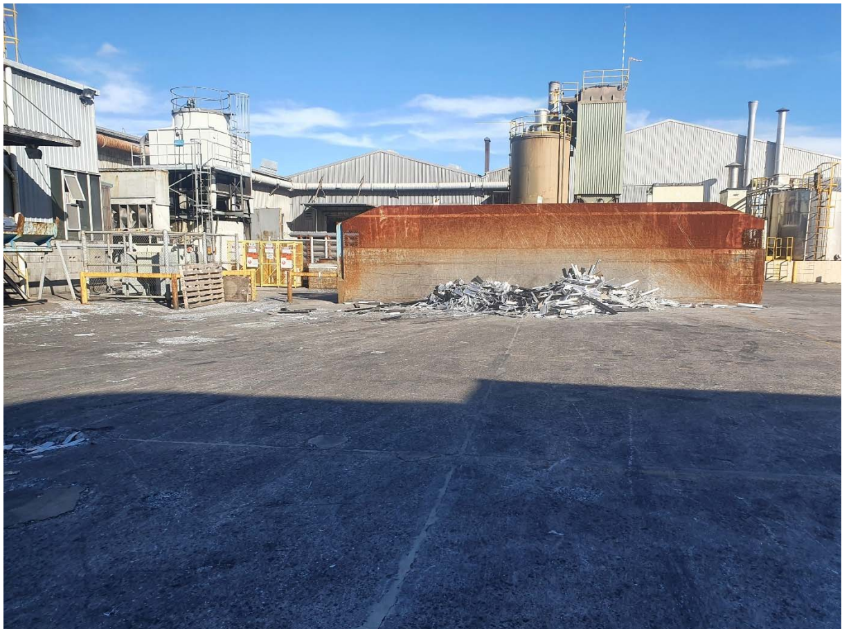
Photo 12 Scrap sorting yard at MCK site, May 2020
