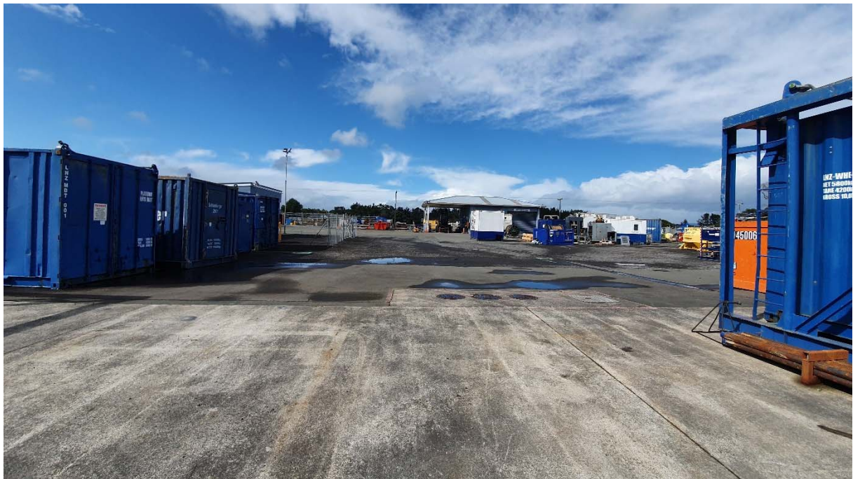
Photo 17 Schlumberger yard and lay dawn area, October 2019
