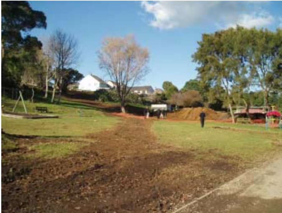
Photograph 5: Looking up stormwater trench through playground to “drum excavation”
