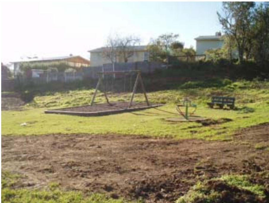
Photograph 6: Playground equipment. Stormwater trench in foreground
