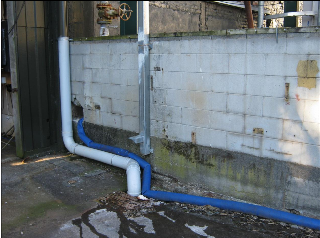
Photograph 1 Oil cooling water sampling point at end of blue hose
