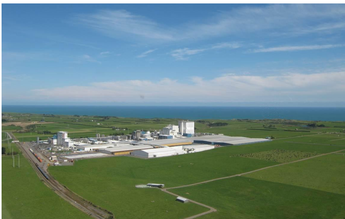
Photograph 1 The Fonterra Whareroa site
