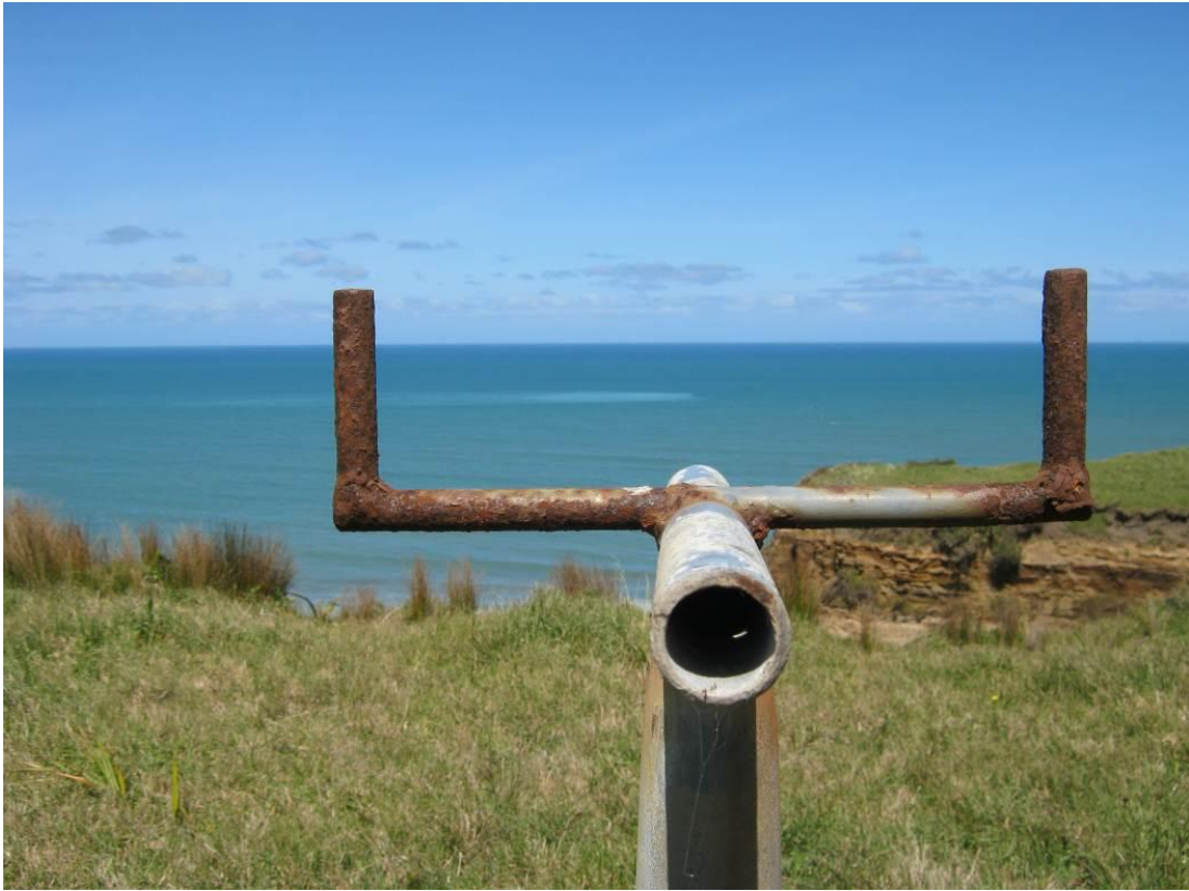
Photograph 10 Outfall discharge visible beyond the 200 m mixing zone on 24 October 2012
