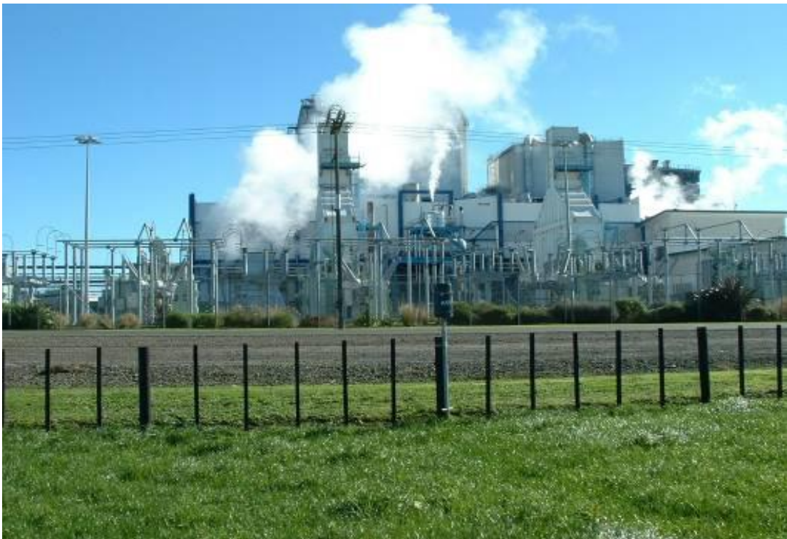
Photograph 3 Air discharges from 'Cogen-I' and 'Cogen-II'
