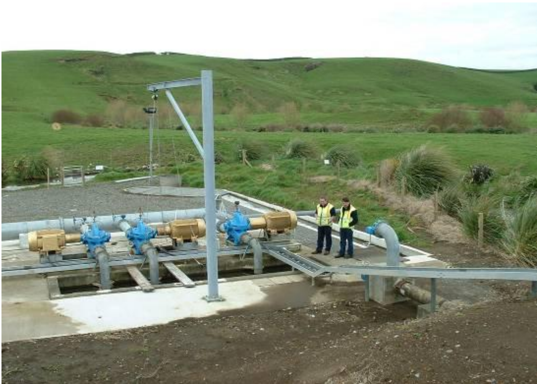
Photograph 2 Tawhiti water intake
