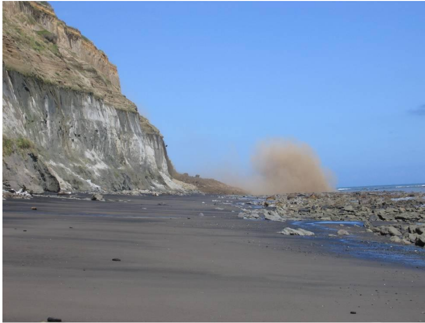
Photograph 8 Erosion of the cliffs close to Pukeroa Reef (2006)
