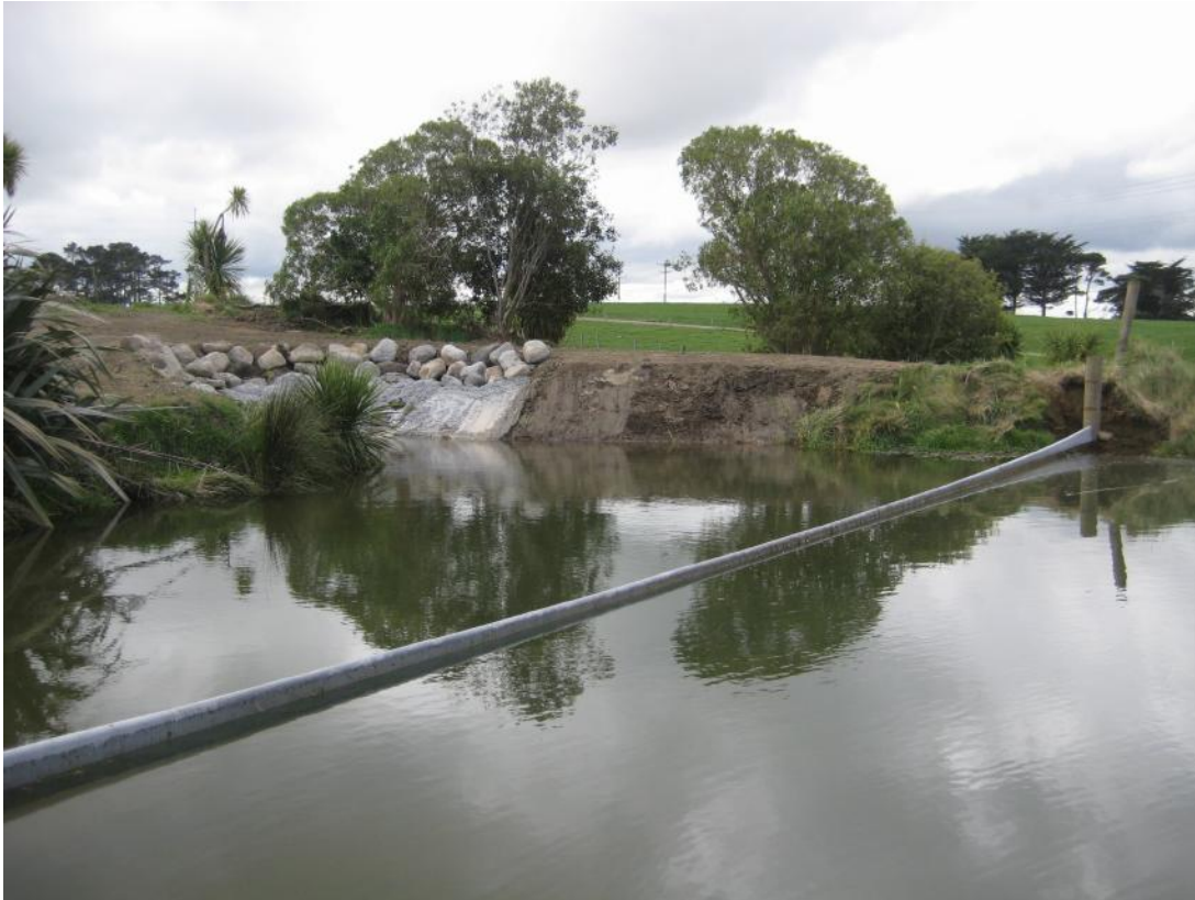
Photograph 6 Tawhiti stormwater pond following remedial work
