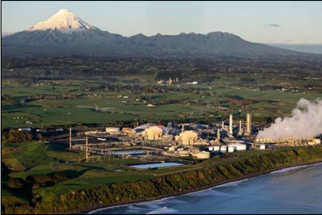
Photo 1 Methanex Motunui site
