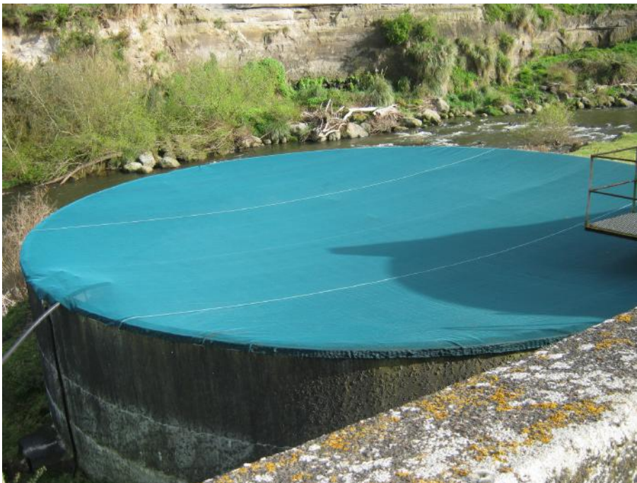
Photograph 1 New cover on the effluent holding tank
