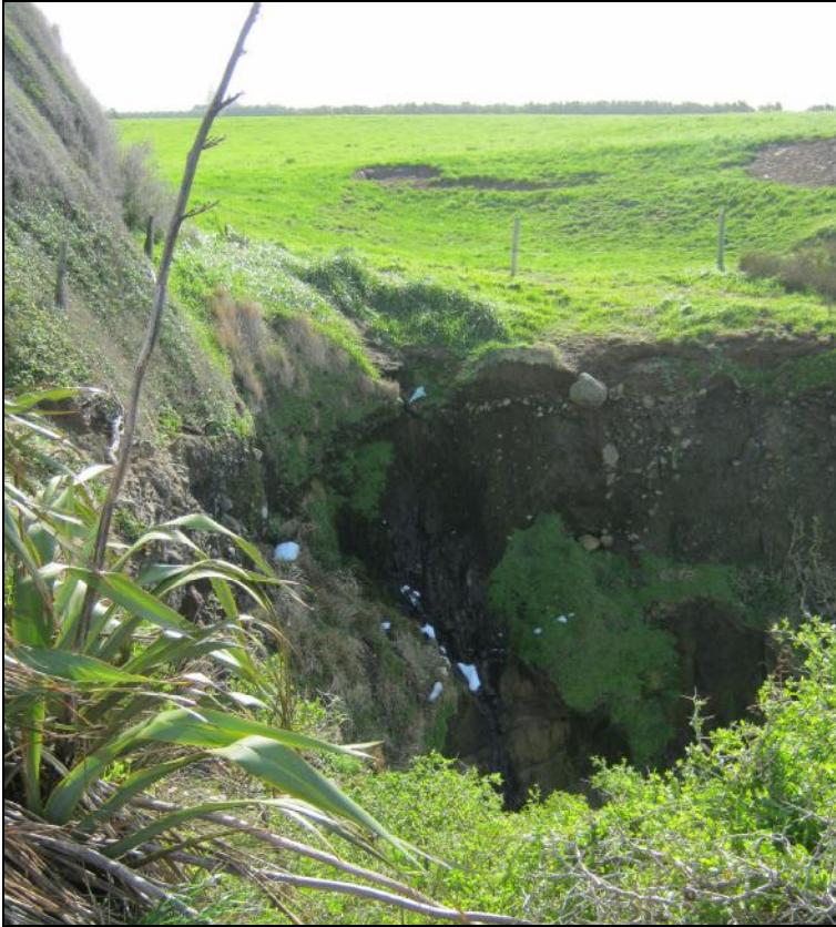
Photograph 2 Foam around point of discharge
